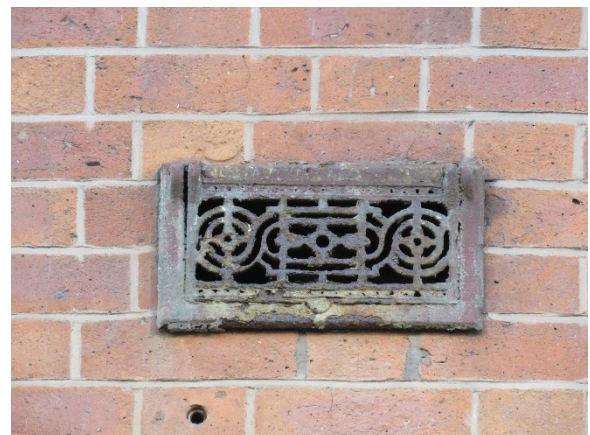
6. Example of an original metal ventilation grill.
