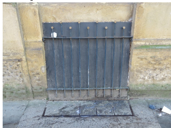
18. Example of in-filled original pavement light.
