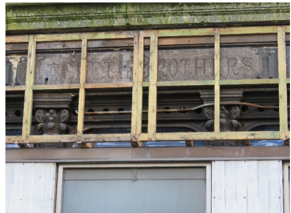
4. Partially uncovered shop frontage with cast iron columns.
