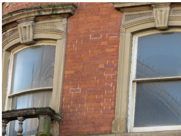
13. Example of patch repointing in cement.
