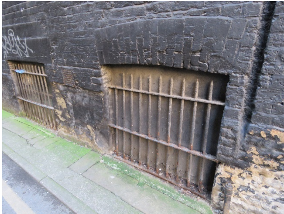
27. Example of early railings to lower ground floor window.
