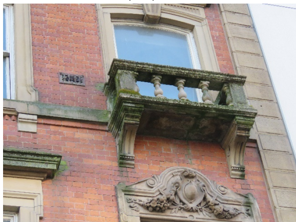
5. Example of sandstone balcony.
