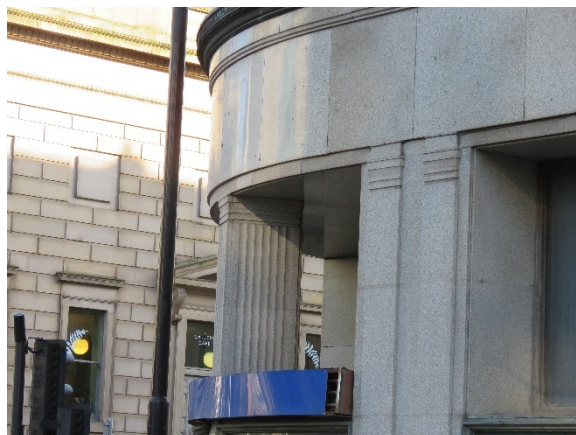
8. Granite cladding to the corner of Mosley Street and Princess Street.
