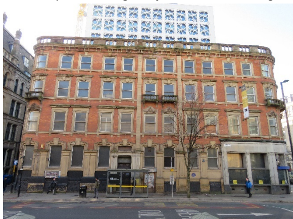
11. Princess Street Elevation (North East)
