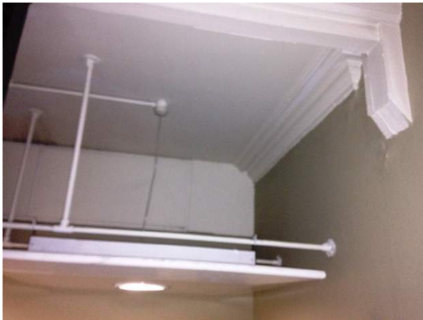
Figure 3.5: Remnant of coving on first floor stair landing
