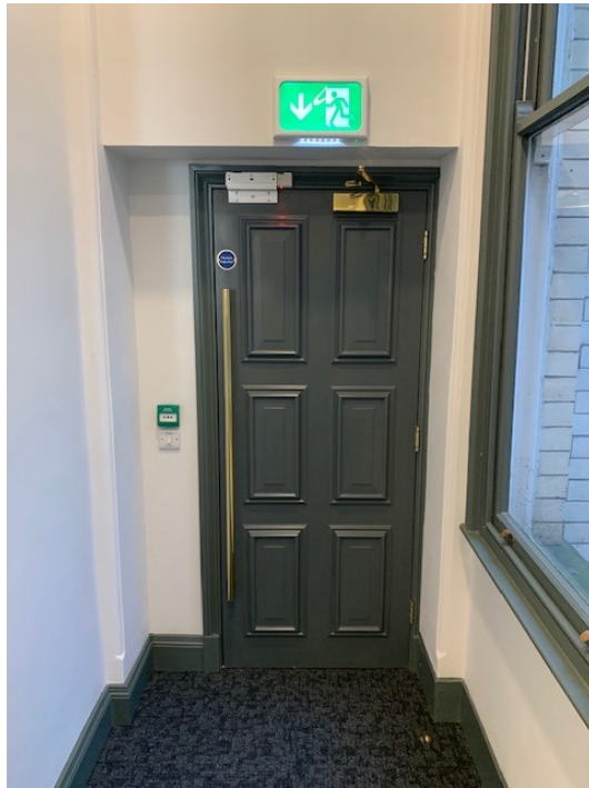
Figure 3.11: Secondary suite door, First Floor
