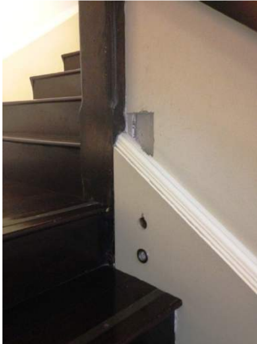
Figure 3.2: Staircase between ground floor and first floor
