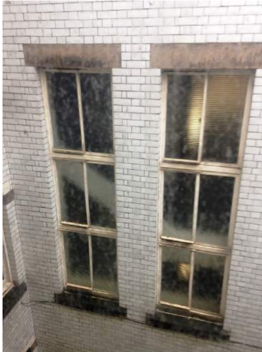
Figure 3.8: Stair windows (photograph taken across light well)
