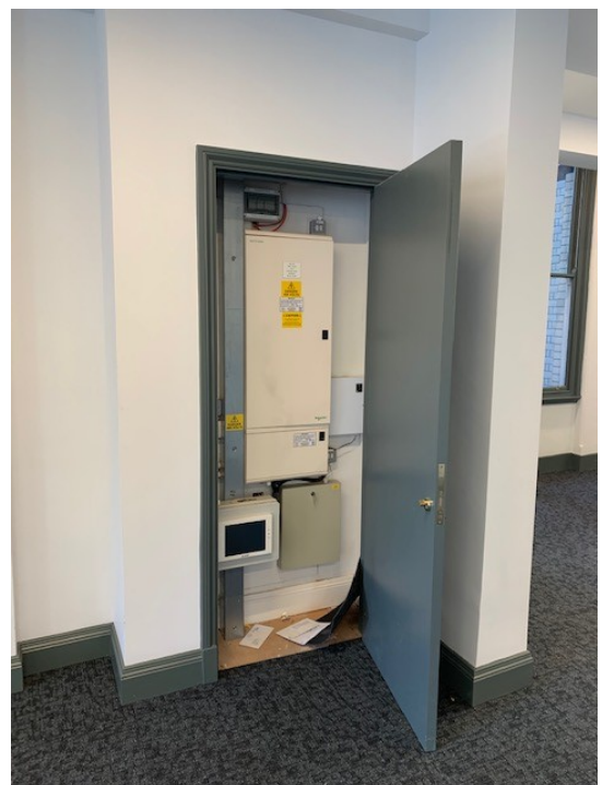
Figure 3.14: Office space, First Floor
