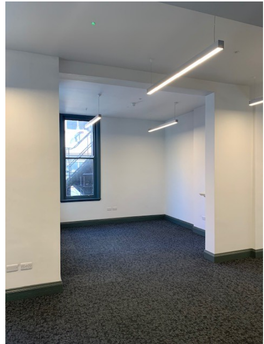
Figure 3.12: Office space, First Floor
