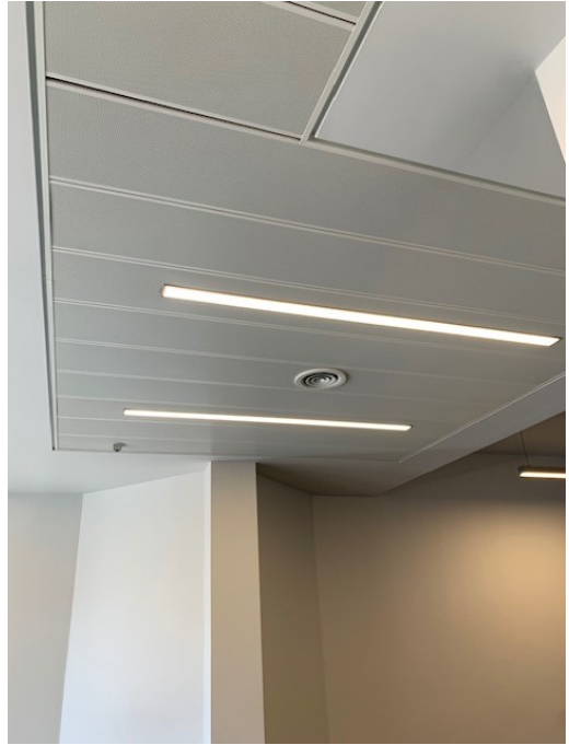
Figure 3.18: Office space, First Floor
