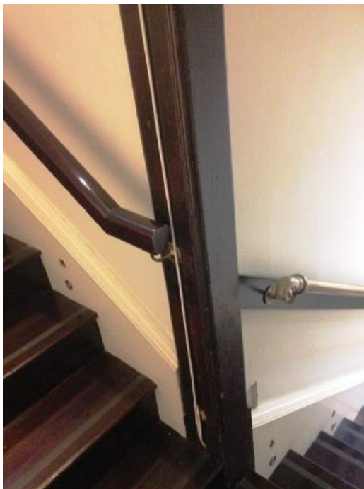
Figure 3.3: Handrails between ground and first floors
