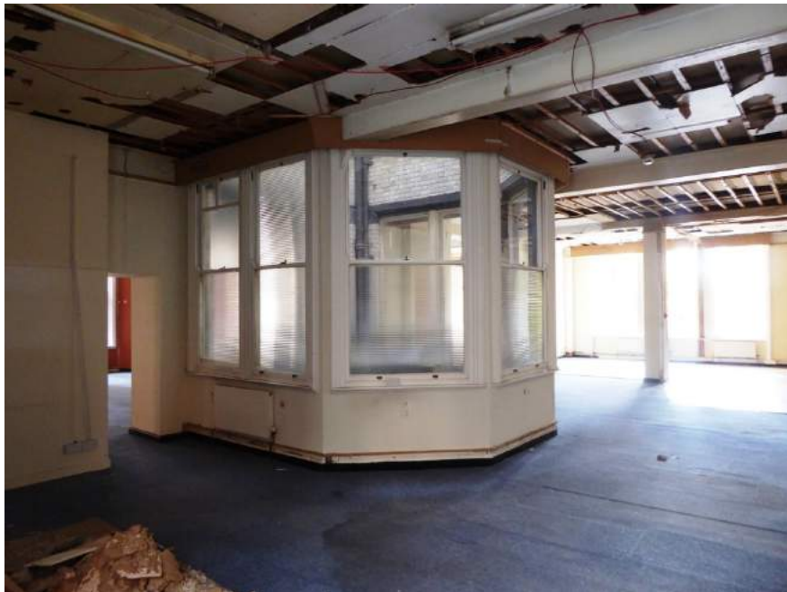
Figure 3.9: Office space, First Floor
