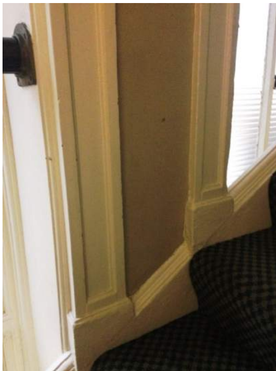
Figure 3.7: Juncture between pilaster and skirting between first and second floor
