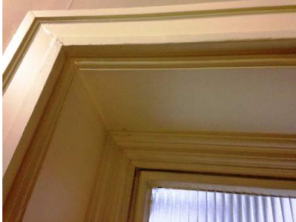
Figure 3.6: Juncture between pilaster and window surround between first and second floor
