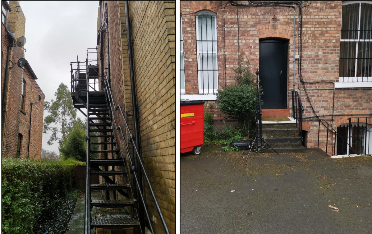
Figure 4: Monitoring Location A (left) and Location B (right) views
