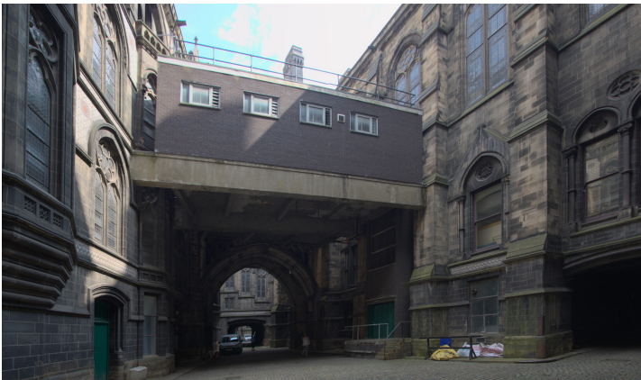
Current condition from Princess Street Courtyard
