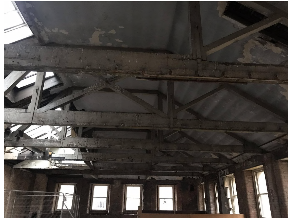
Figure 2.1: Photograph of Roof Trusses
