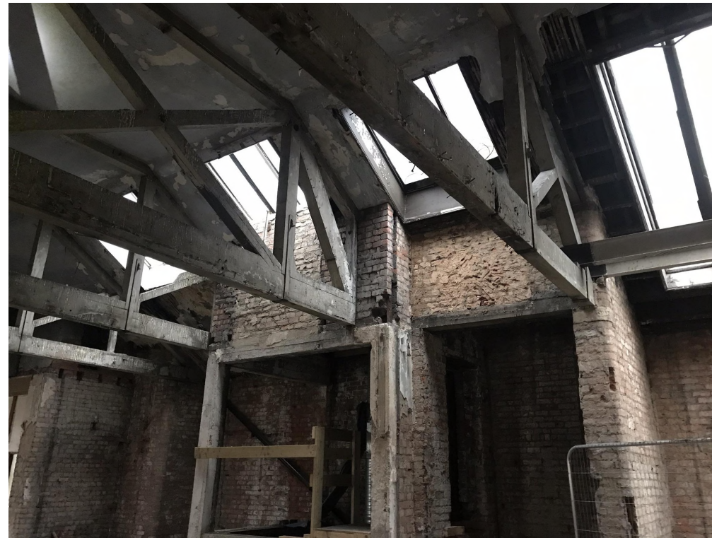
Figure 2.3: Photograph of Concrete Encased Steelwork
