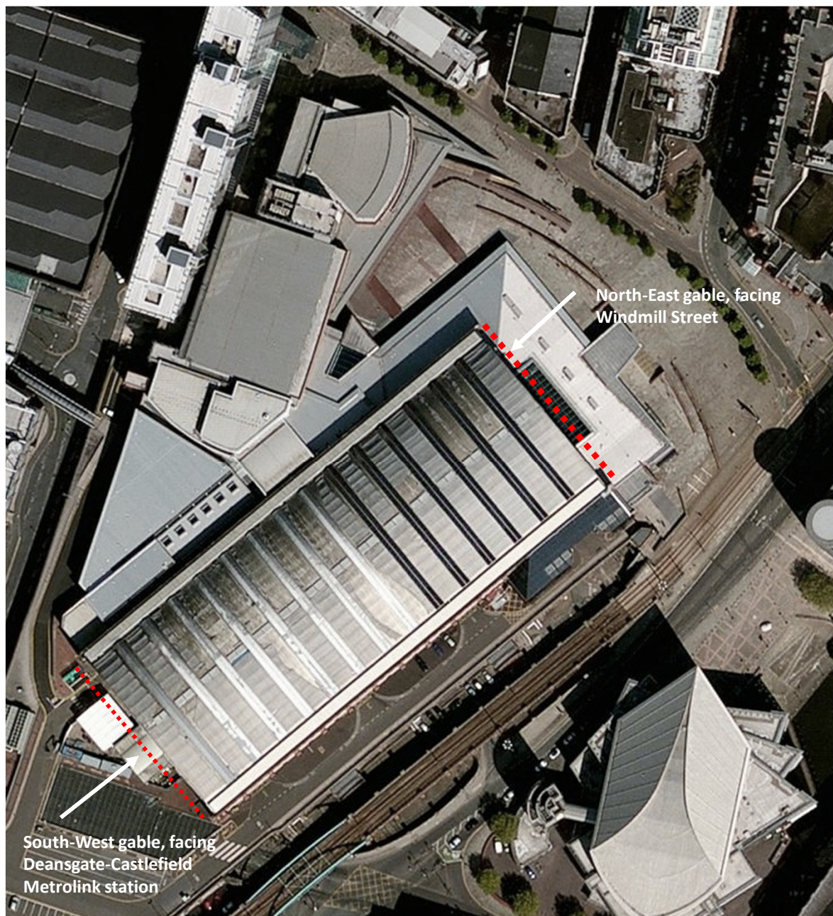
Manchester Central Convention Centre – Roof view indicating gables location
