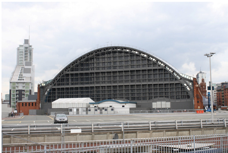
Manchester Central South-West (rear) gable view
