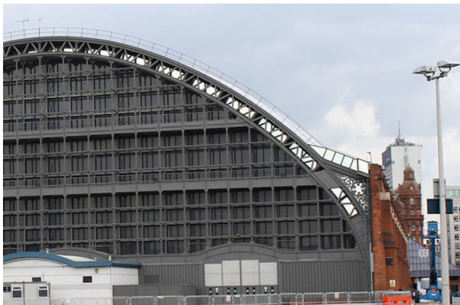
Manchester Central South-West (rear) gable view
