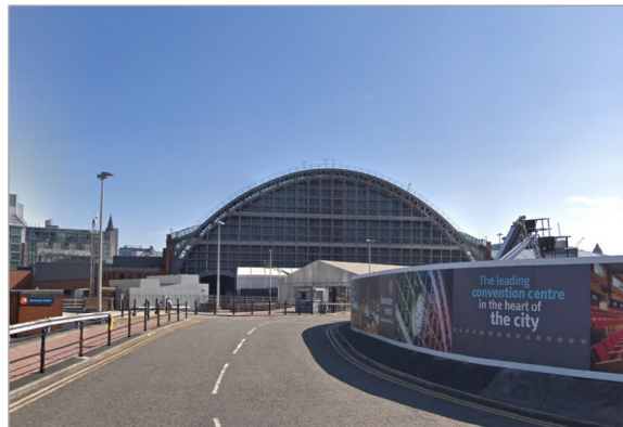
Image 04 – View from Deansgate metrolink station
