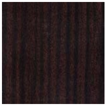
(L) Dark Timber Screening Timber panels located on substation
