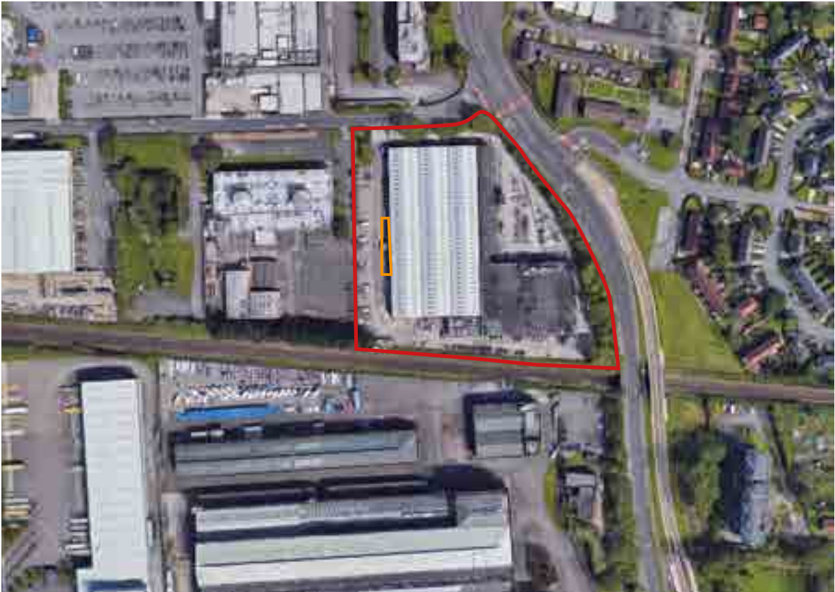
Figure 2. The aerial photograph identifies the Virgin Media site and application boundary.
