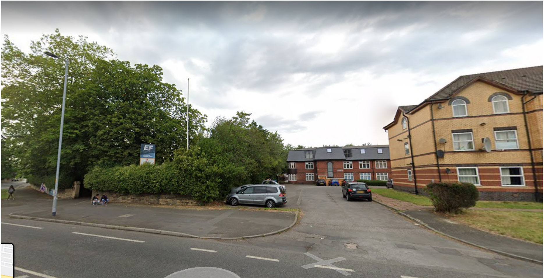
View of proposed siting to the left of residential flats and access road
