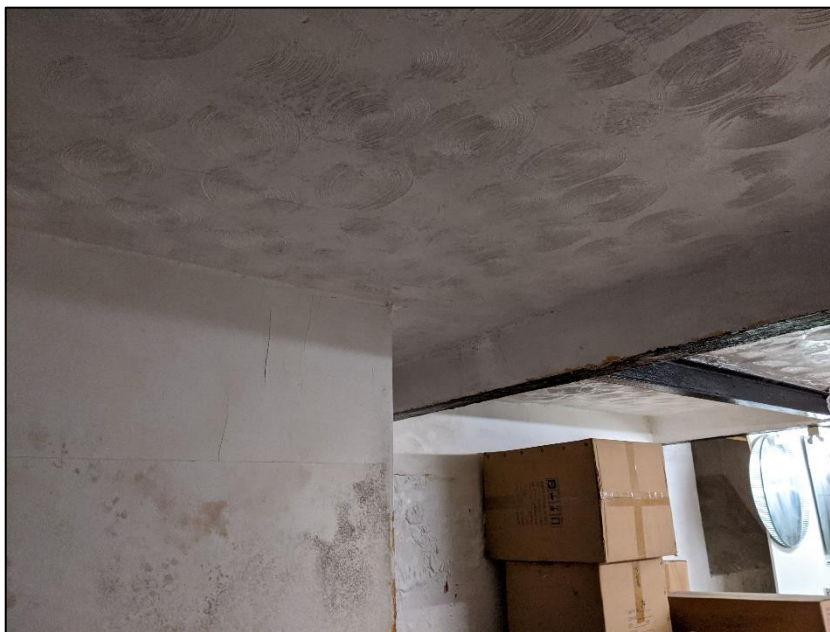
Photograph 7 showing the basement
