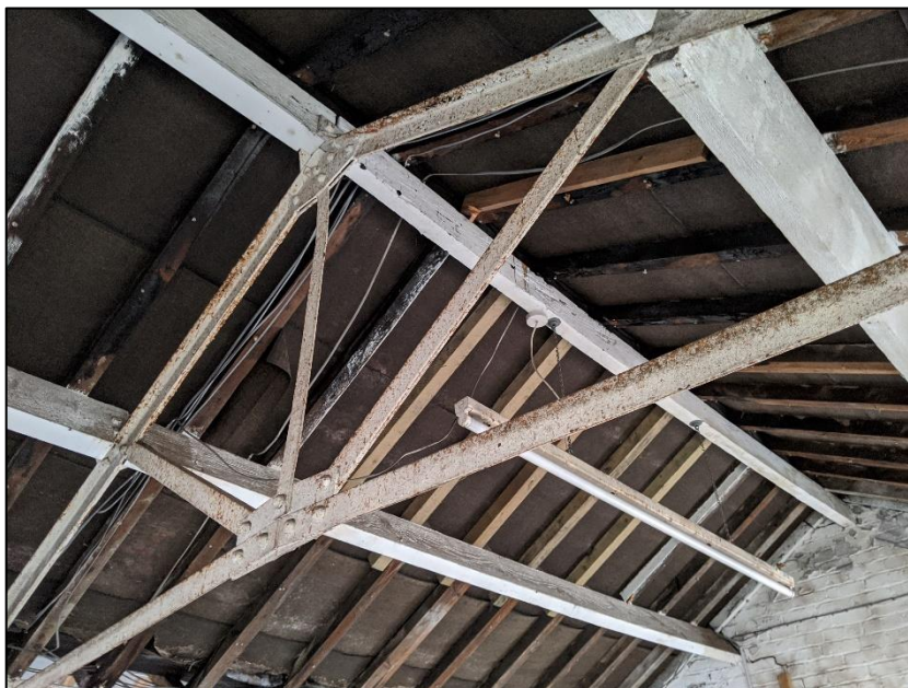
Photograph 3 showing the roof structure of the upper floor
