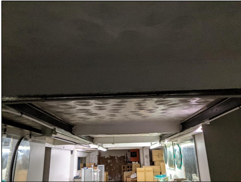
Photograph 6 showing the basement
