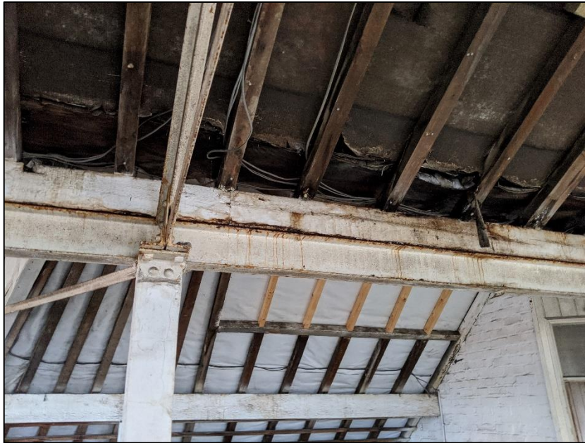
Photograph 4 showing the roof linings
