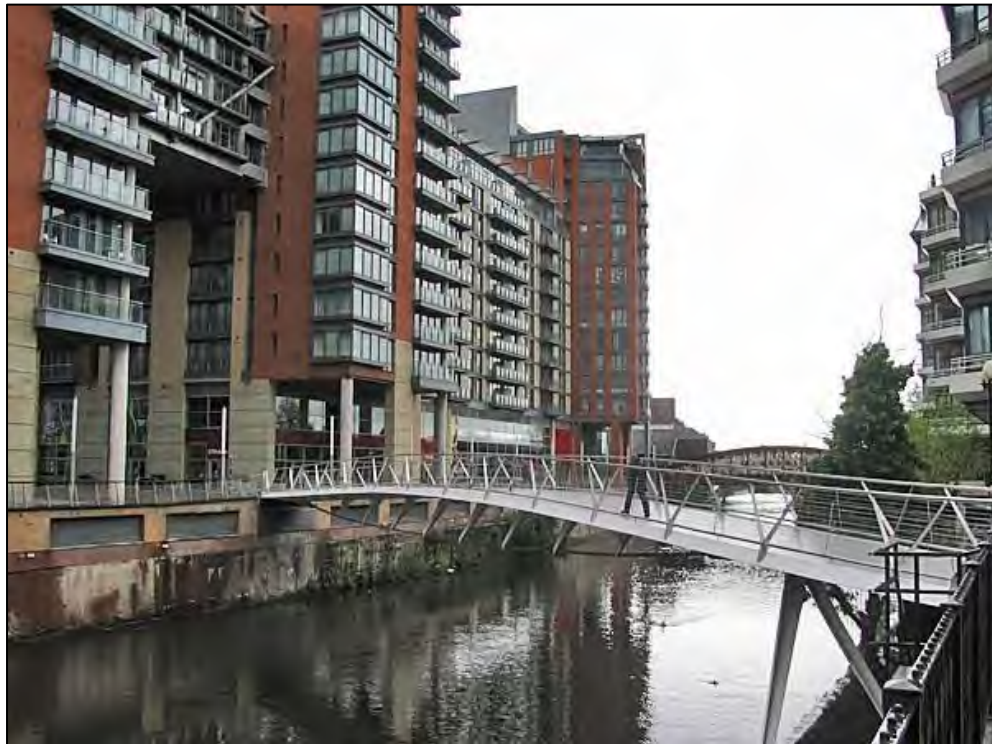
Figure 3.1 Irwell Pedestrian Footbridge
