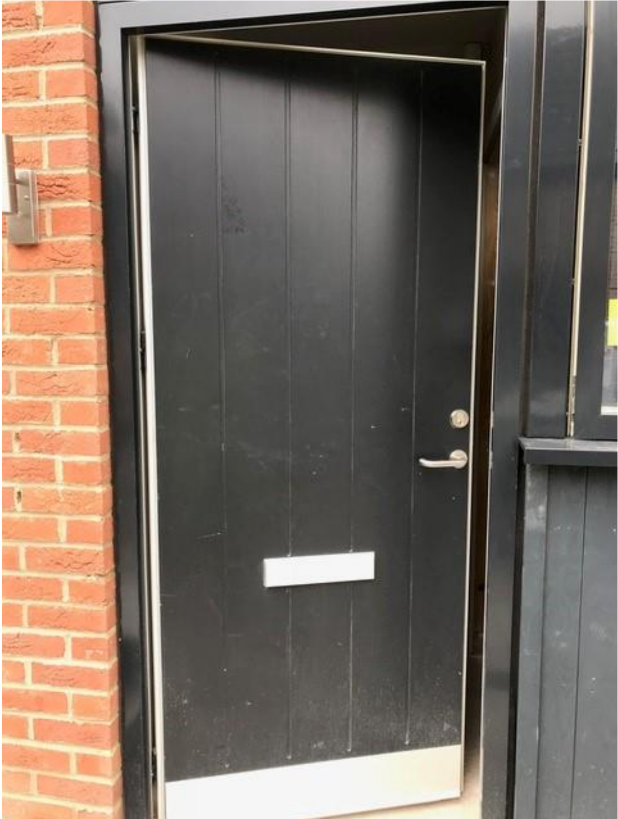
Insert 4: Velfac composite insulated entrance door
