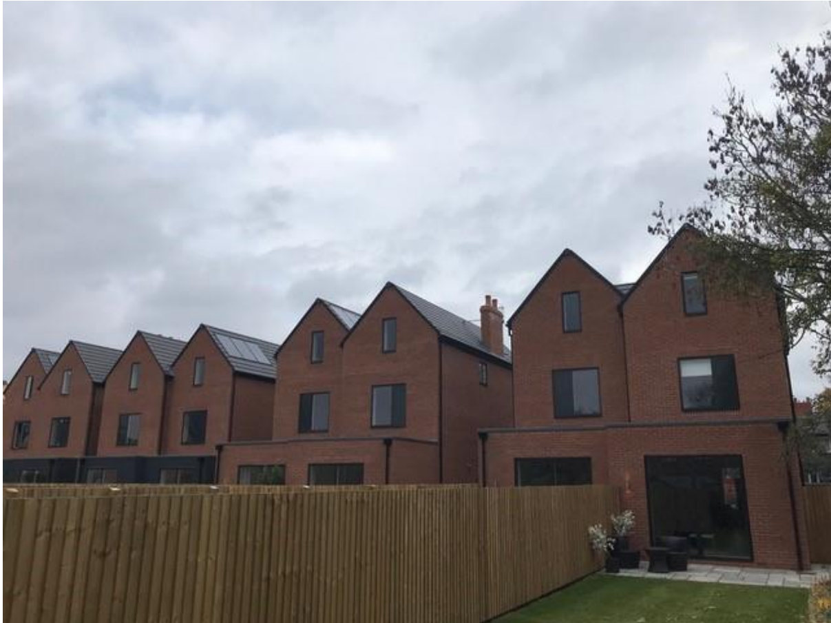
Insert 1: Solar Photovoltaic Panels installed to selected roof areas.
