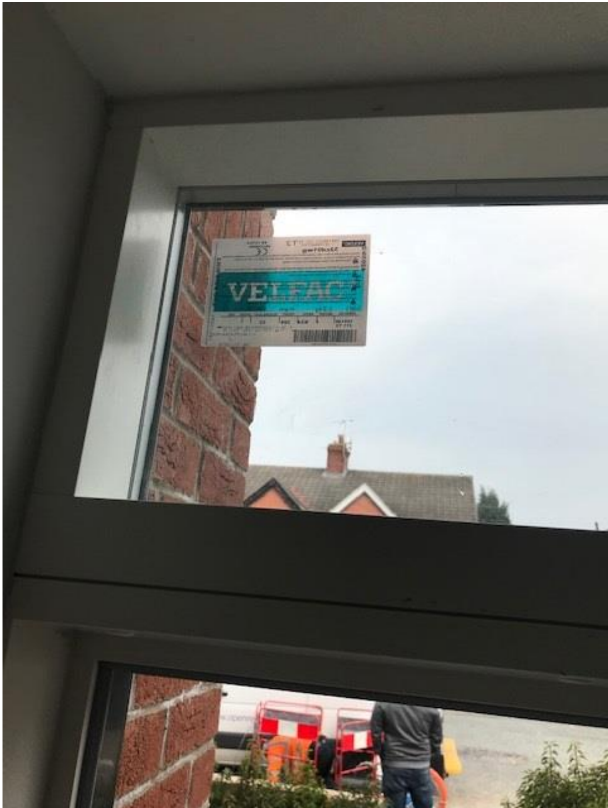
Insert 3: Velfac double glazed window with U value 1.55
