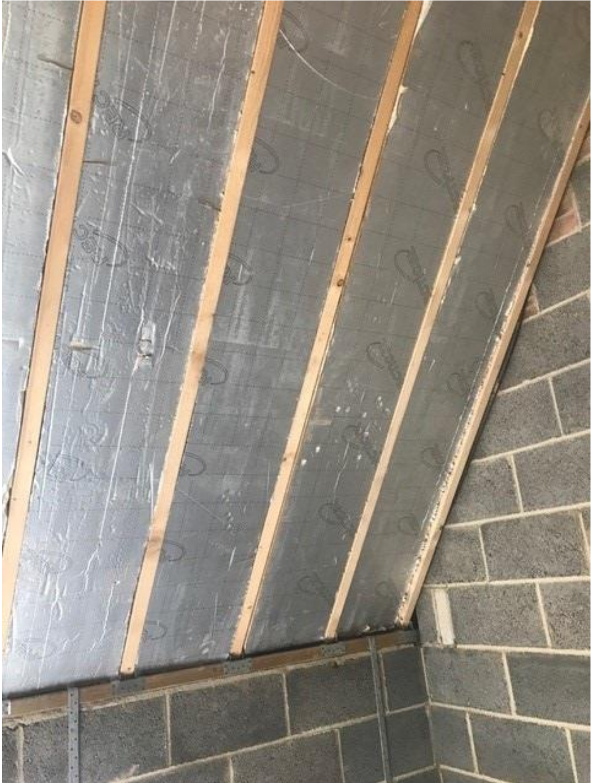
Insert 2: Insulation Board installed between roof rafters.
