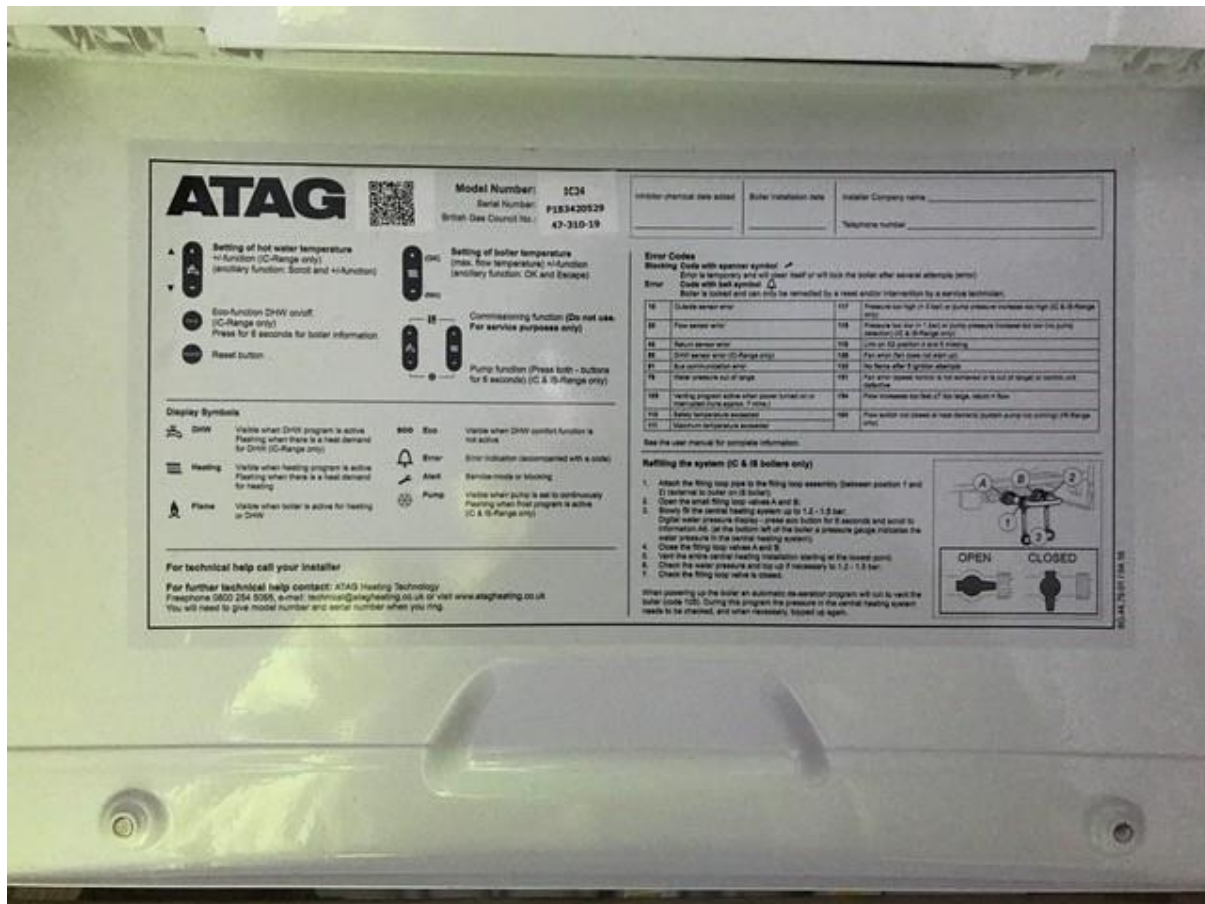
Insert 5: Mains Gas Boiler Identification label
