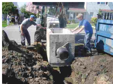
Smaller Smart Filter® being lowered into position
