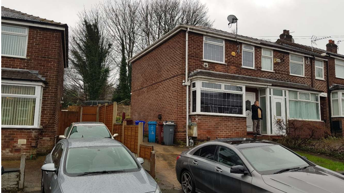
Rear Elevation – Kathkin Ave elevation – showing gable elevation of No.16
