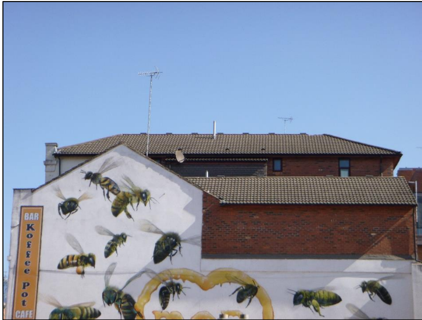
Photograph 3 showing the roof of the property
