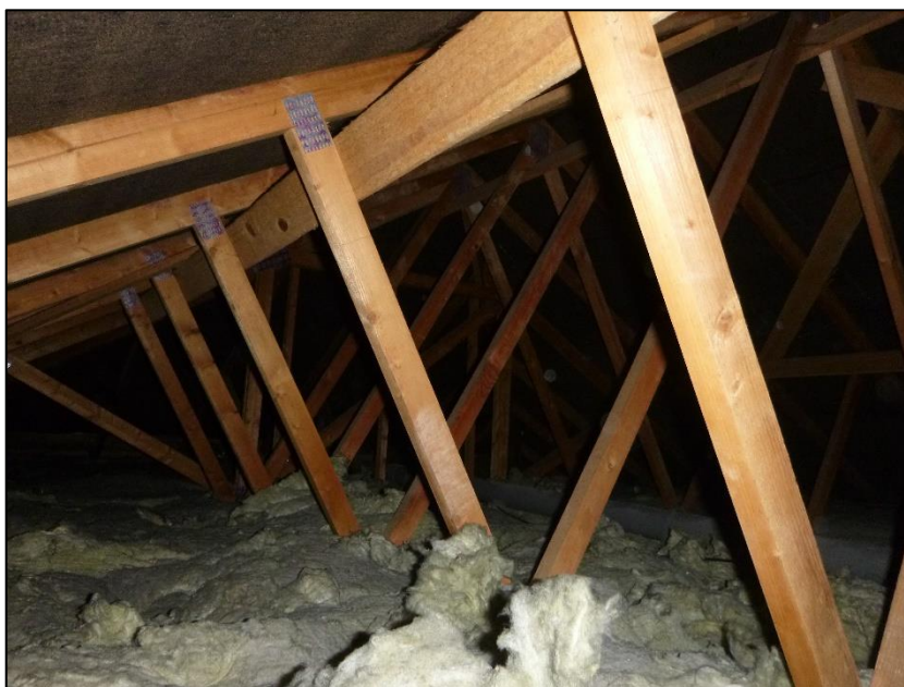
Photograph 4 showing the roof joists
