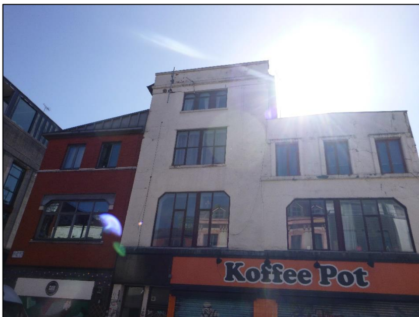
Photograph 2 showing the front elevation
