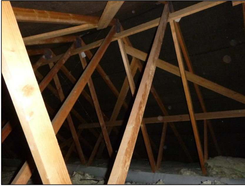
Photograph 5 showing the roof void
