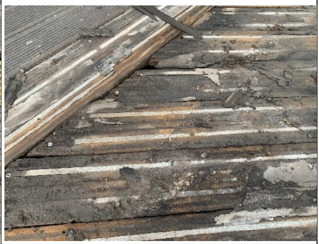
Deterioration of Wooden Flooring Beneath Non-Slip Covering of Boardwalk
