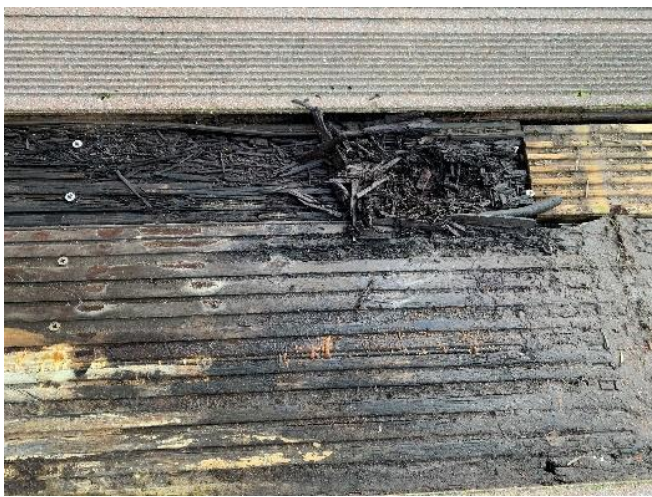
Deterioration of Wooden Flooring Beneath Non-Slip Covering of Boardwalk
