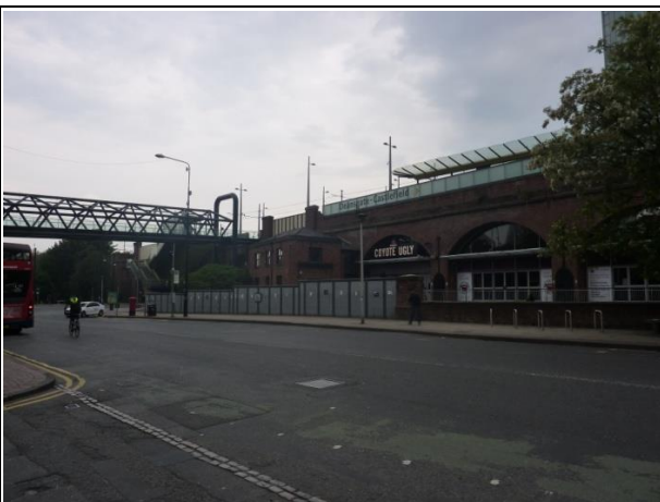
View Northwest Towards Lock Keepers Cottage
