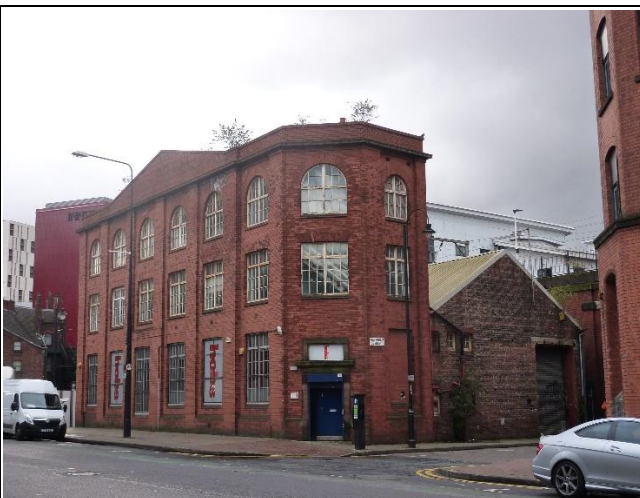
Whitworth House With Viaduct to the Rear
