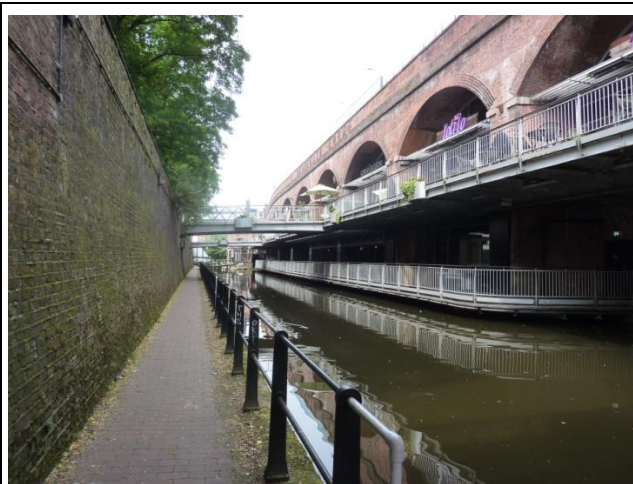
View from Lock 90 Looking West Showing Upper and Lower Walkways
