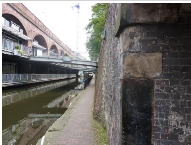
View from Canal Level Towards Lock 90 Showing Upper and Lower Walkways
