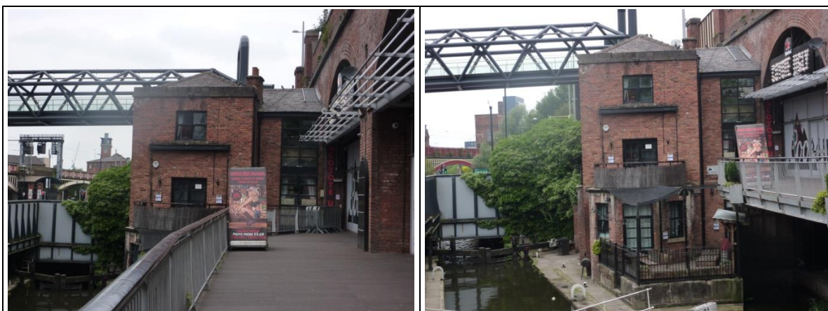
Lock Keepers Cottage East Elevation
