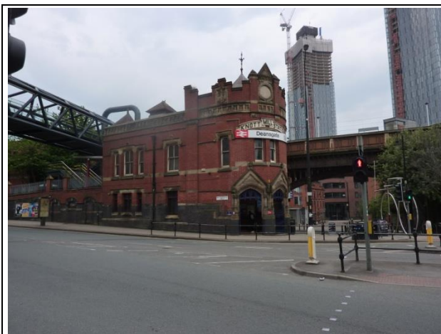
Deansgate Station North Elevation
