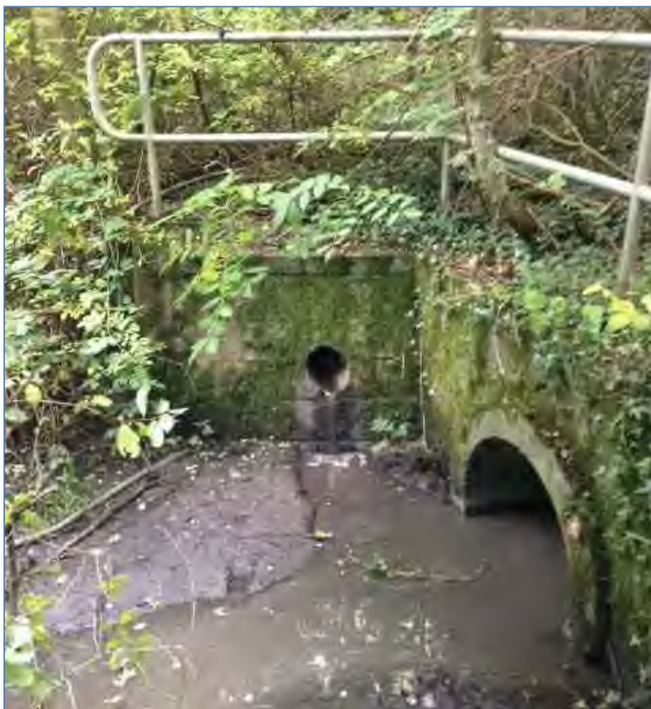
Figure 1.8 – Headwall with 900Φ and 225Φ outlets
