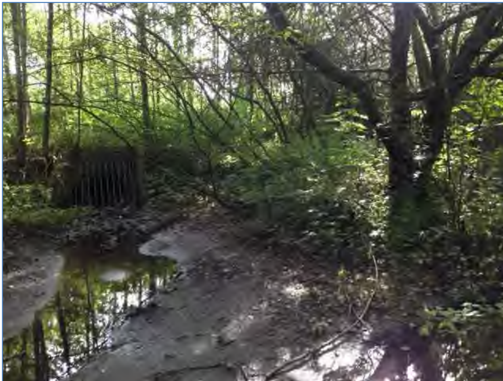
Figure 1.5 – Goodmans Headwall with 900Φ pipe outlet
