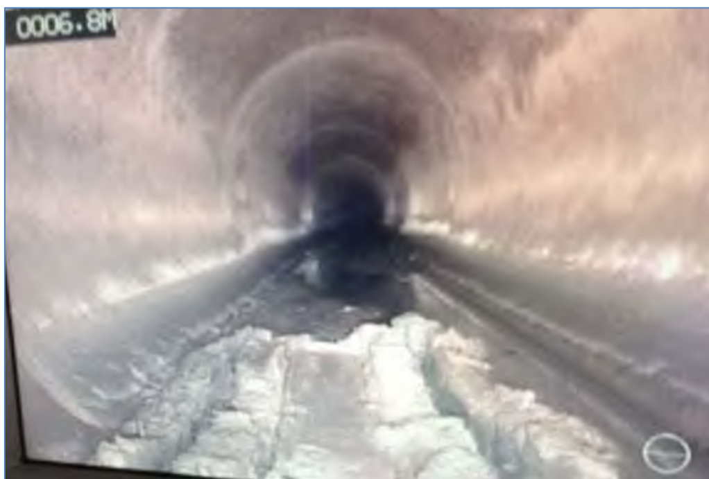
Figure 1.9 – Interior of the 1000 \Phi pipe
