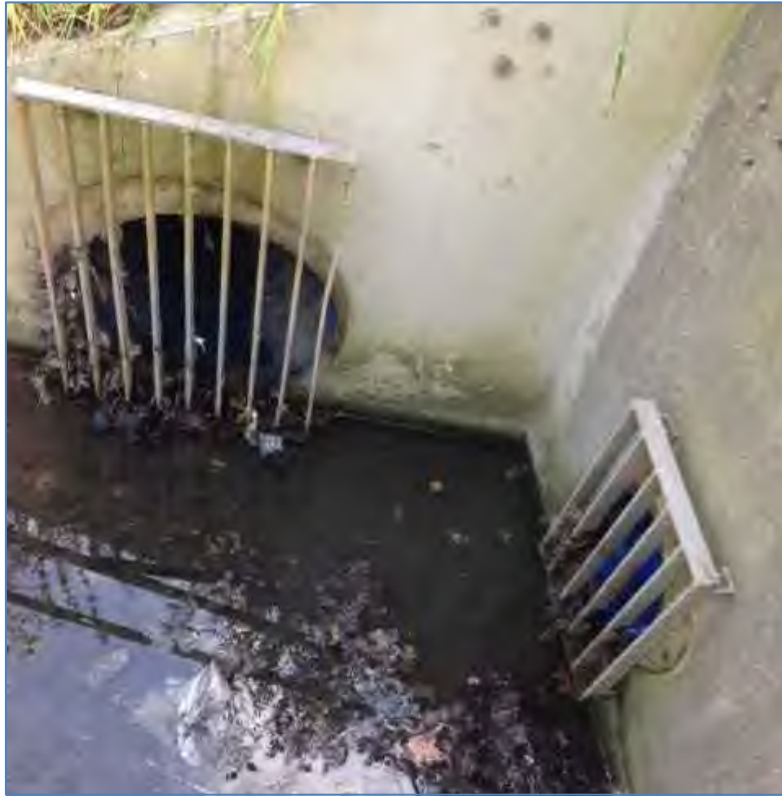
Figure1.4 – Headwall installed during Metrolink works with 300Φ and 450Φ outlets
