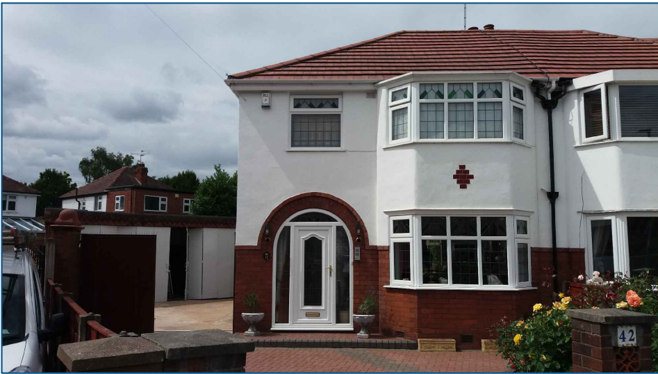
PHOTOGRAPH No3 (FRONT ELEVATION & PART GARAGE)
