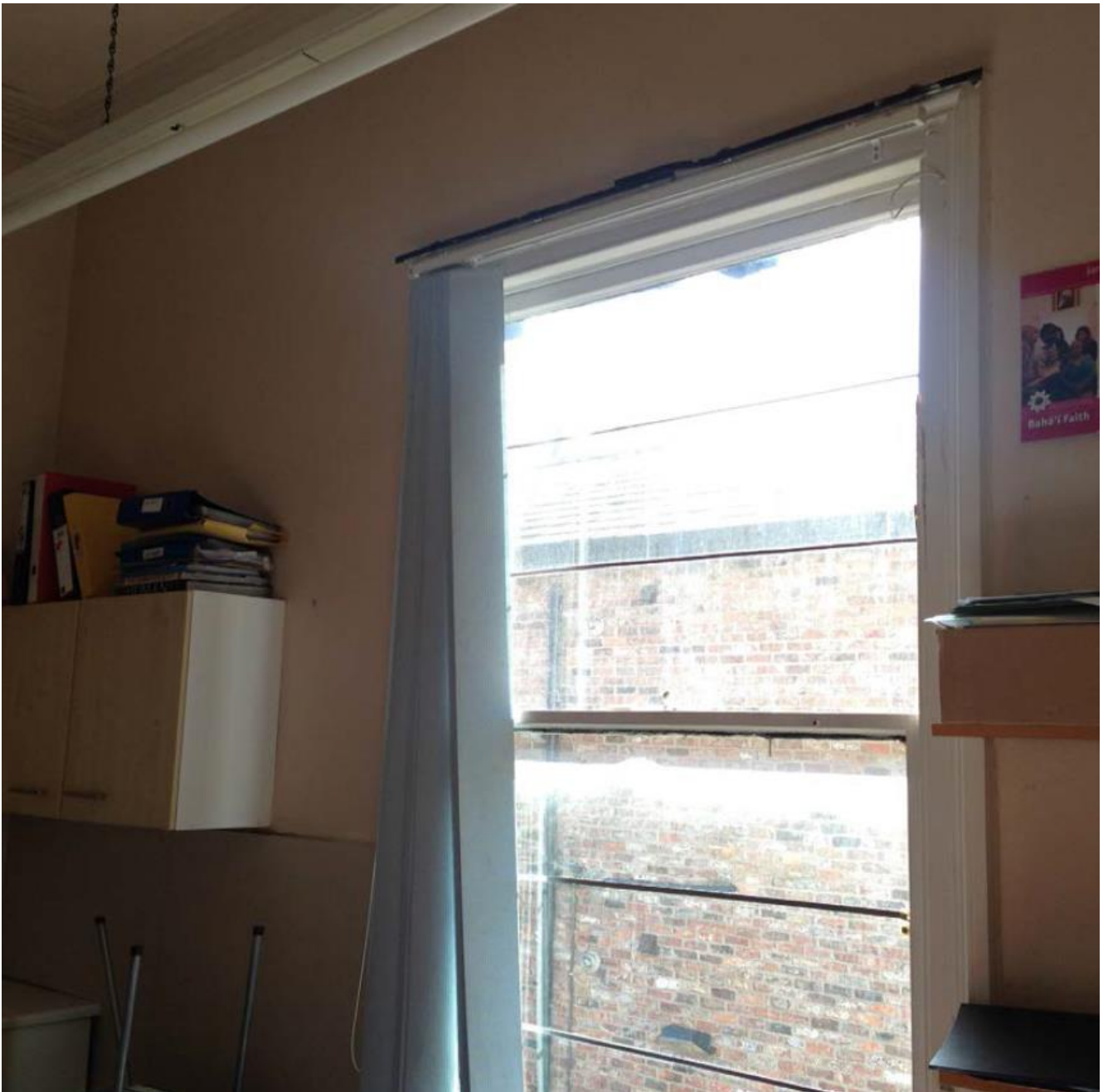
Plate 12: First Floor Window, provided by Orco Heritage Statement 2014 (revised 2016)
