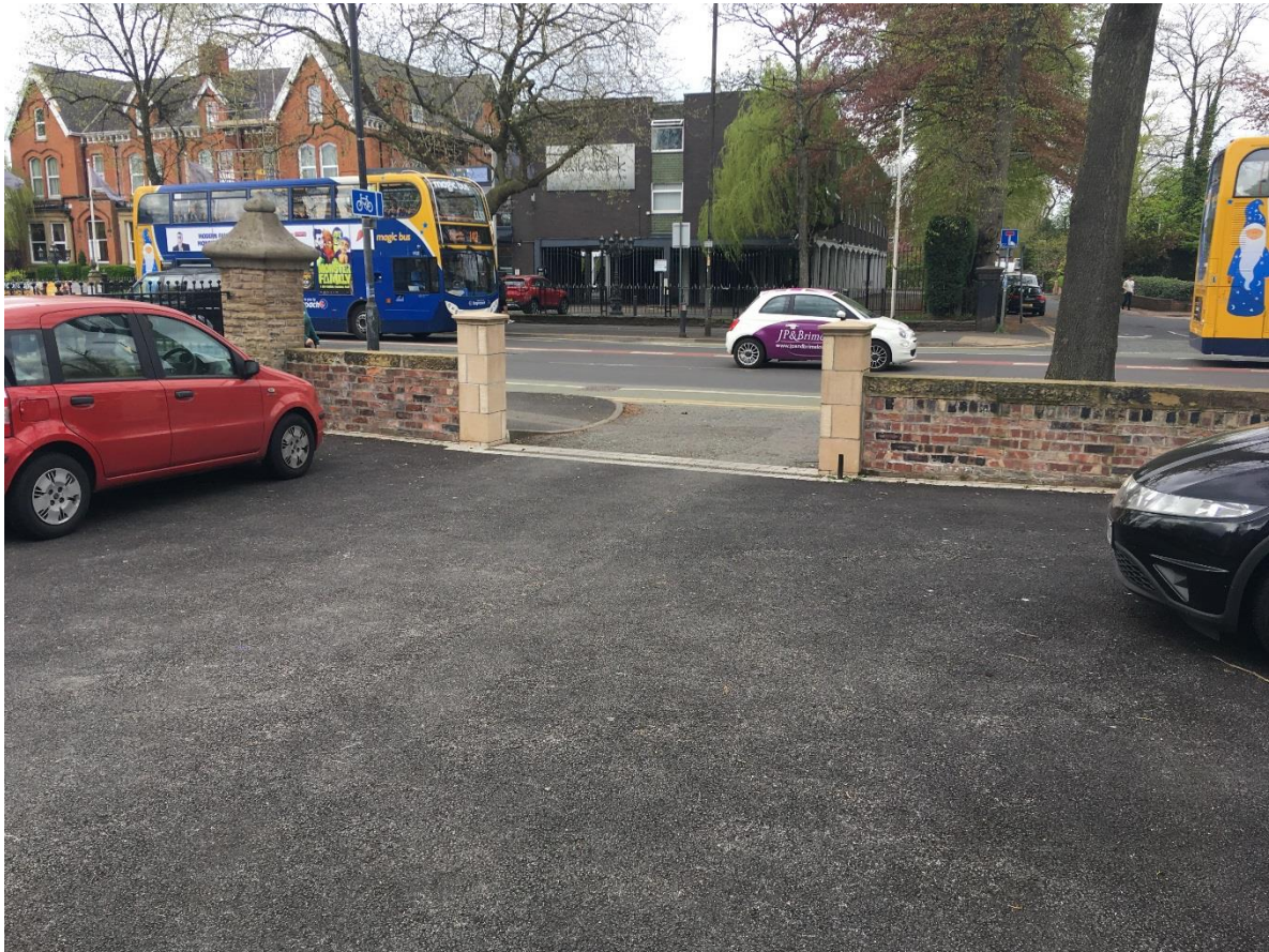
Plate 25: Rebuilt Entrance Piers and tarmacadam parking area
