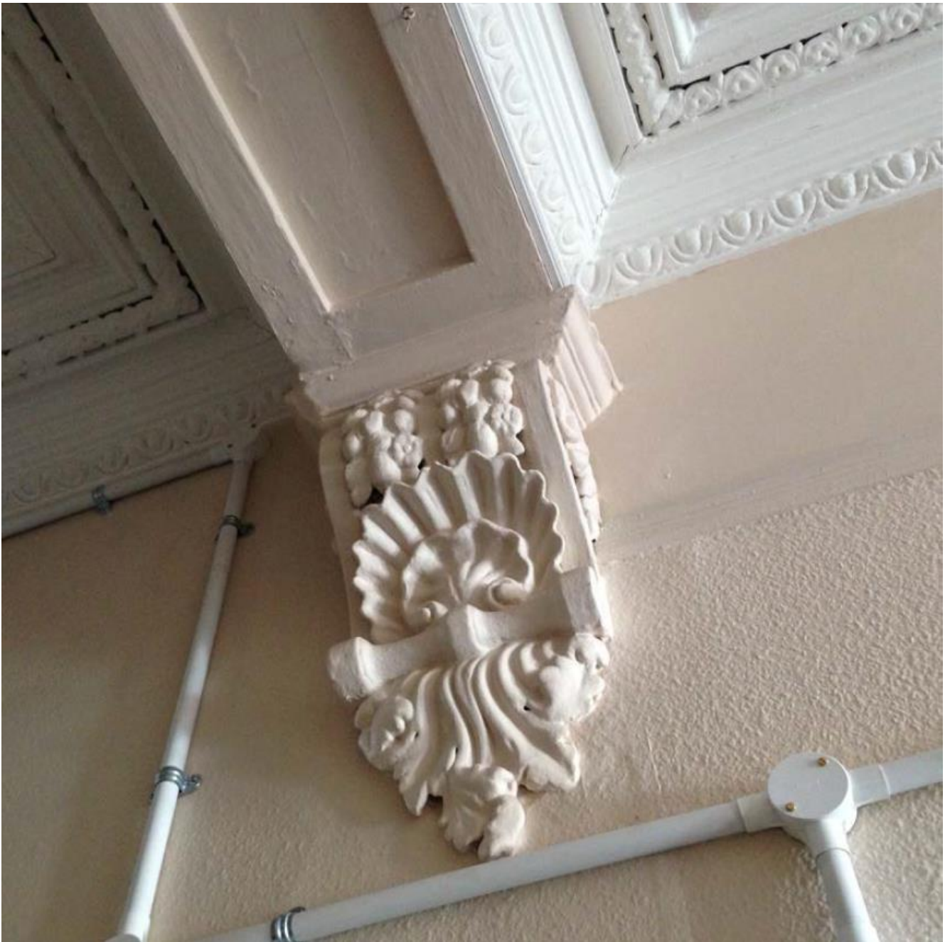
Plate 5: Plasterwork in main hallway, provided by Orco Heritage Statement 2014 (revised 2016) prior to conversion to flats, also shows applied electrical conduits
