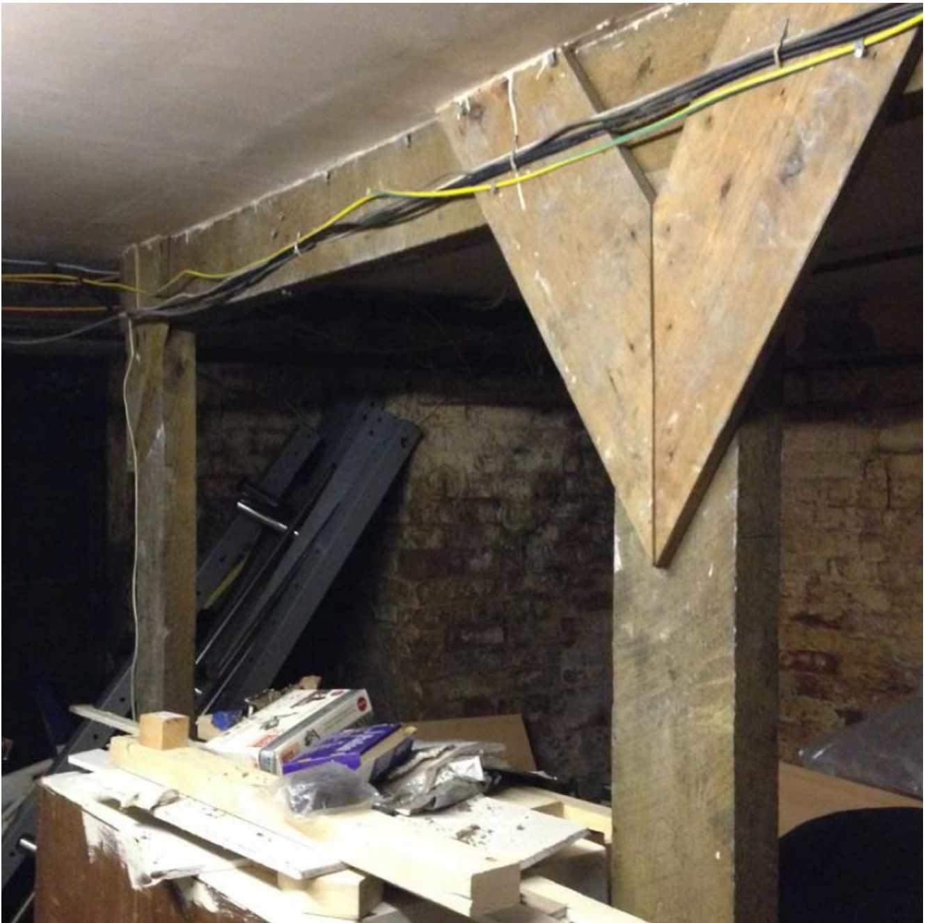
Plate 3: Exposed Brickwork and Electricals in Basement, provided by Orco Heritage Statement 2014 (revised 2016)
