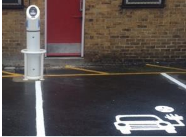
Fig 3.2 – Floor mounted post on concrete plinth in tarmac parking bay with bay marking
