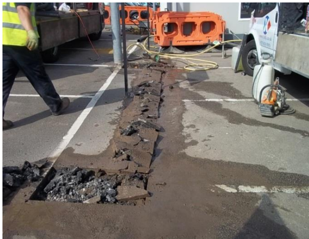
Fig 3.5 – Post Foundations being dug
