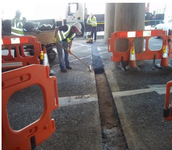
Fig 3.9 – Reinstatement Road Surface with Existing Material Type
