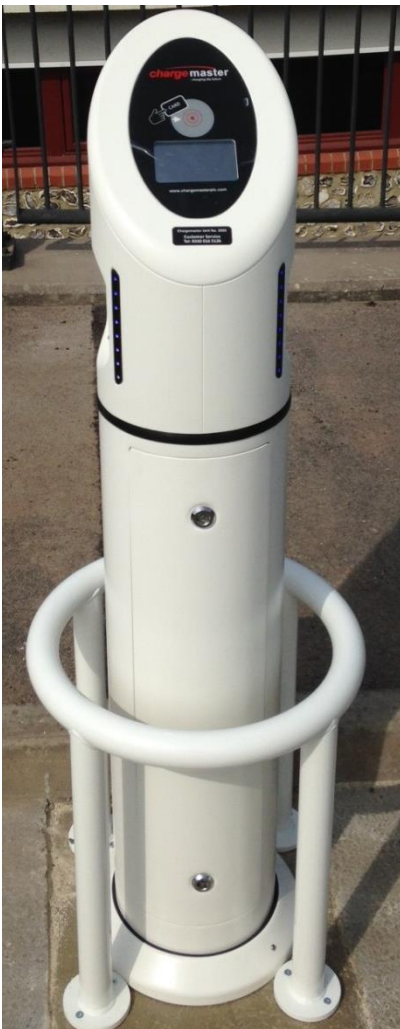
Fig 3.3 – Floor mounted post on concrete plinth
