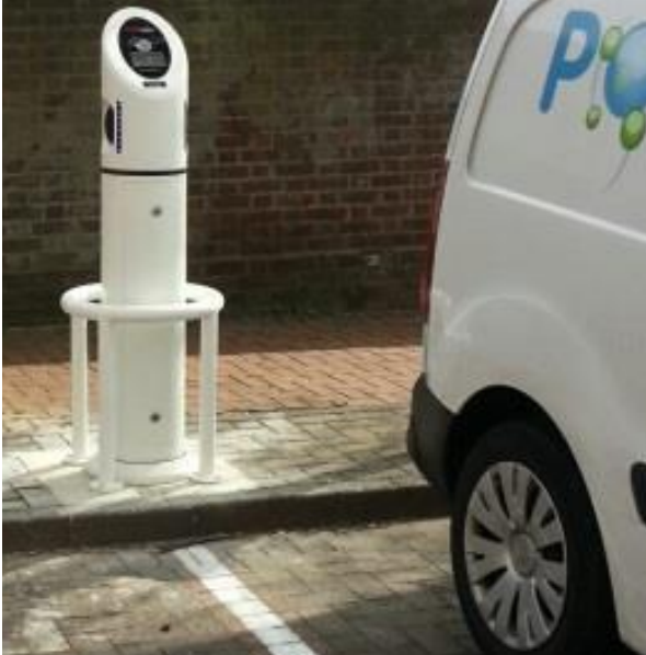
Fig 3.11 – Install of post and guardrail onto concrete plinth within a block paving site
