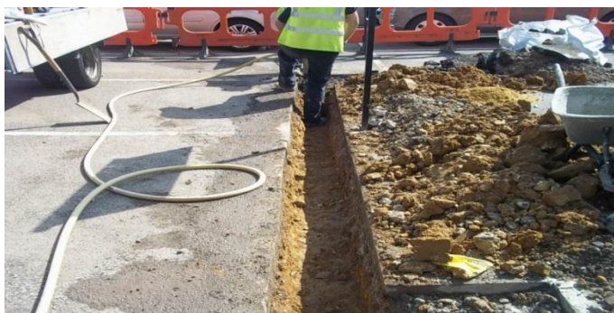
Fig 3.7 – Check Trench Depth and consolidate Base Warning Tape
