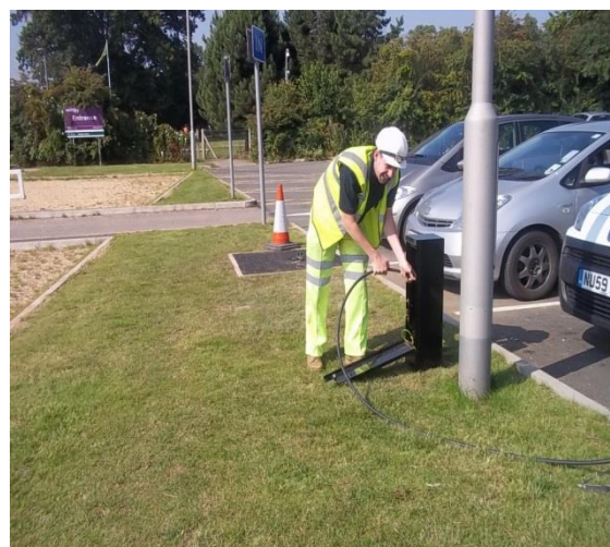
Fig 3.10 – SWA cable being fed through
