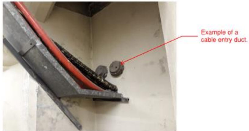
Figure 9 - Existing HV Duct Penetration
