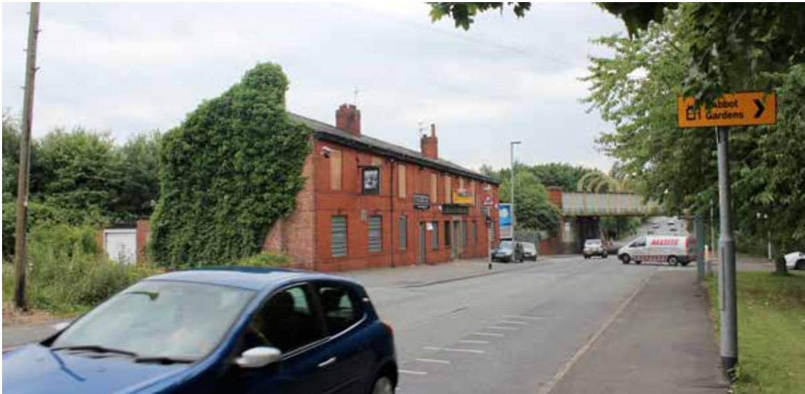
Fig.6 - Photograph illustrating existing front elevation in context
