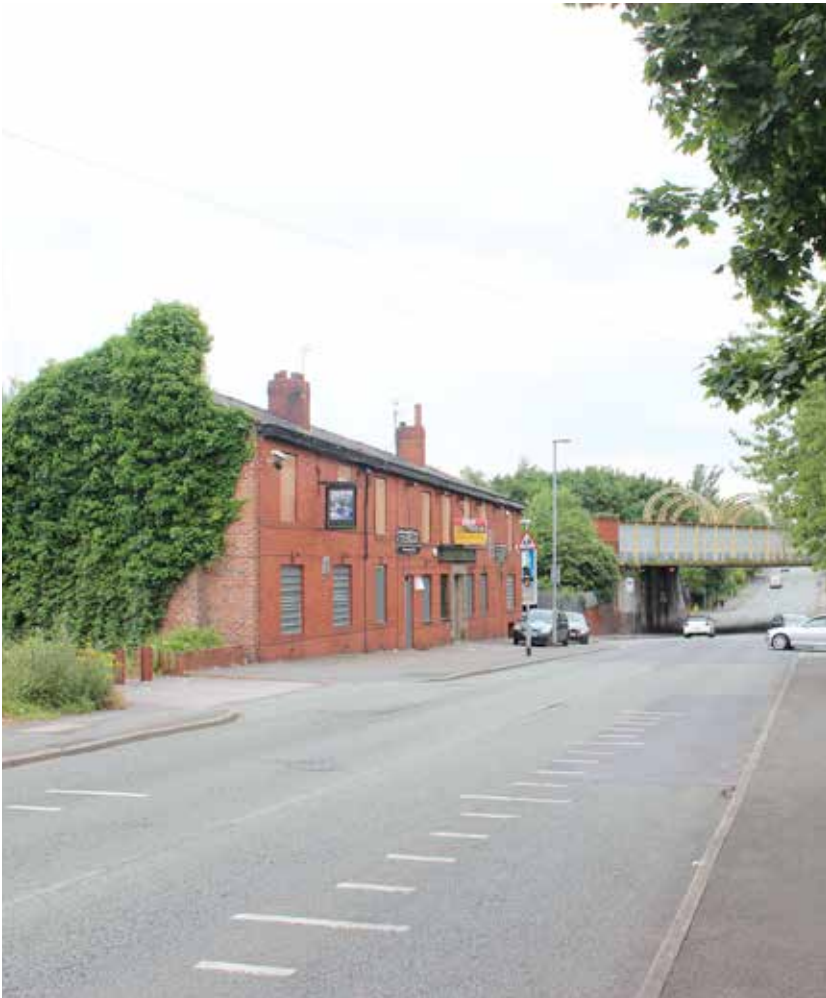
Fig.8 - Photograph illustrating existing front elevation
