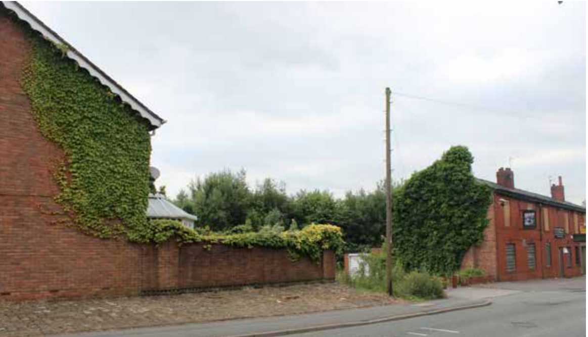
Fig. 7 - Photograph illustrating Adjacent property building height
