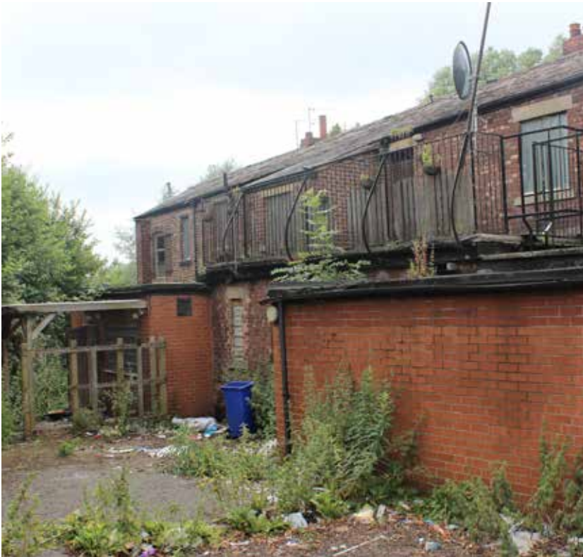
Fig.9 - Photograph illustrating existing rear elevation
