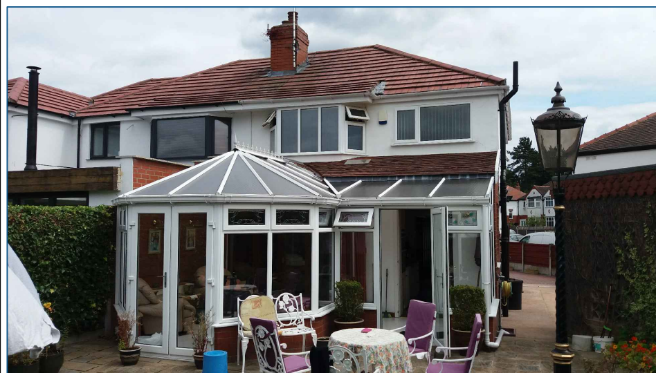
PHOTOGRAPH No1 (REAR ELEVATION & PART GARAGE SIDE)
