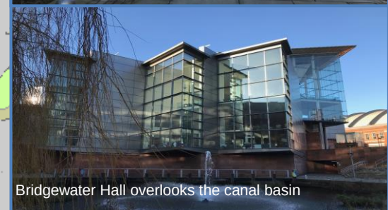
Looking north-west across the front of the premises towards the steps that provide access to the basin and canal-side commercial units
