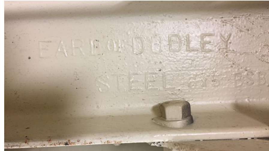
Figure 2 Detail of the steelwork supports (to be removed)
