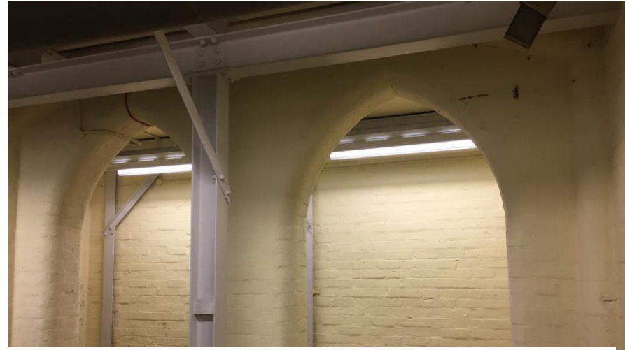
Figure 3 The steel supports (proposed for removal)
