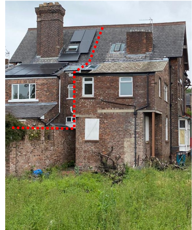
View of the rear where extension would be added
