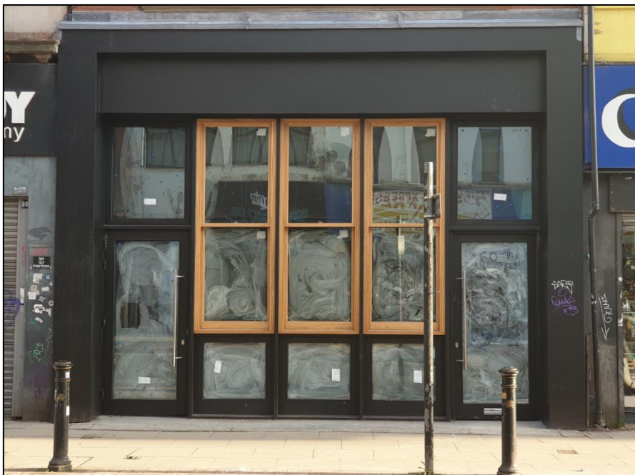
Figure 19: Dark grey aluminium shopfront at 60 Oldham Street.
