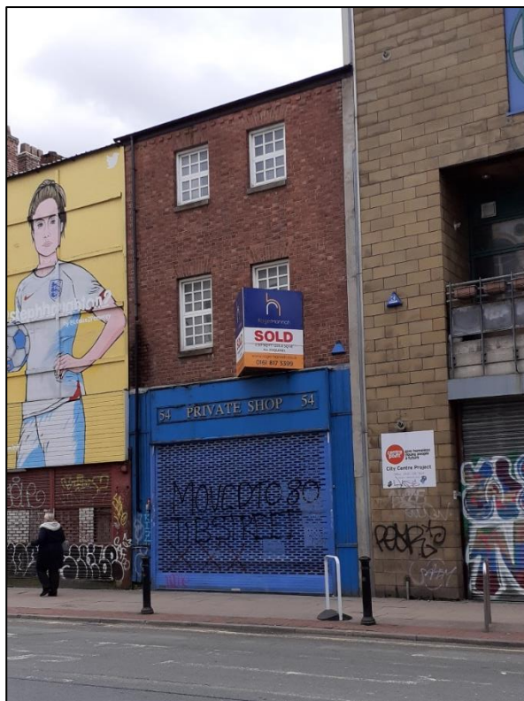
Figure 3: Front elevation of 54 Oldham Street.
