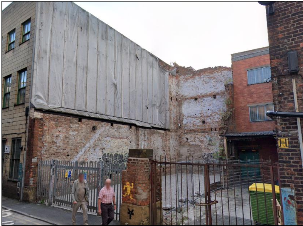
Figure 5: Rear elevation of 54 Oldham Street from Spear Street.
