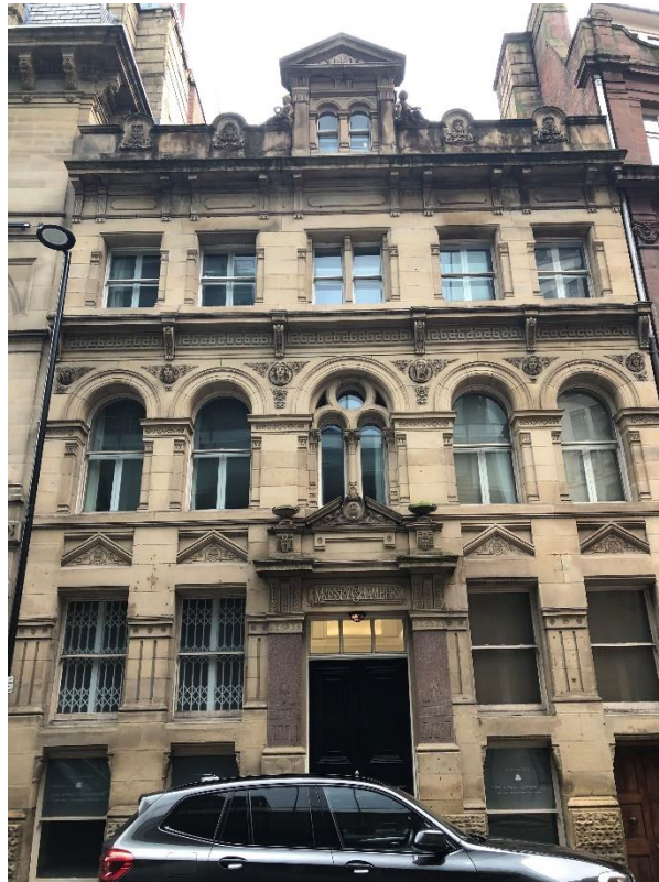
Figure 2: The principal front elevation of Massey Chambers as seen from Booth Street.
