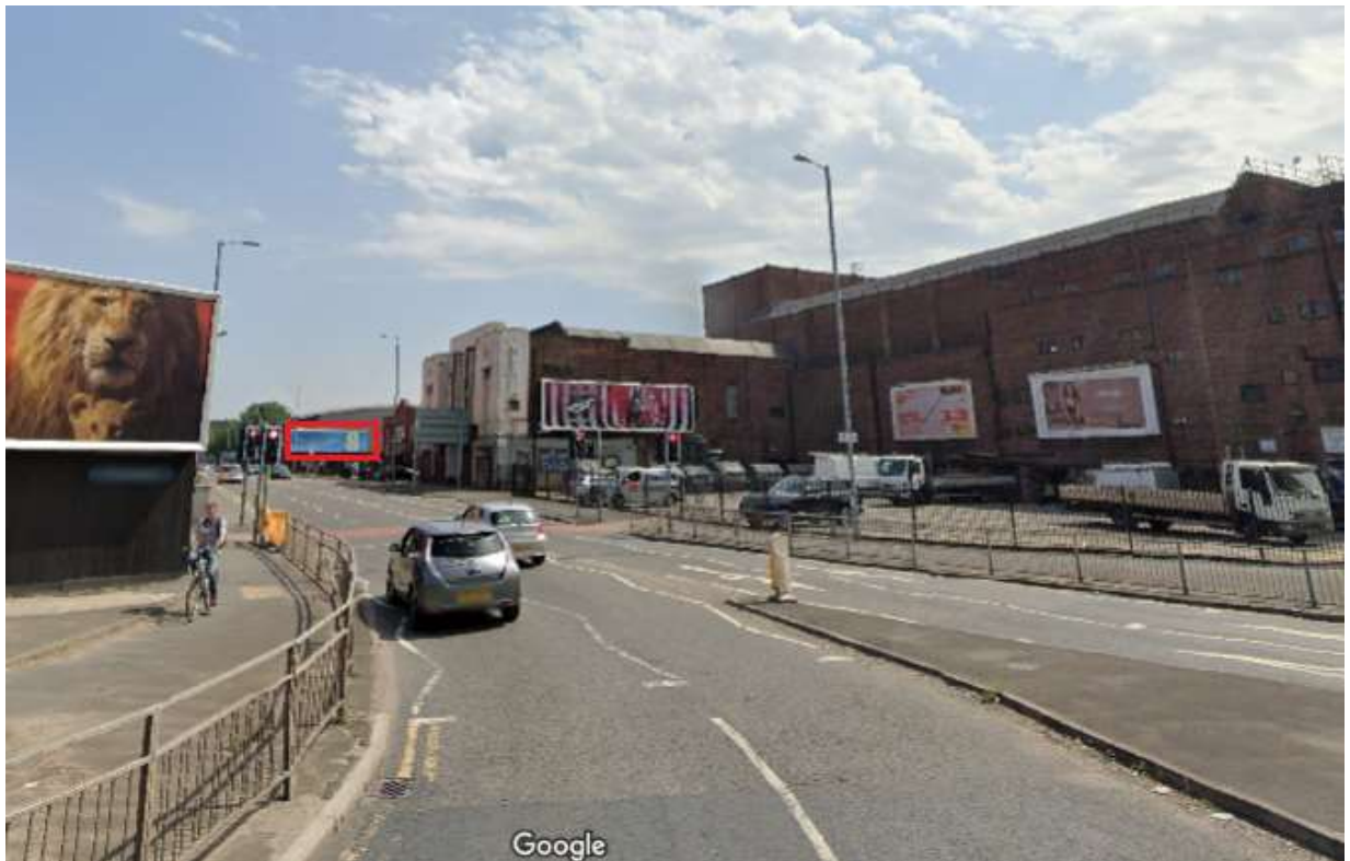
Figure 3.1 – Image Looking Towards the Proposal Site from the A57 Hyde Road Eastbound Carriageway
