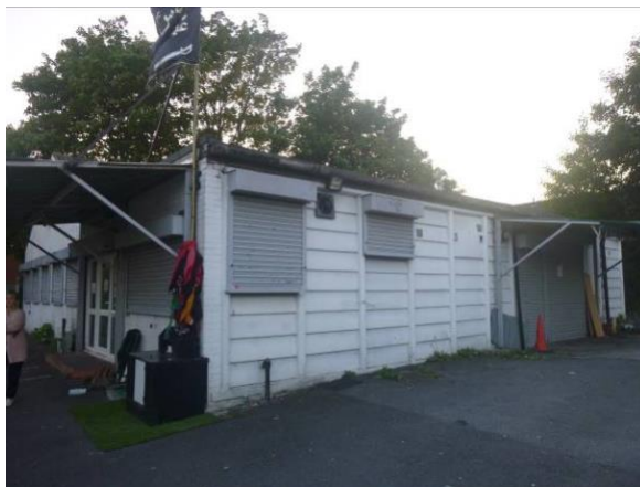
P1 SE corner showing canopies
