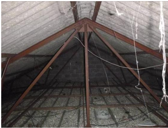
P7 Loft showing unlined roof
