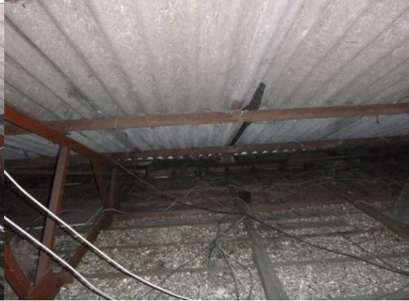
P8 Loft showing daylight at eaves
