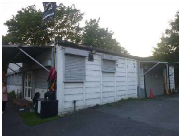
P1 SE corner showing canopies
