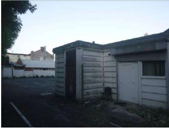
P5 Boiler house
