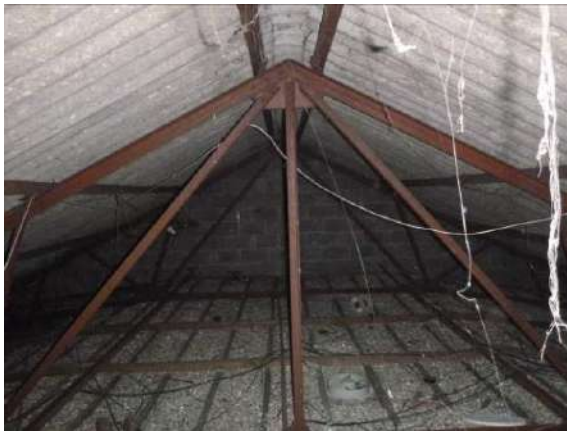
P7 Loft showing unlined roof
