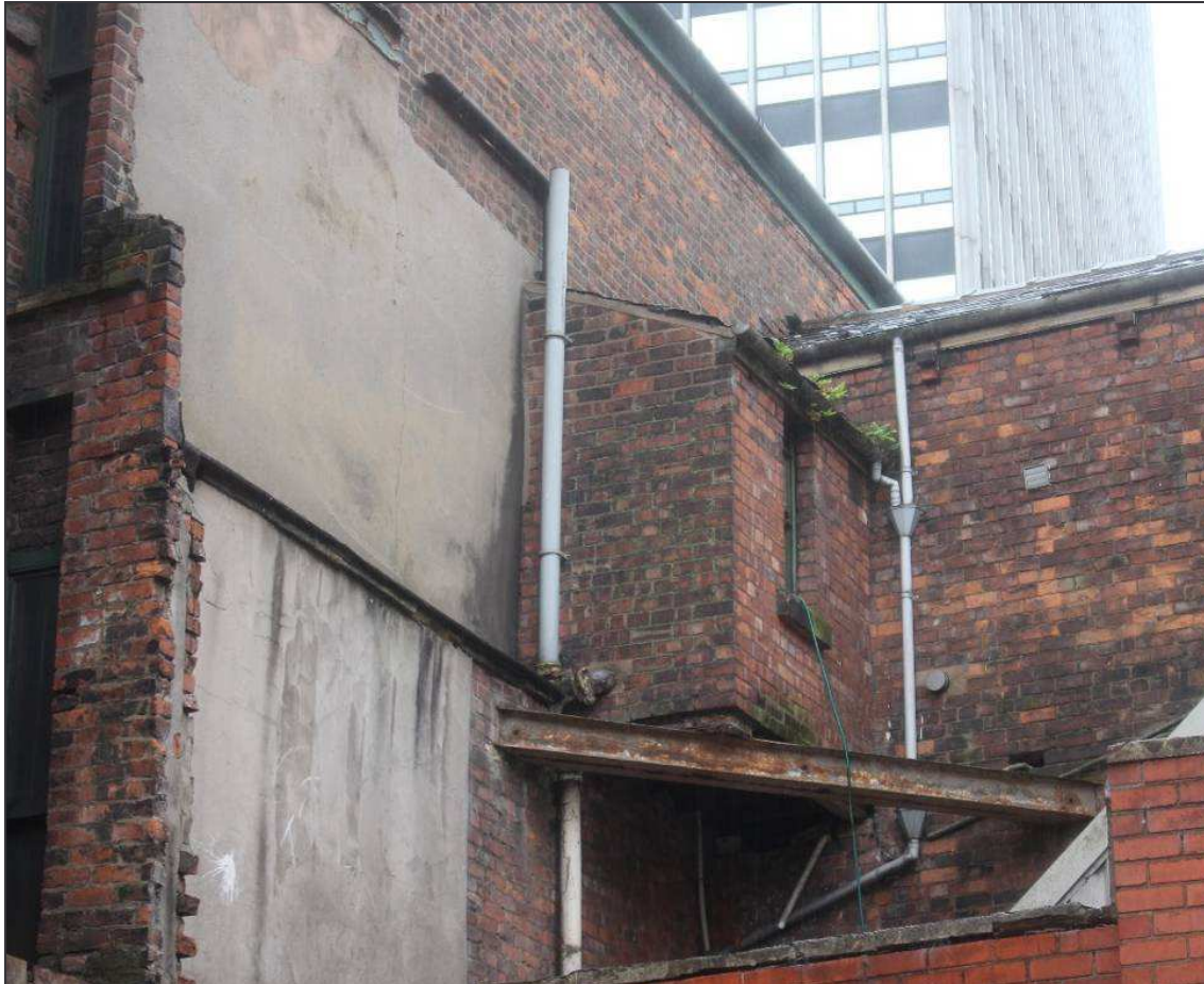
Plate 27: Detail of the first-floor extension to the north-east façade
