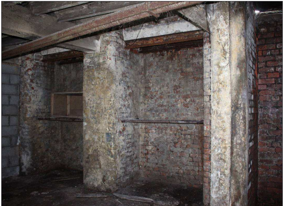
Plate 108: Detail of the recessed window apertures within the south-east wall
