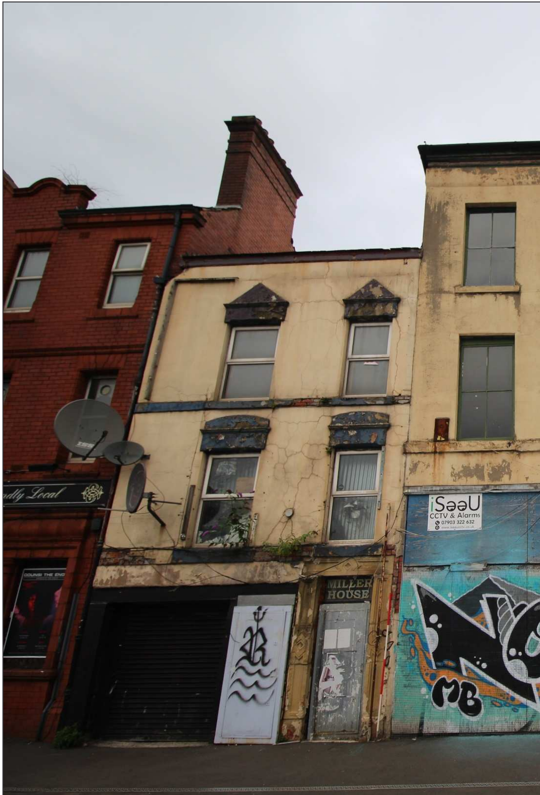
Plate 21: The south-western façade of the 88a Miller Street
