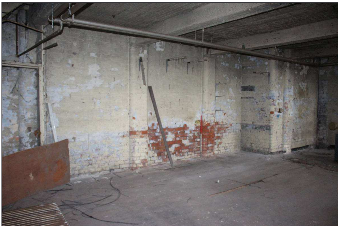
Plate 103: Detail of the blind recesses within the north-west wall
