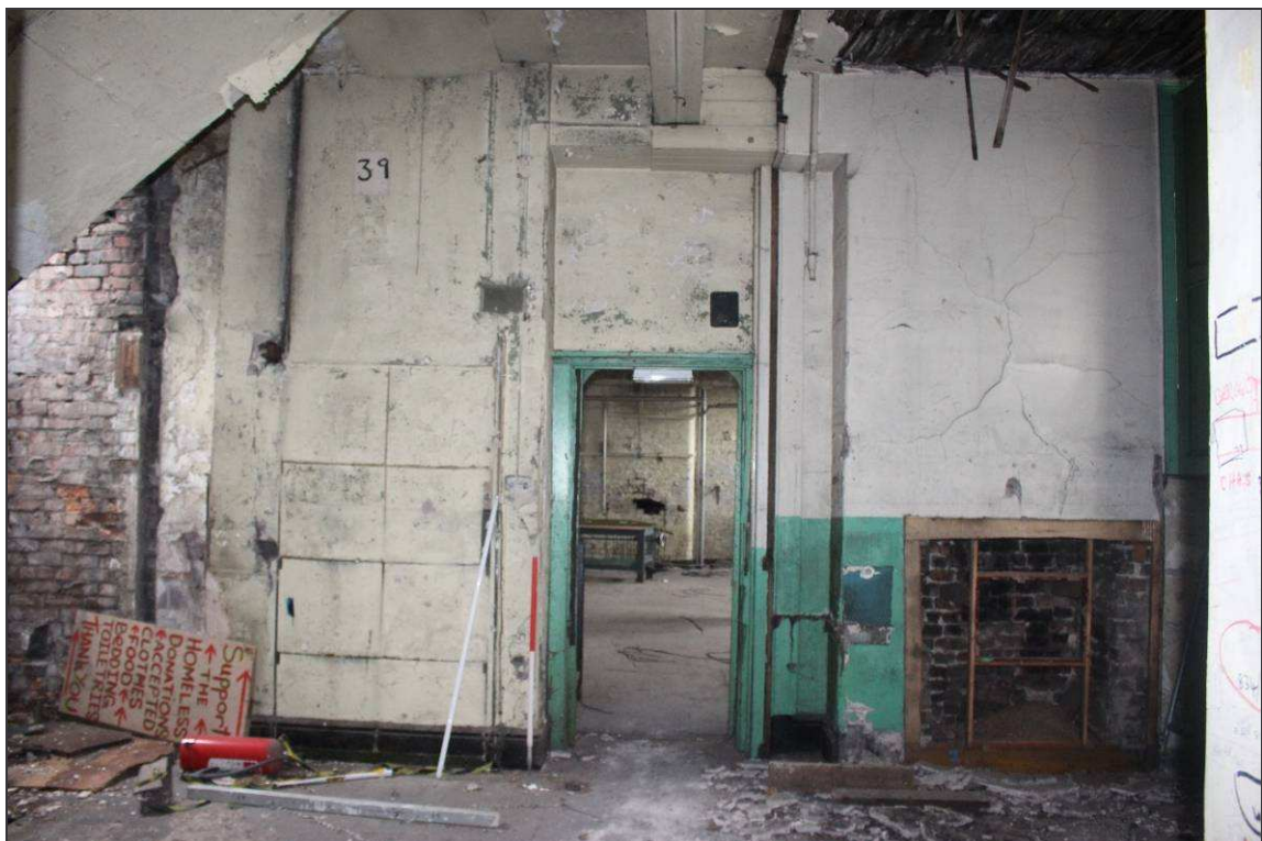
Plate 99: The doorway within the north-eastern wall leading into the later extension of the warehouse
