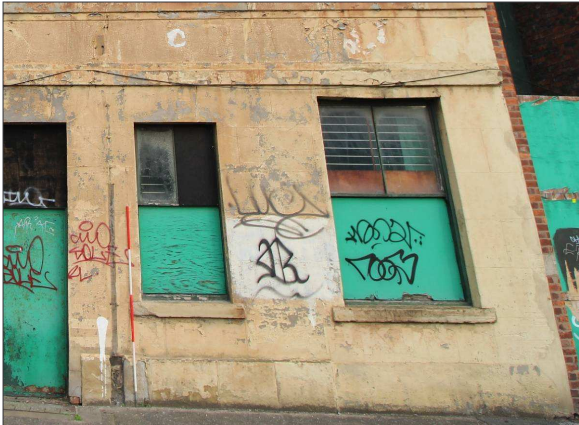
Plate 33: Detail of the ground-floor window apertures
