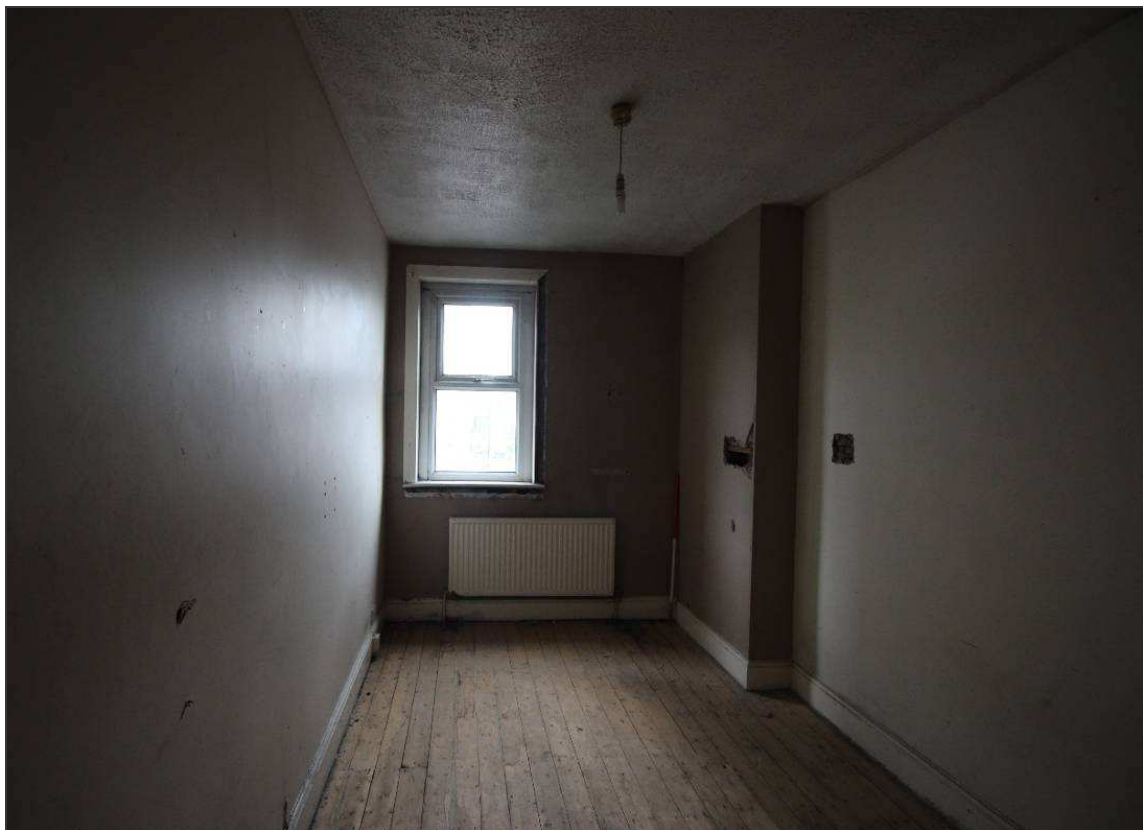
Plate 62: General view of the southern bedroom, detailing the modern window
