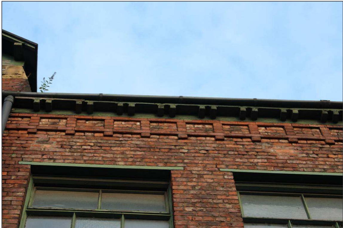
Plate 35: Detail of the string band on the warehouse extension
