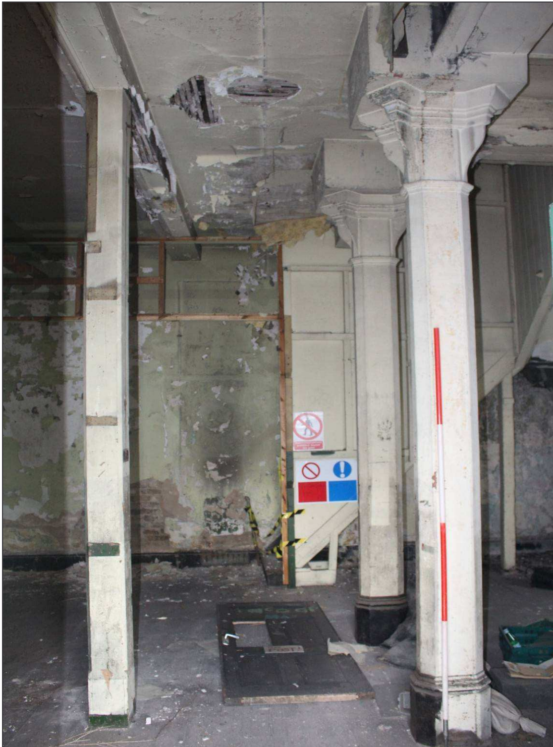
Plate 93: The columns within the centre of the original warehouse
