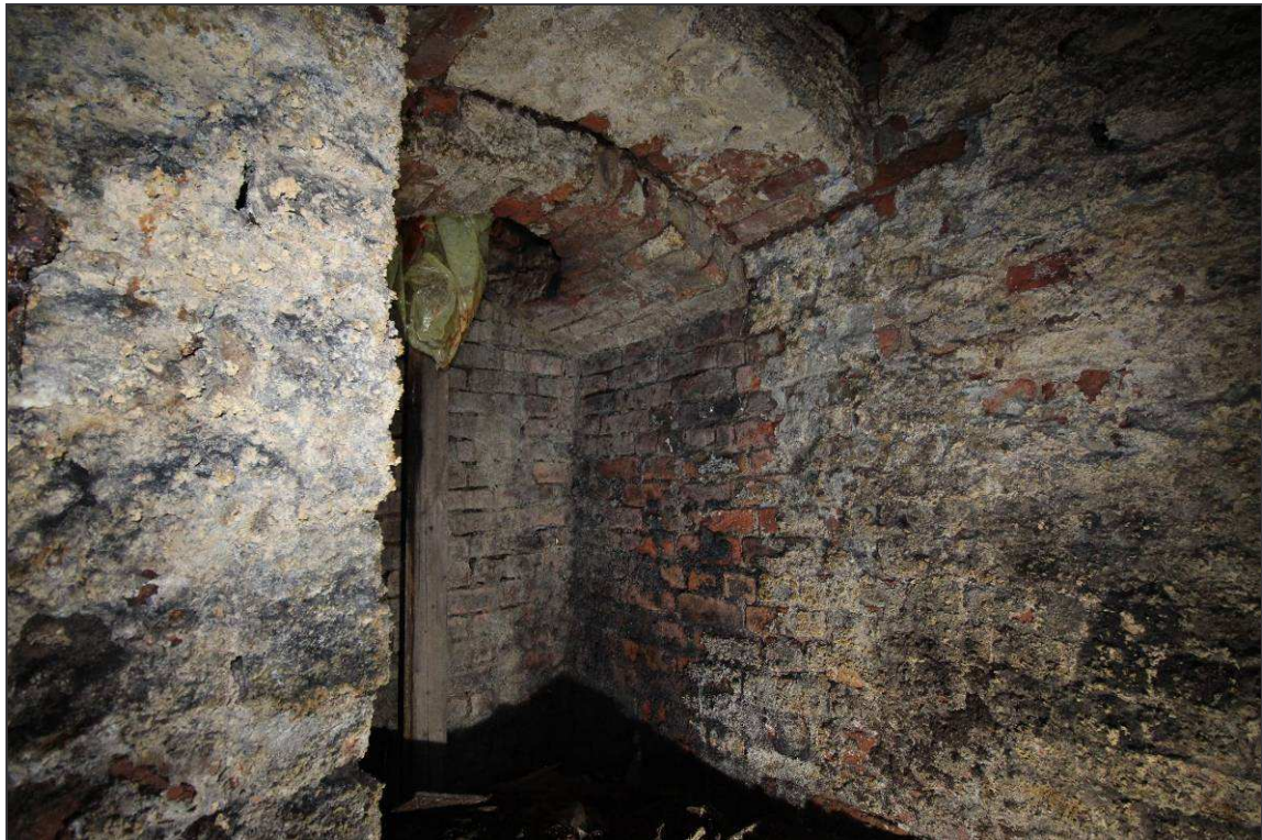
Plate 120: The blocked-up doorway at the eastern end of the room
