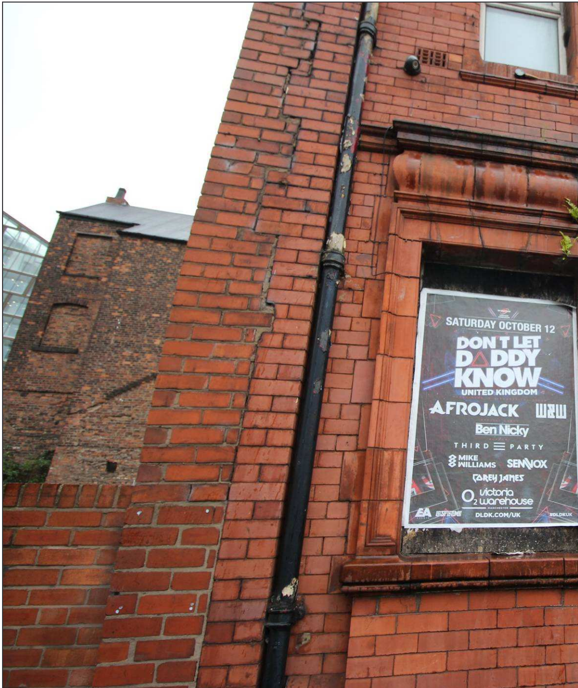
Plate 17: Detail of the keyed joint between the north-west and the north-east wall
