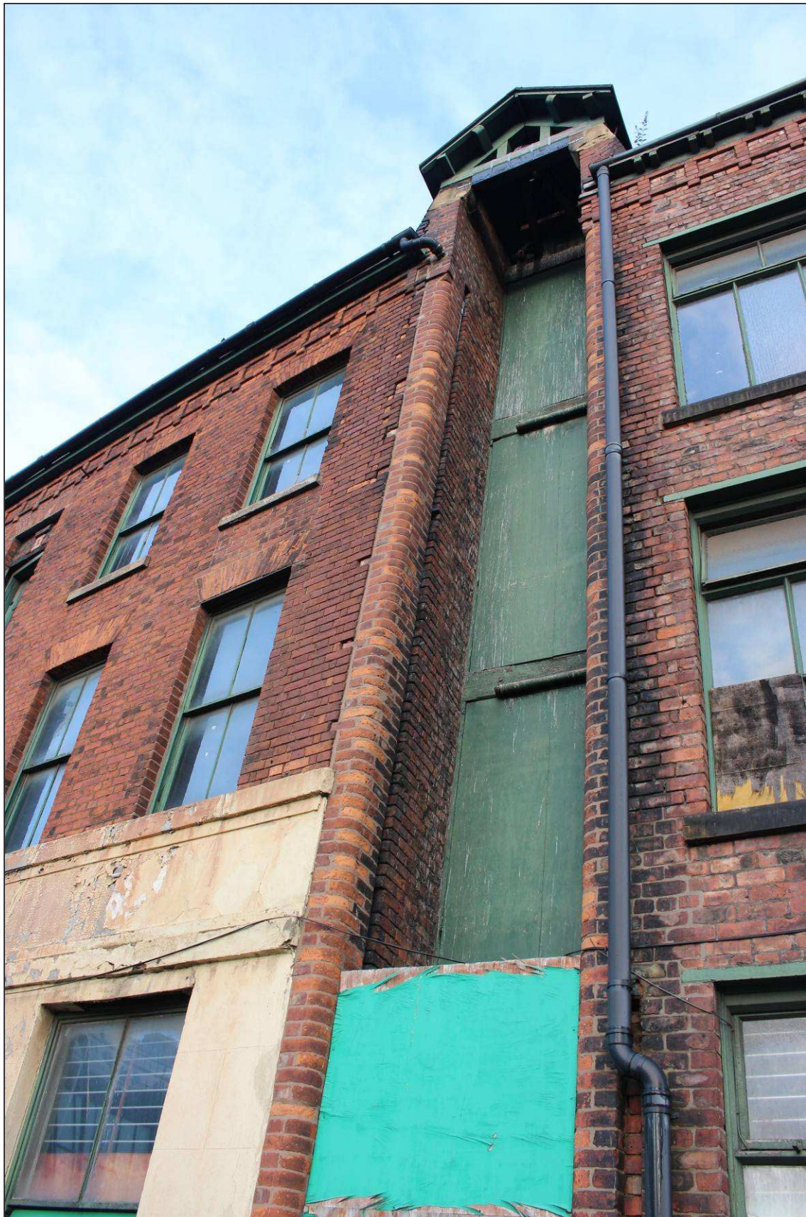
Plate 36: The hoist tower within the centre of the south-eastern façade
