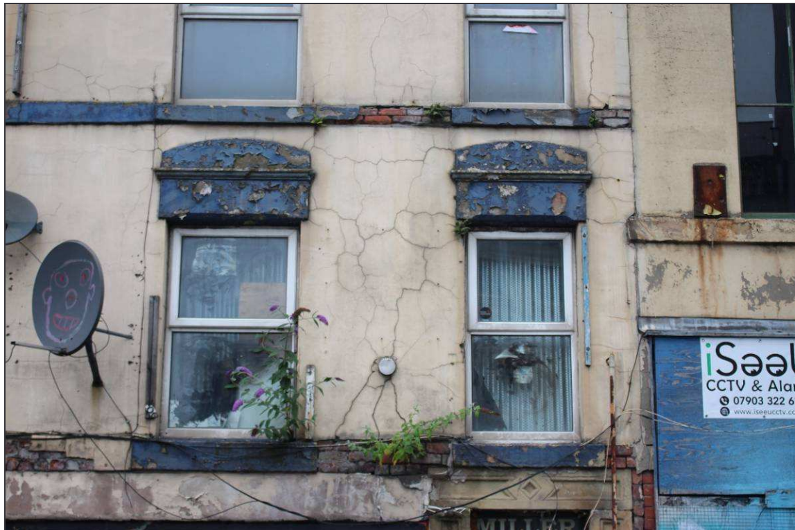
Plate 24: Detail of the first-floor apertures
