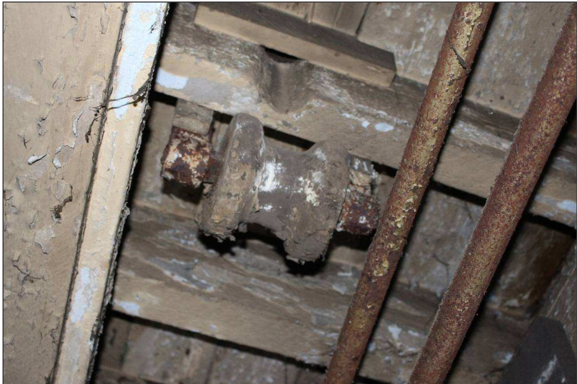
Plate 110: Detail of the pull wheel within the ceiling
