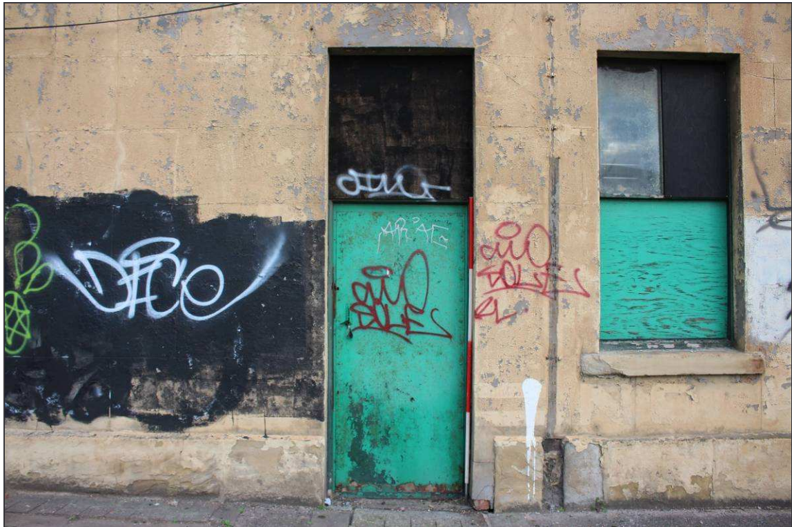
Plate 32: Detail of the doorway into original warehouse on the south-eastern façade
