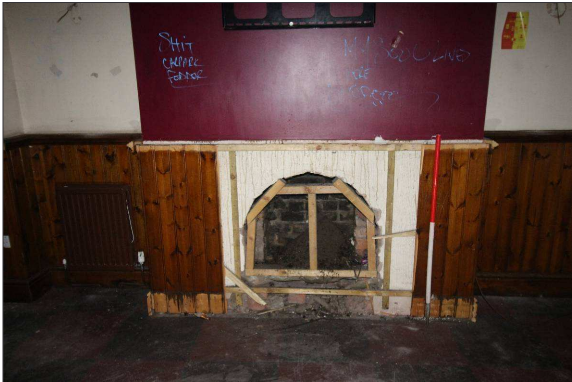
Plate 41: Detail of the blocked-up fireplace within the south-eastern wall
