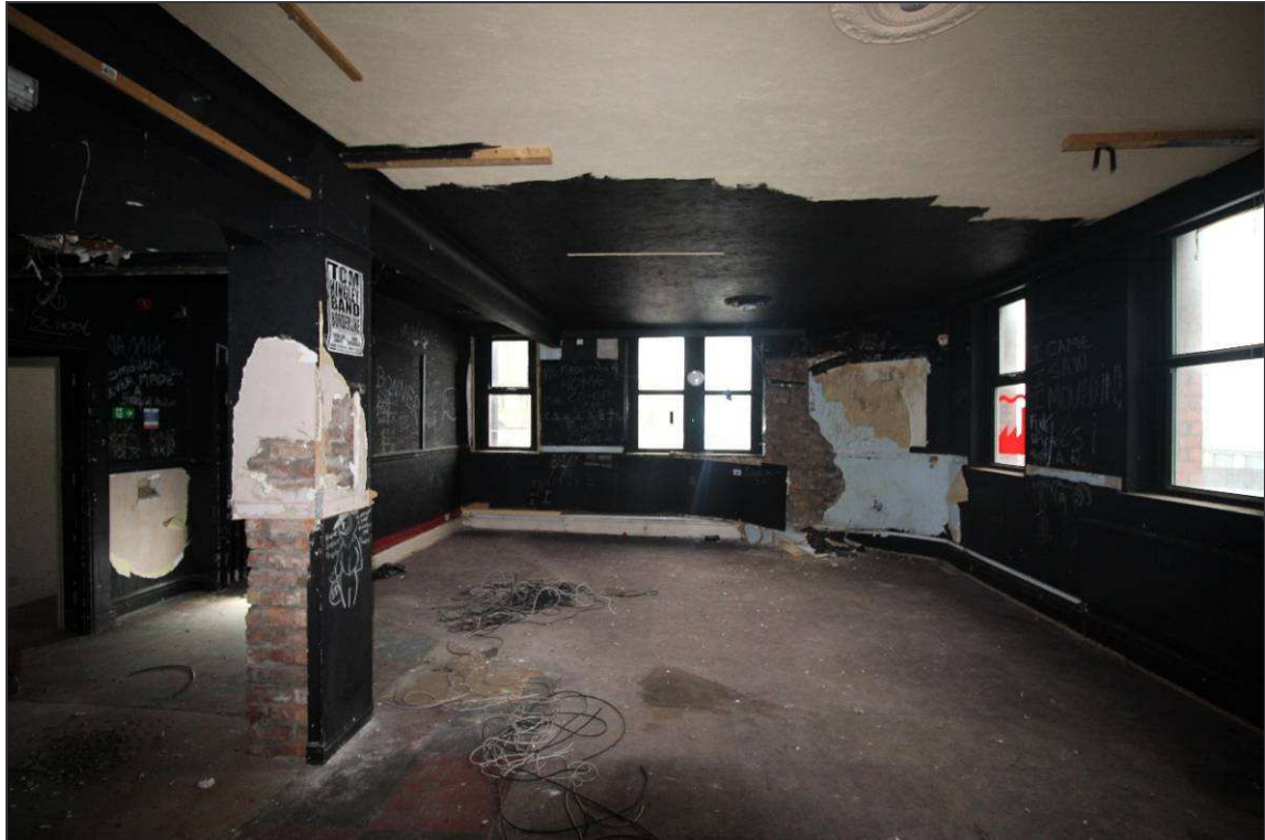
Plate 49: General view of the south-western wall, detailing the window apertures
