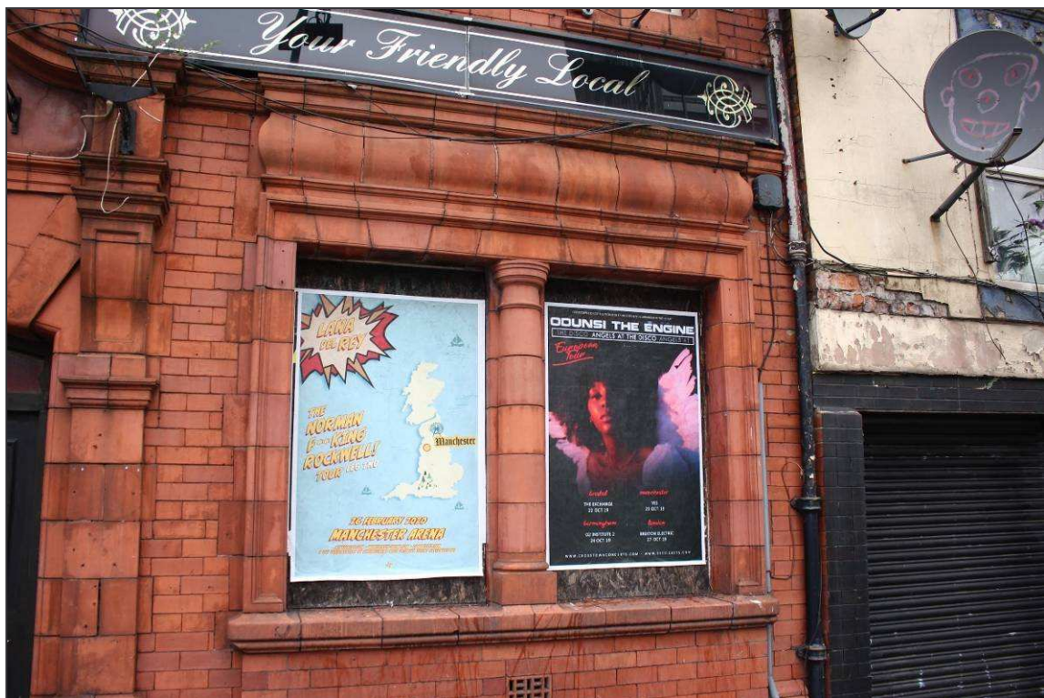
Plate 9: Detailed view of the south-eastern window on the ground floor of the south-western façade
