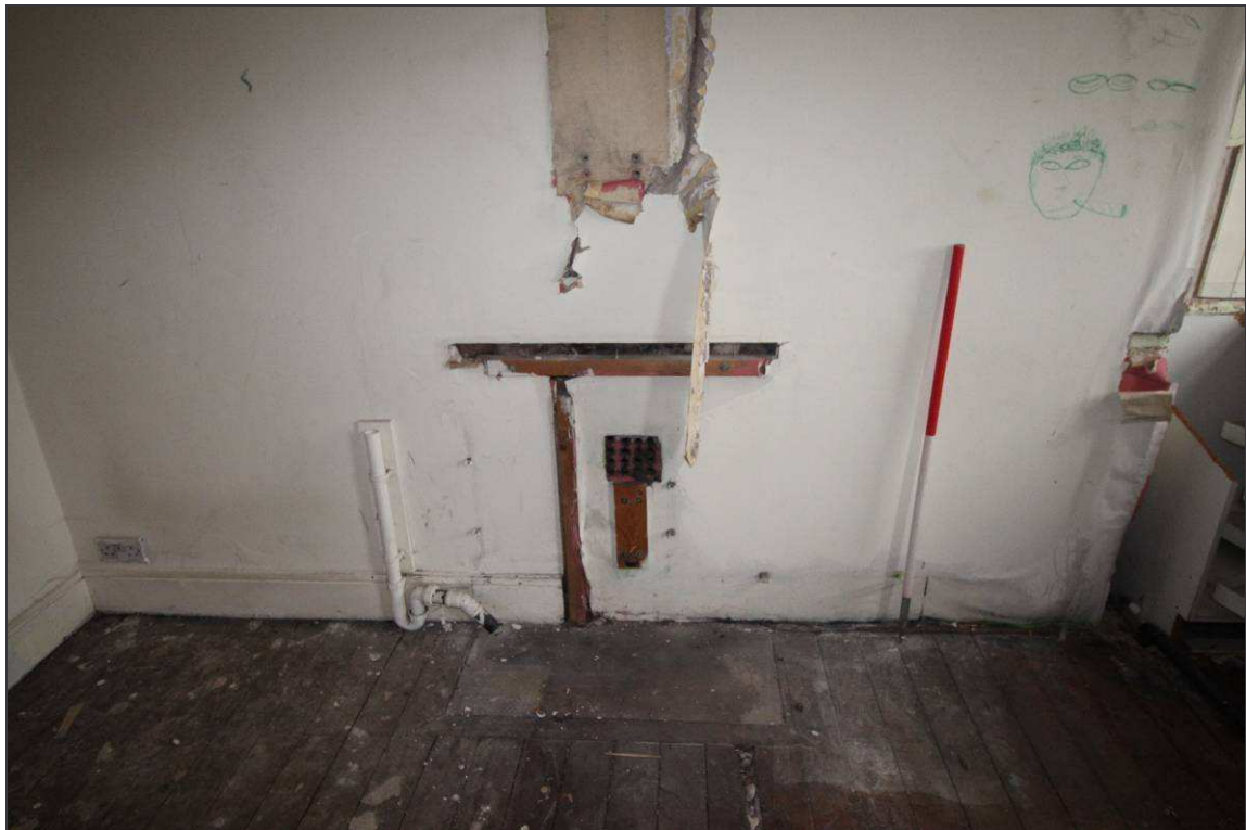
Plate 58: Detail of the blocked-up fireplace within the south-eastern wall
