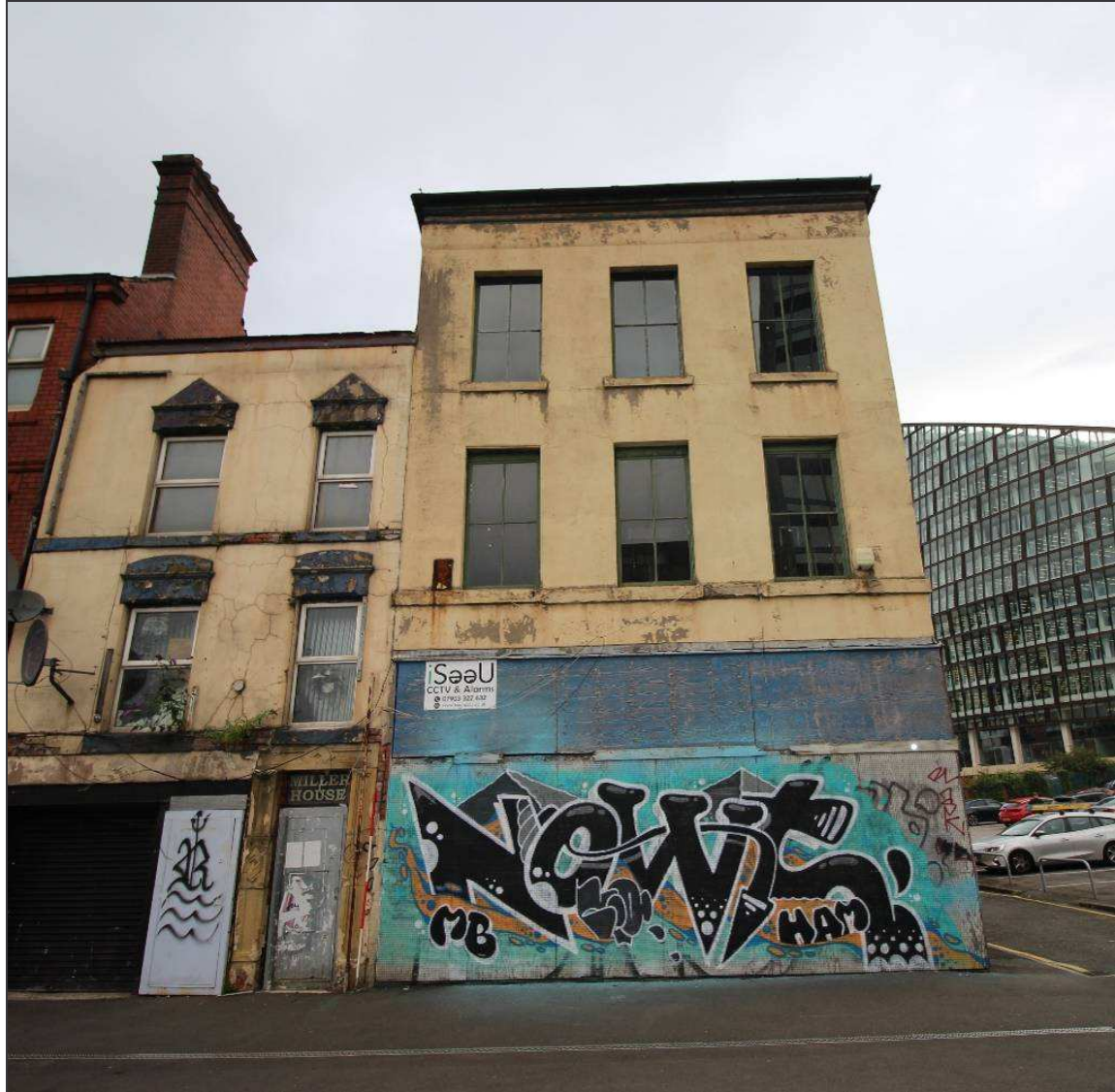
Plate 28: General view of the south-western façade of the warehouse
