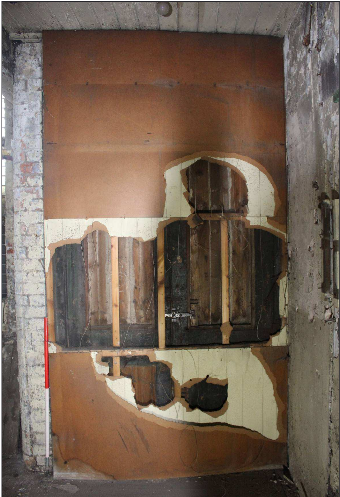
Plate 106: The blocked-up hoist door
