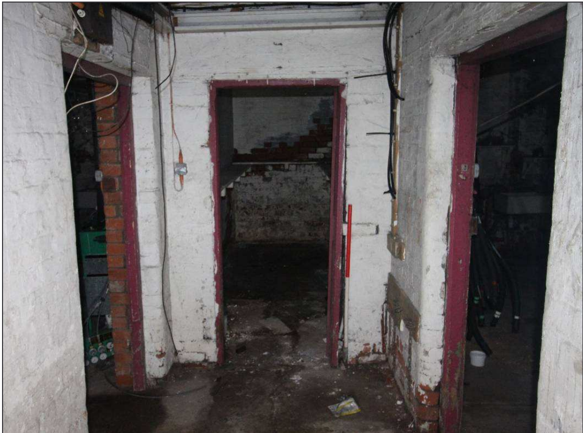
Plate 73: Detail of the doorway leading into the north-western room
