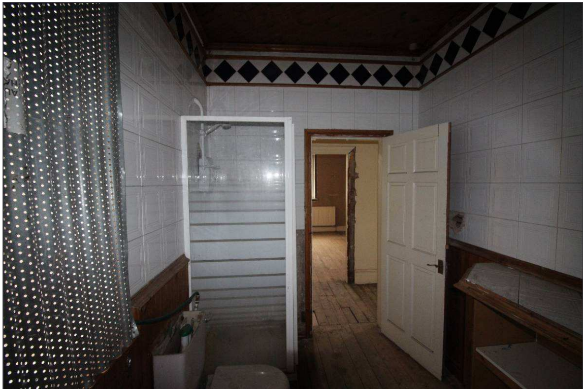
Plate 61: The south-west wall of the bathroom, detailing the doorway at the north-western end
