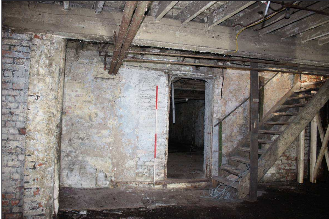
Plate 112: The south-western wall of the central room, detailing the central doorway
