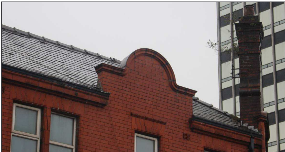
Plate 16: Detail of the central parapet wall
