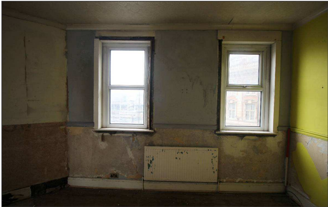
Plate 64: Detail of the window apertures within the north-western wall
