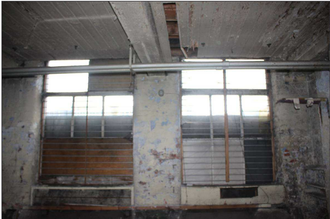
Plate 102: Detail of the recessed window apertures within the south-east wall
