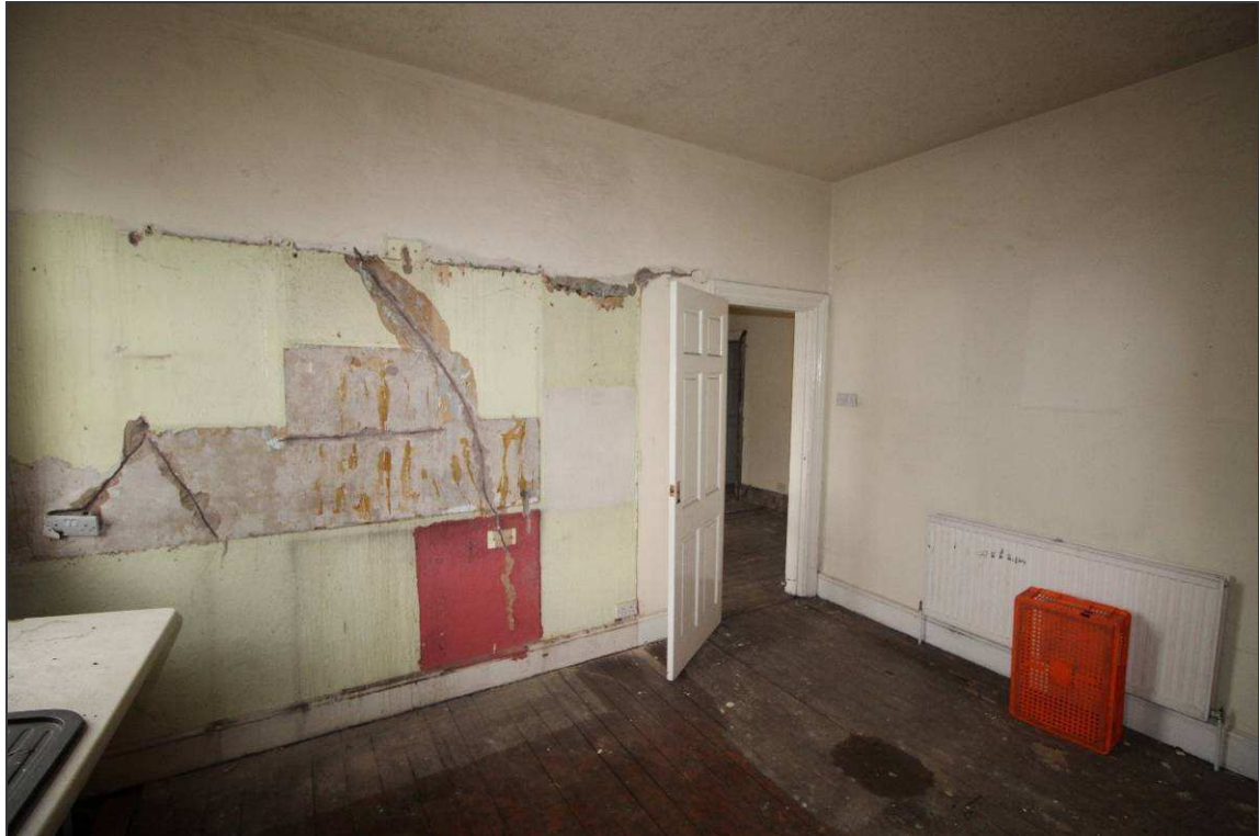
Plate 57: General view of the north-western wall, detailing the doorway into the kitchen
