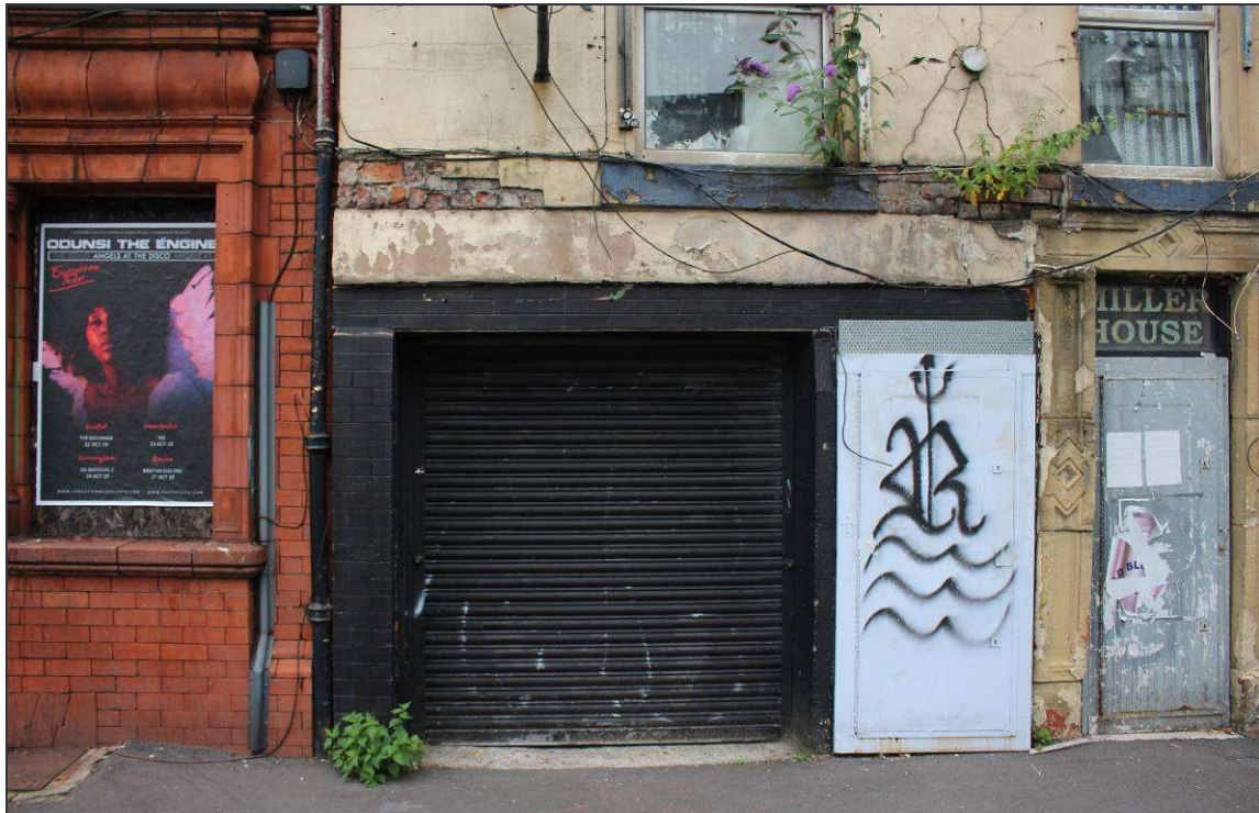
Plate 22: The shop front on the ground floor of the south-western façade
