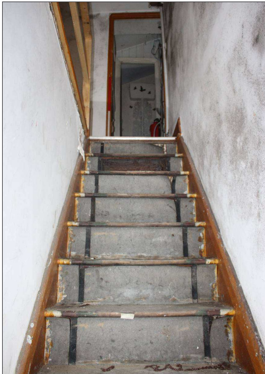
Plate 85: The timber staircase leading to the second-floor
