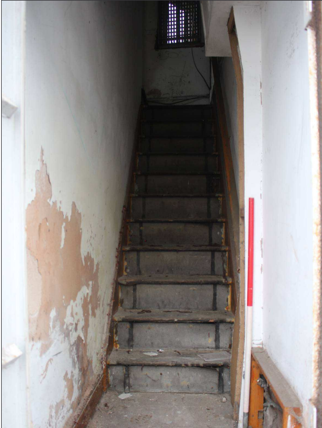
Plate 82: The timber staircase leading to the first floor
