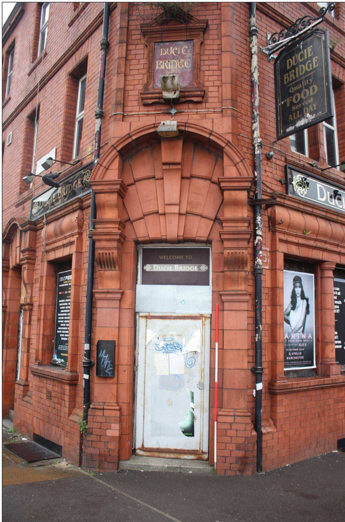
Plate 18: Detail of the doorway within the western façade
