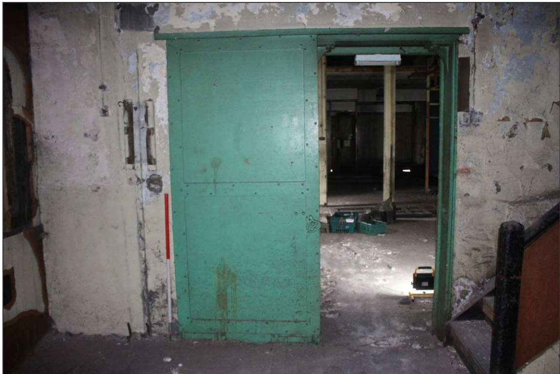
Plate 100: Detail of the riveted door within the north-eastern doorway
