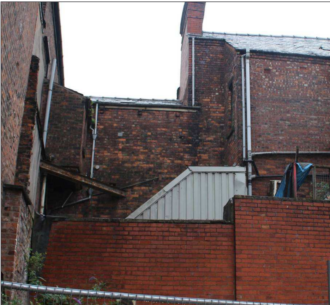
Plate 26: The north-east façade of the office building
