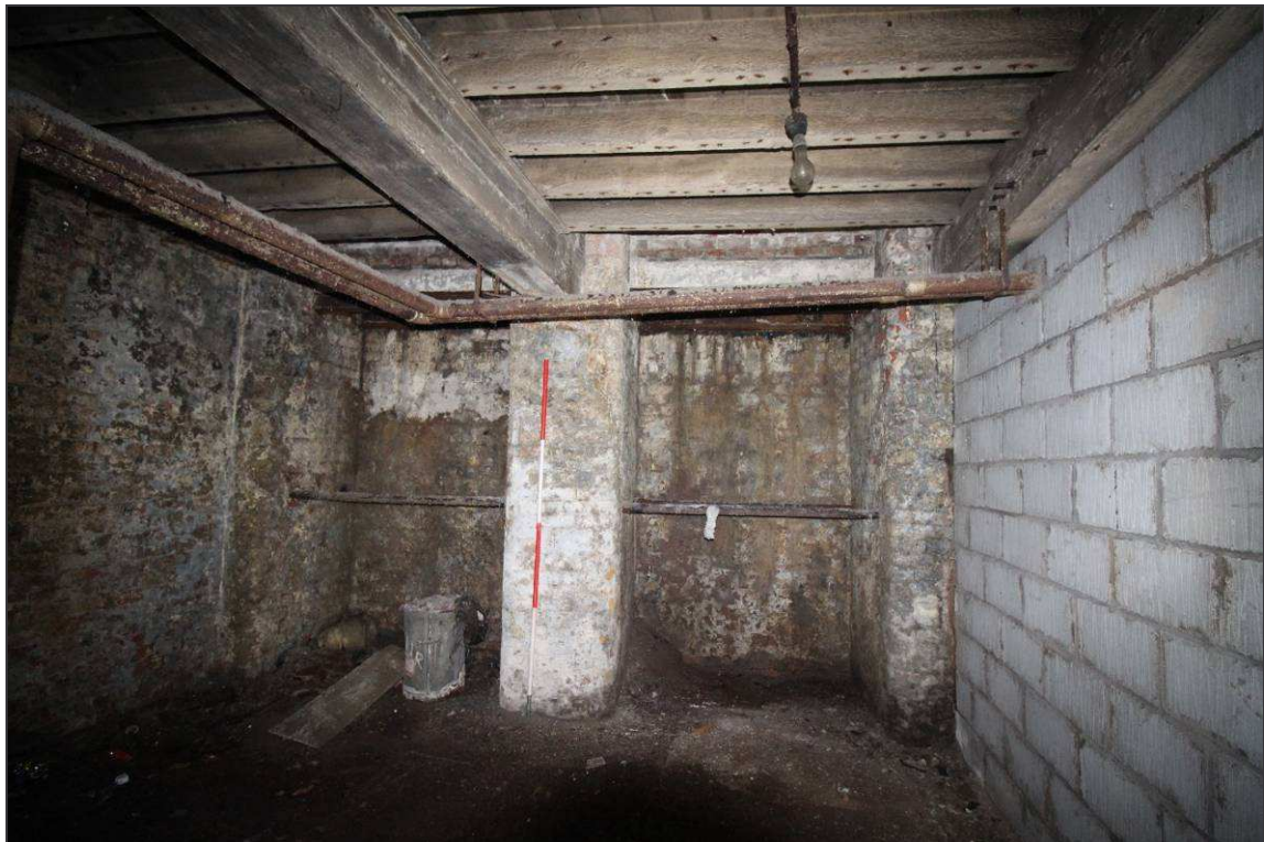
Plate 113: General view of the north-eastern room within the basement
