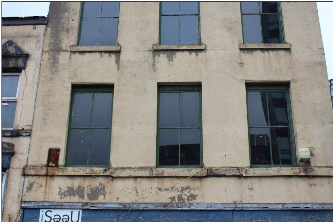
Plate 29: Detail of the first-floor window apertures on the south-western façade
