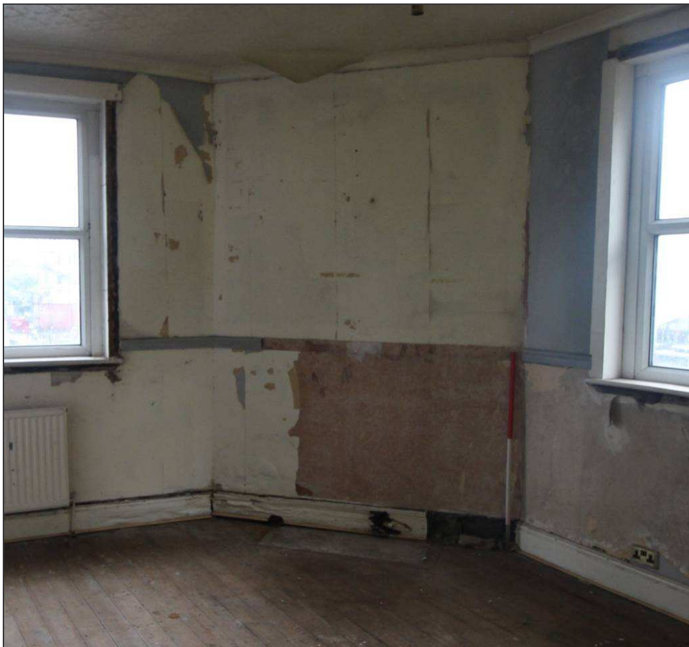
Plate 65: Detail of the blocked-up fireplace within the western wall
