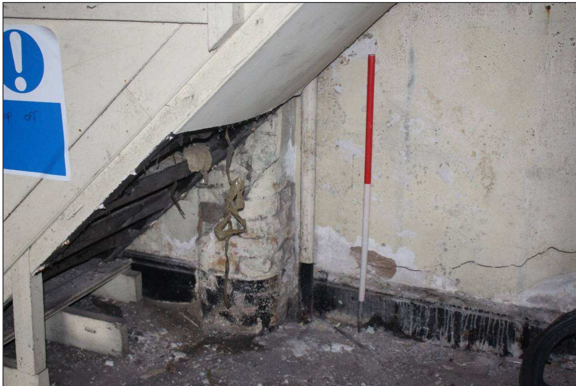
Plate 97: Detail of the possible position of an earlier staircase leading up into the first-floor of the warehouse
