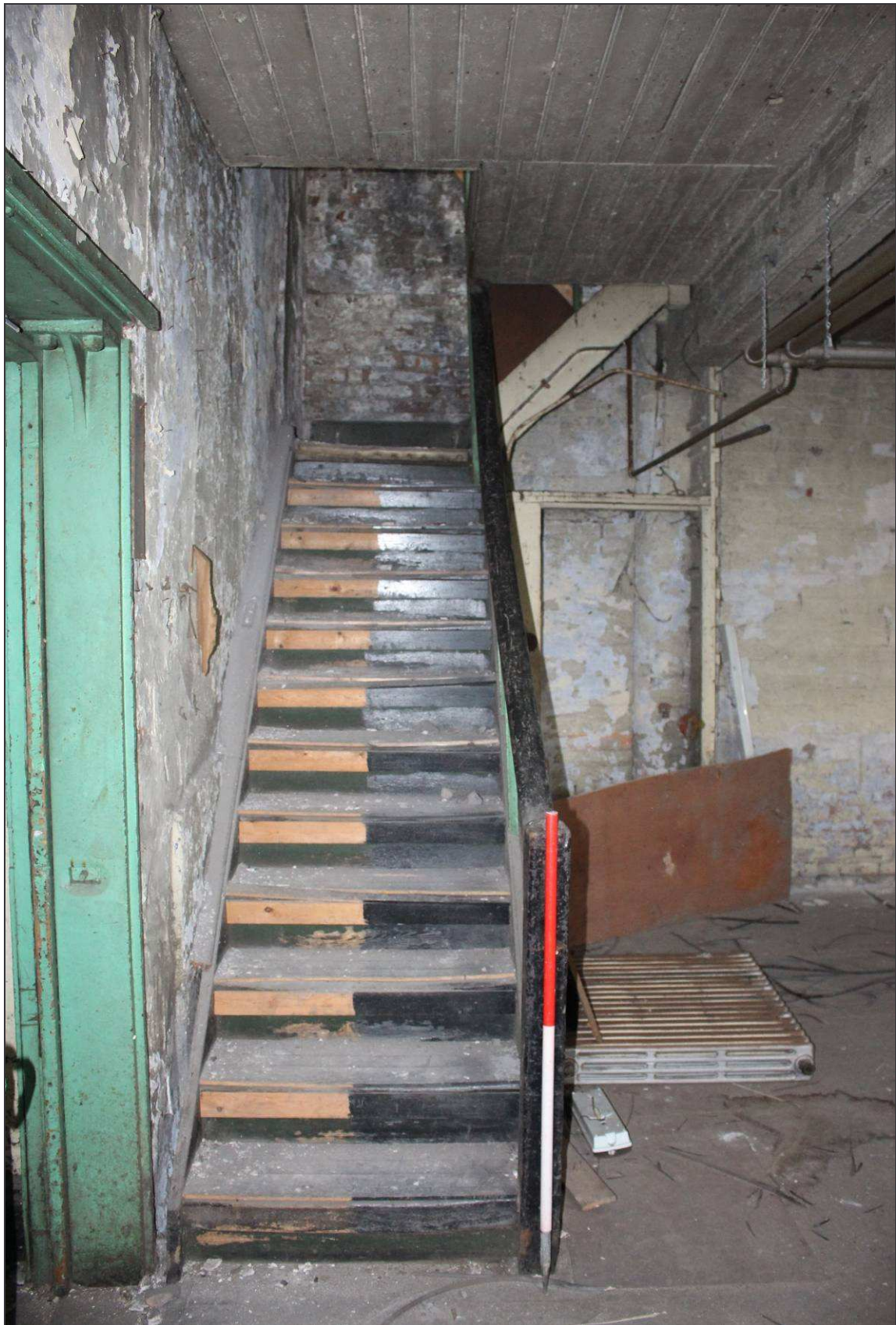
Plate 105: The timber staircase leading to the first-floor of the extension
