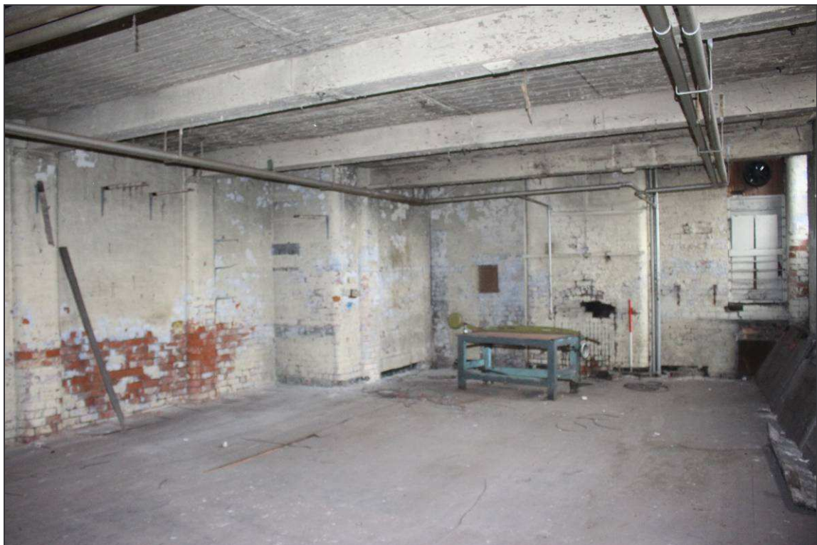
Plate 101: General view of the later extension to the warehouse
