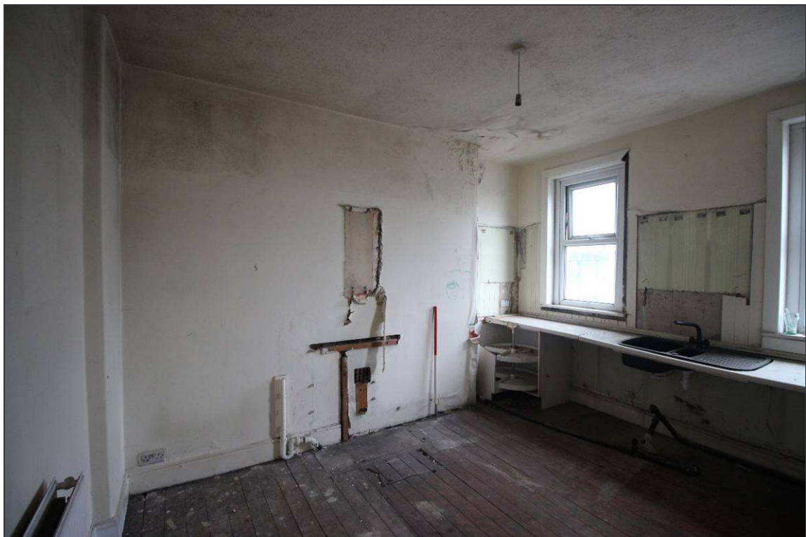
Plate 56: The kitchen at the south-west corner of the second-floor
