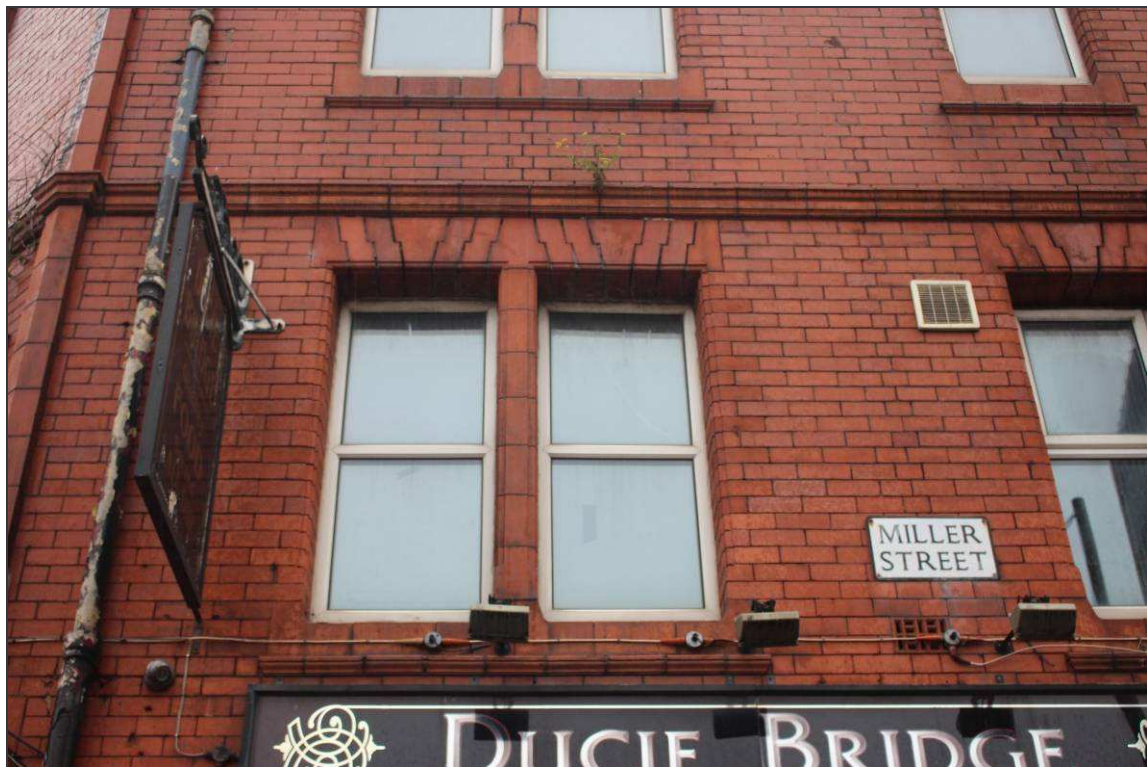
Plate 10: Detail of the first-floor window apertures
