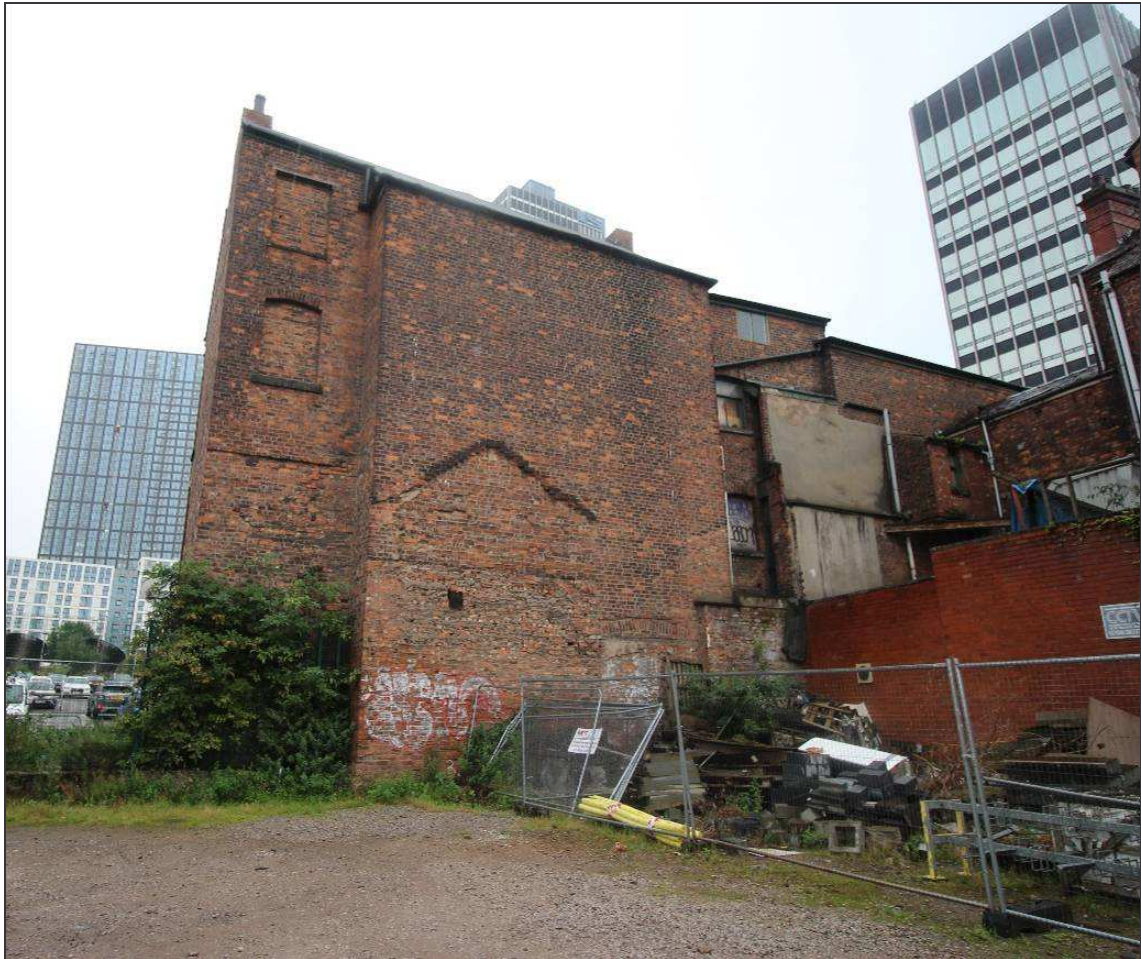
Plate 39: General view of the north-western façade of the warehouse
