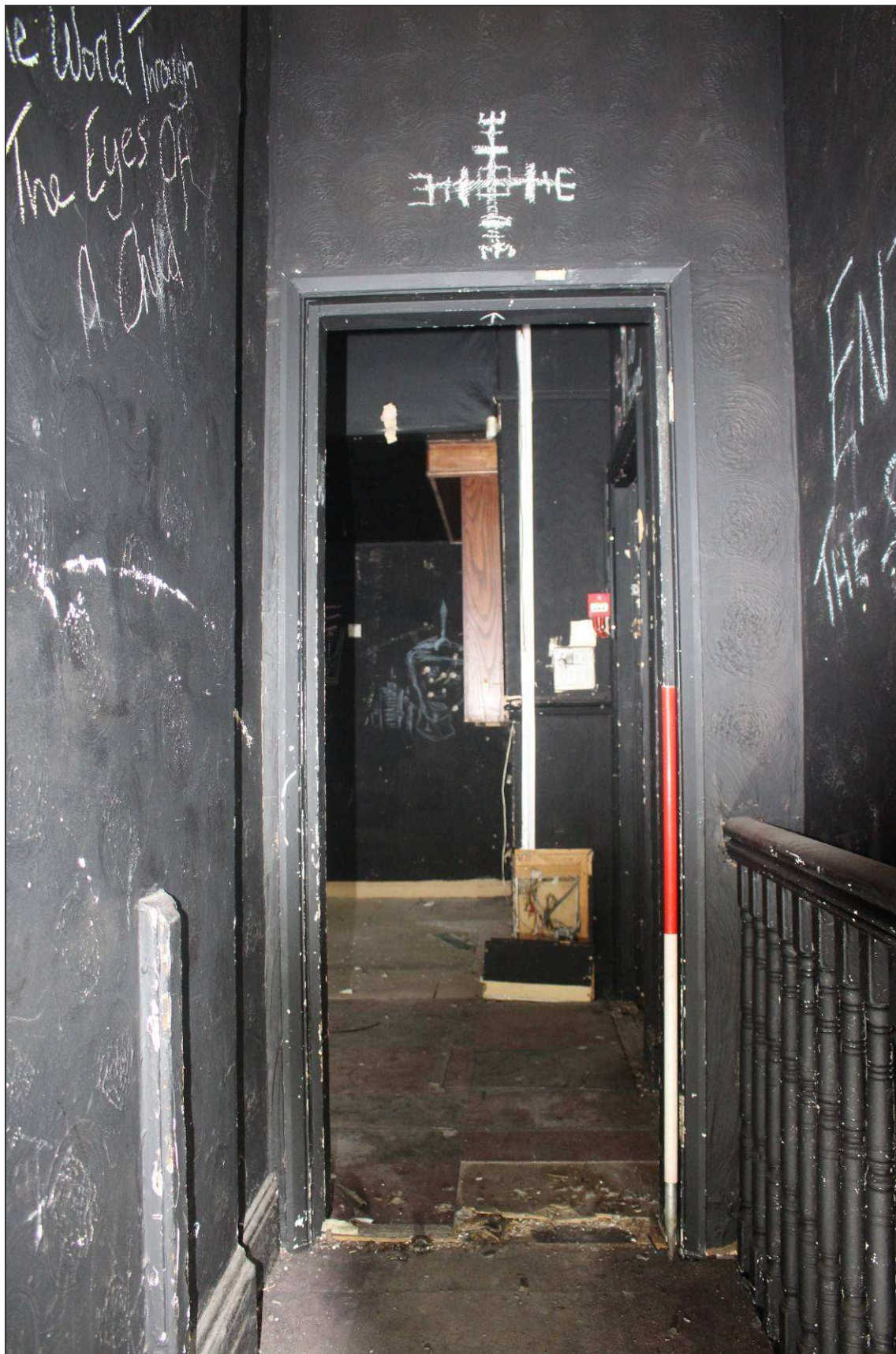
Plate 46: Detail of doorway leading into the first floor of the public house
