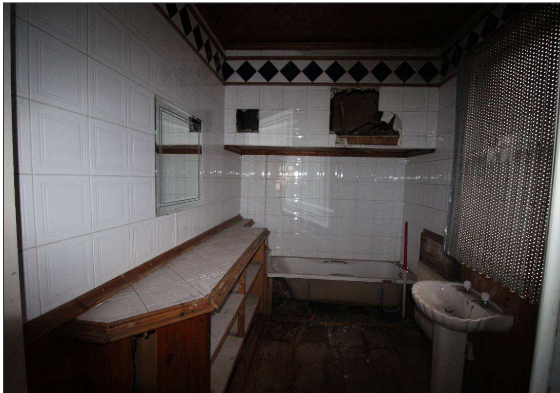
Plate 60: The modern bathroom the second floor
