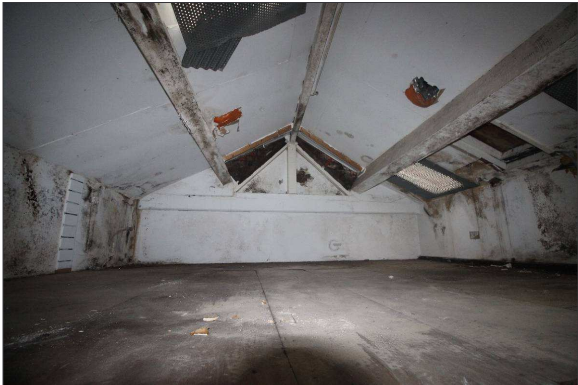
Plate 90: General view of the roof space
