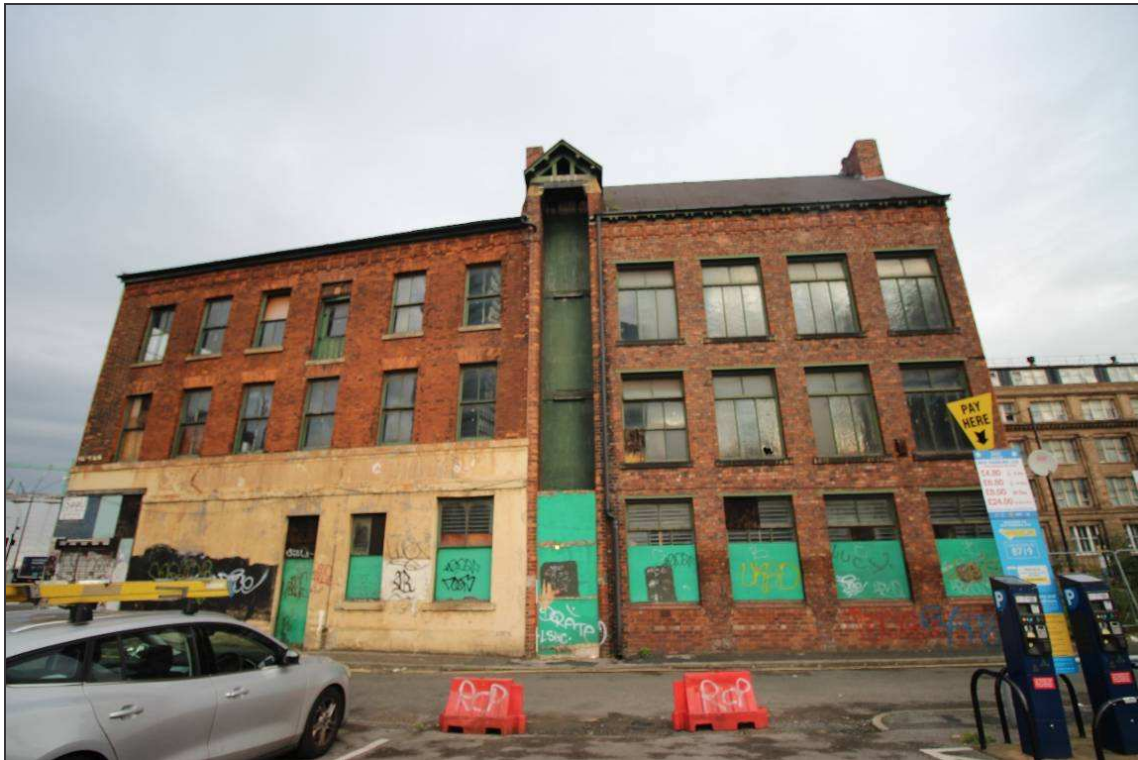
Plate 30: General view of the south-eastern façade of the warehouse
