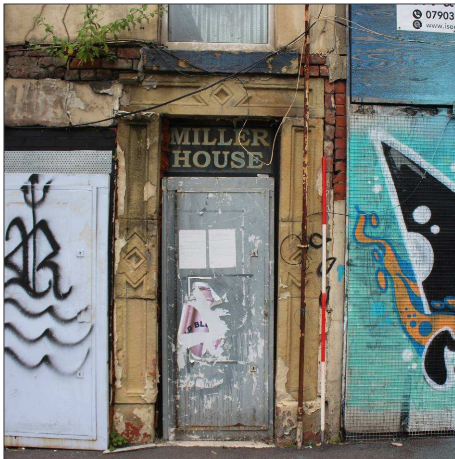
Plate 23: Detail of the south-eastern doorway
