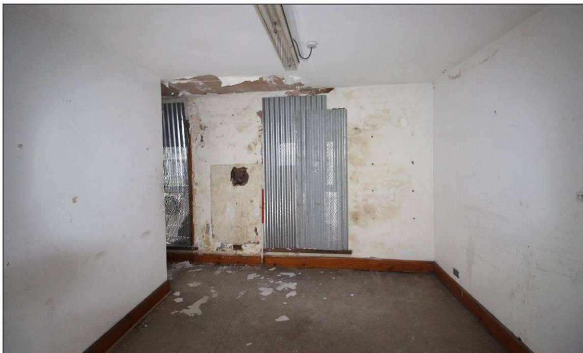
Plate 84: Detail of the blocked-up window within the first-floor room
