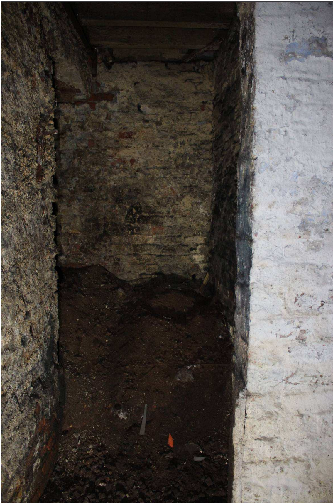
Plate 119: The narrow corridor leading to the blocked-up doorway
