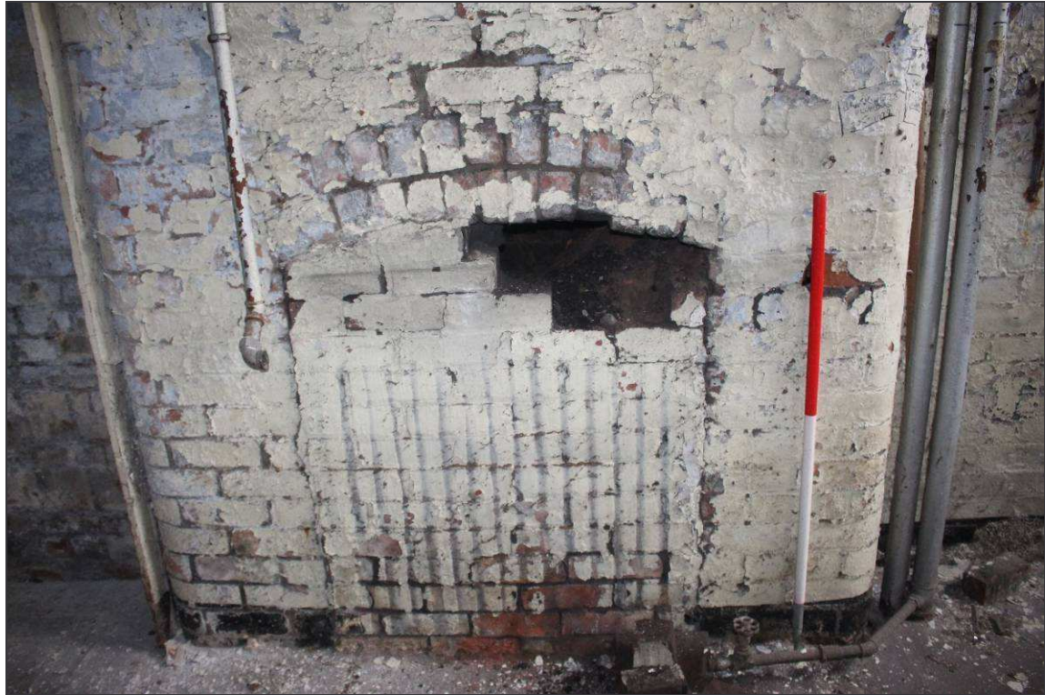
Plate 104: The blocked-up fire-place in the north-east wall
