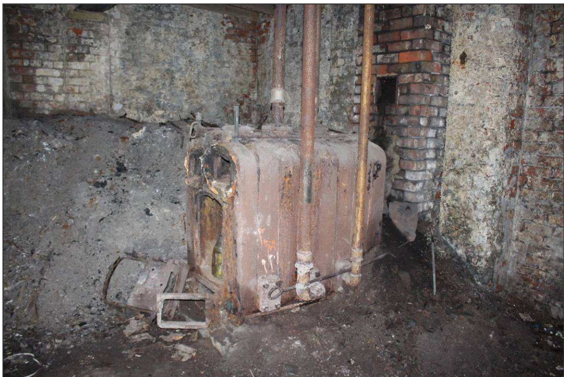
Plate 114: The later boiler within the north-eastern room
