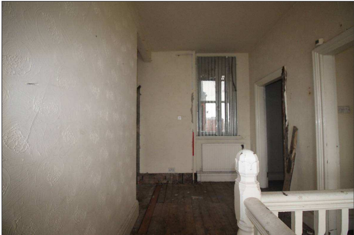
Plate 55: General view of the second-floor landing detailing the single window within the north-eastern wall
