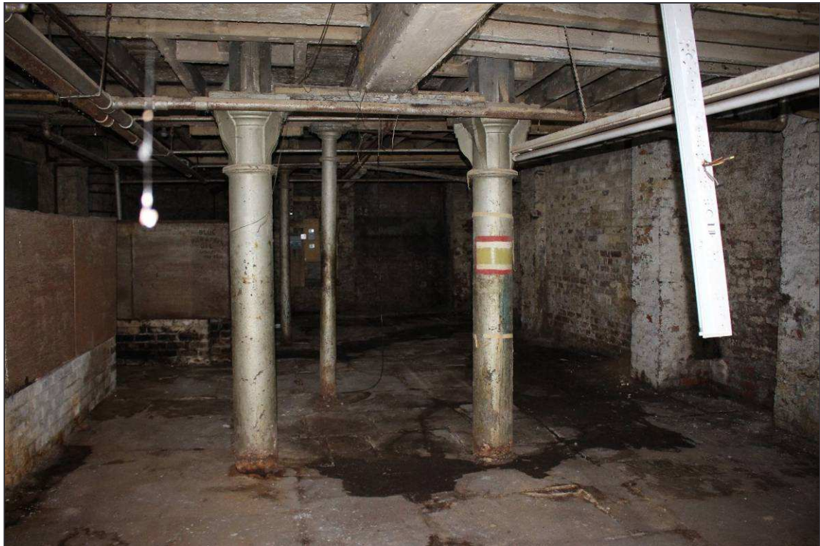
Plate 116: General view of the south-western room of the basement
