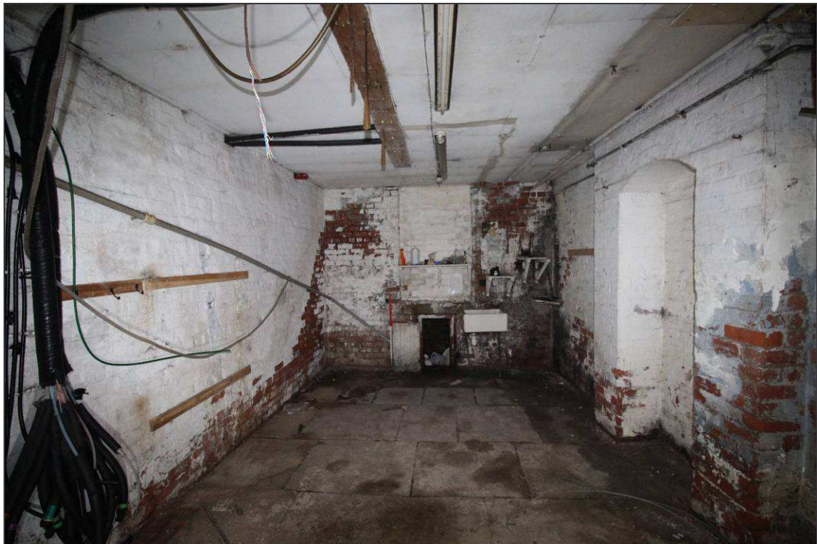
Plate 80: The north-eastern room of the basement
