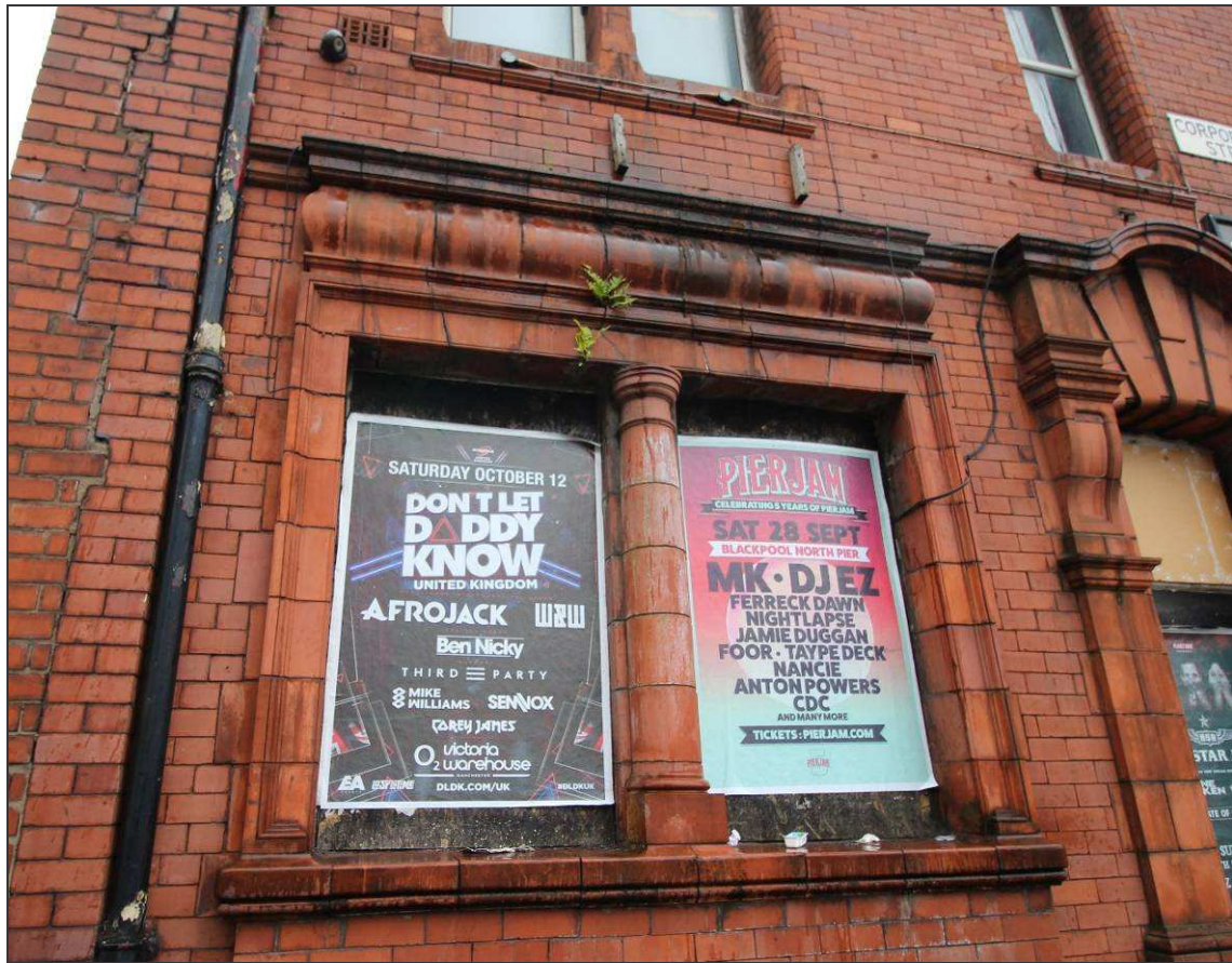
Plate 14: Detail of the north-west window on the south-western façade
