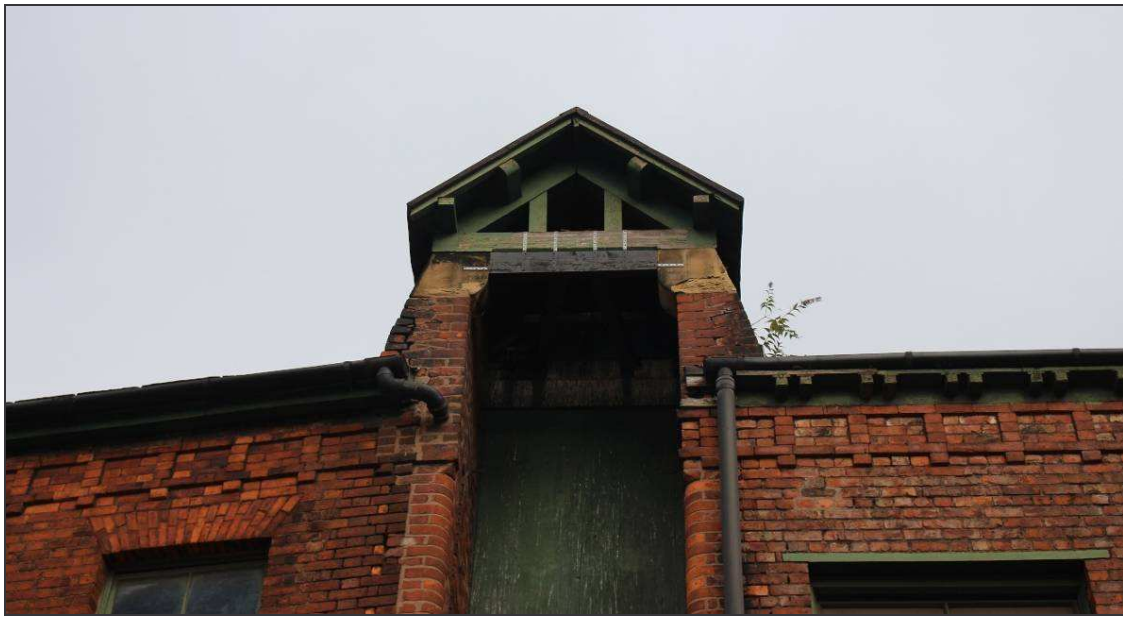
Plate 37: Detail of the timber truss of the hoist tower
