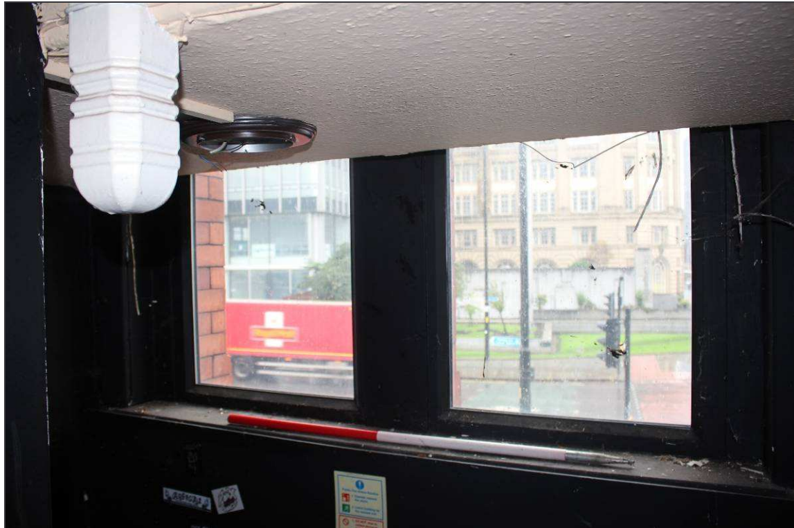
Plate 45: Detail of window apertures on the first-floor landing of the central staircase
