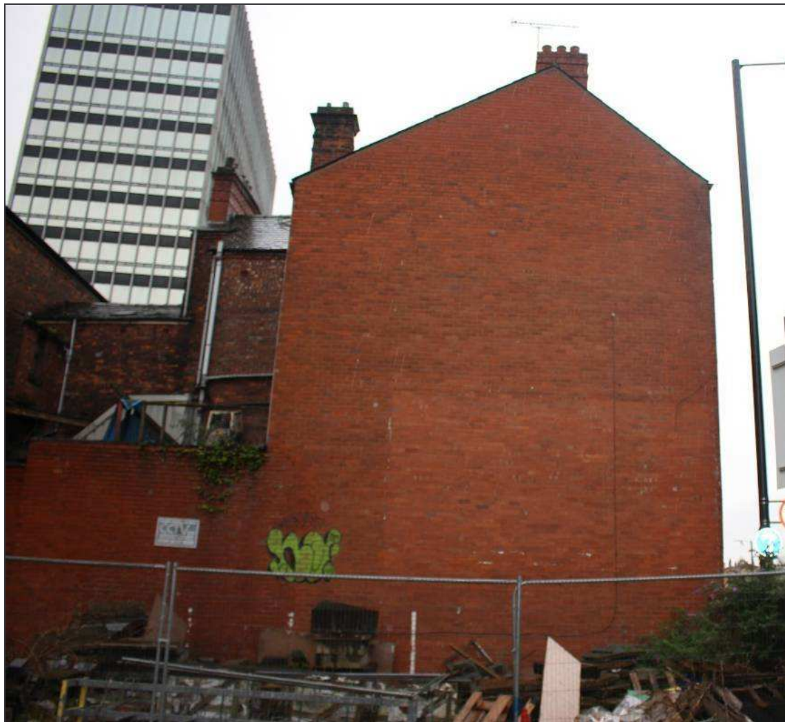
Plate 19: The rebuilt north-eastern façade
