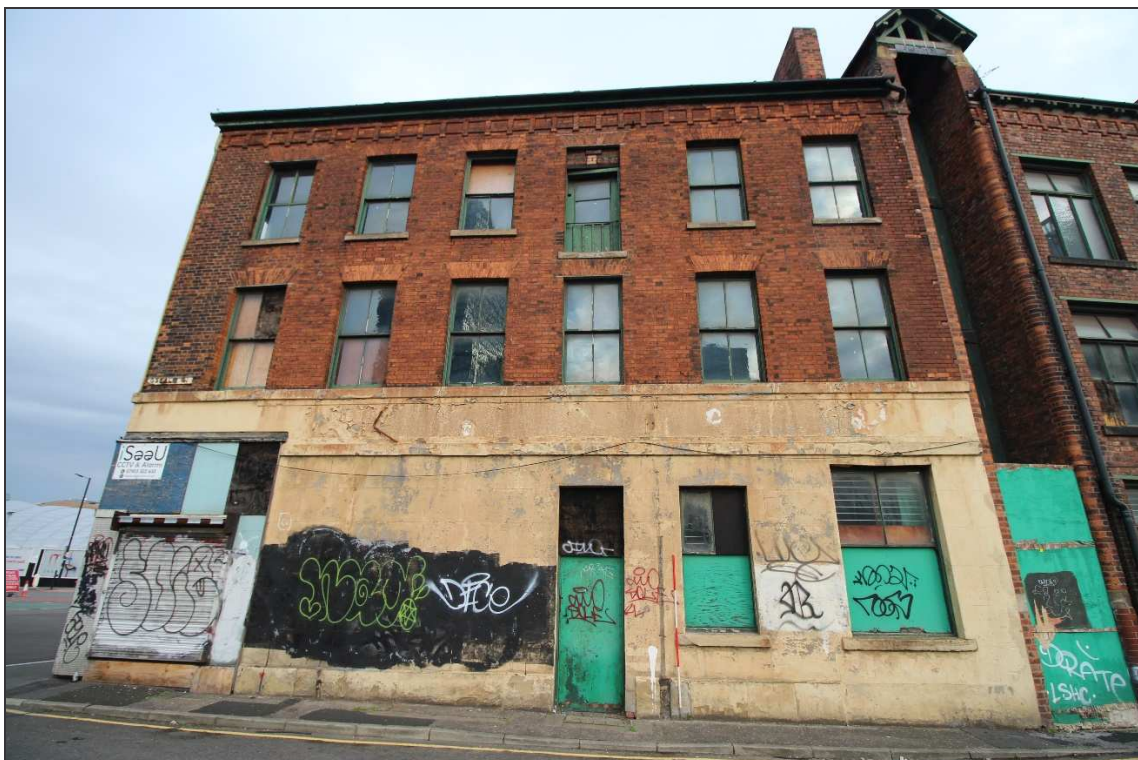
Plate 31: General view of the original warehouse façade
