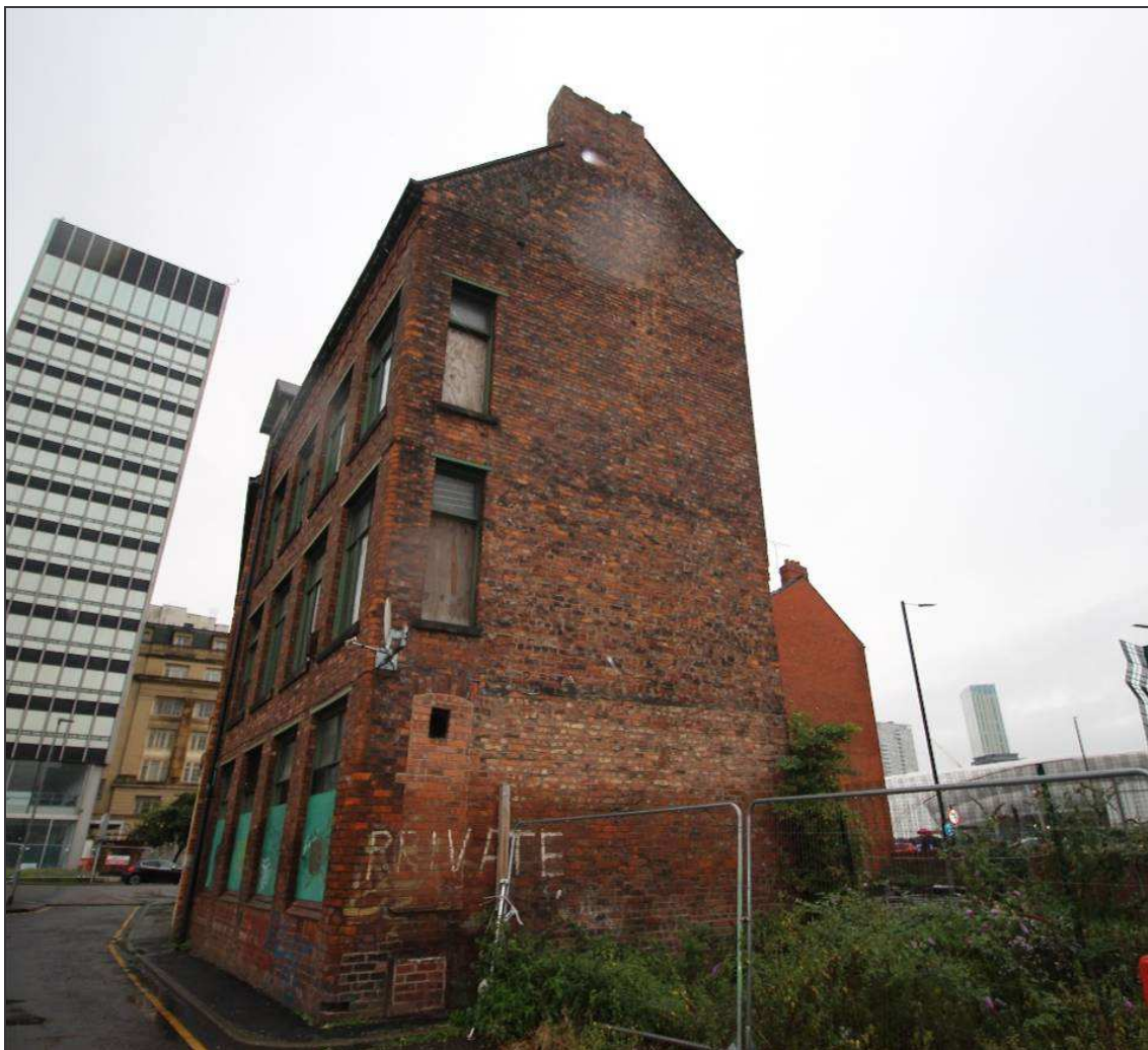
Plate 38: General view of the north-eastern façade of the warehouse
