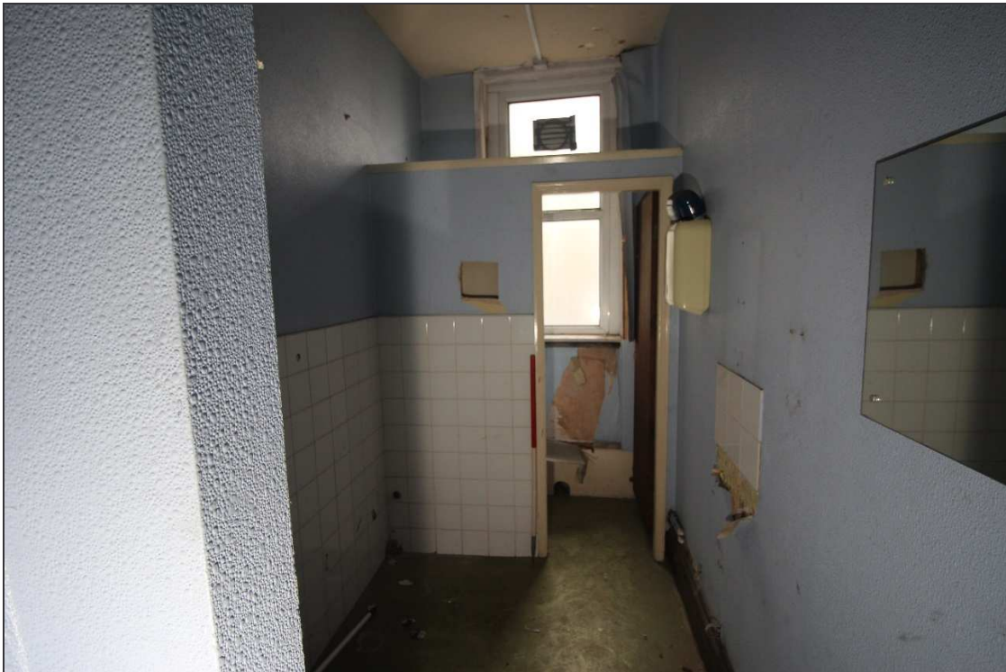
Plate 52: General view of the gent's toilets on the first-floor
