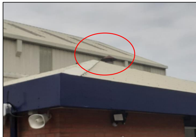
Figure 9: View of existing extract ductwork / termination cowl to be reused
