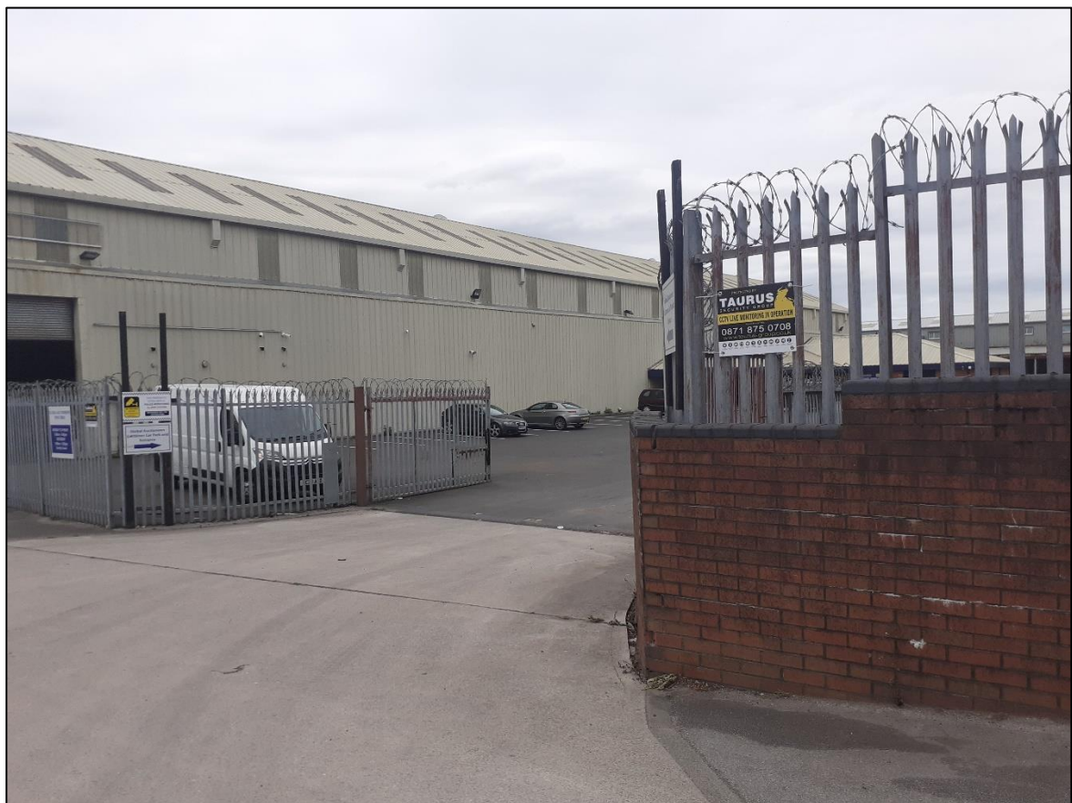
Figure 5: View of the site access. The loading bay in the south west corner of the building is also visible.
