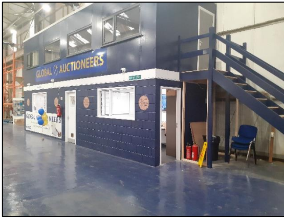
Figure 3: View of the interior of the north building.
