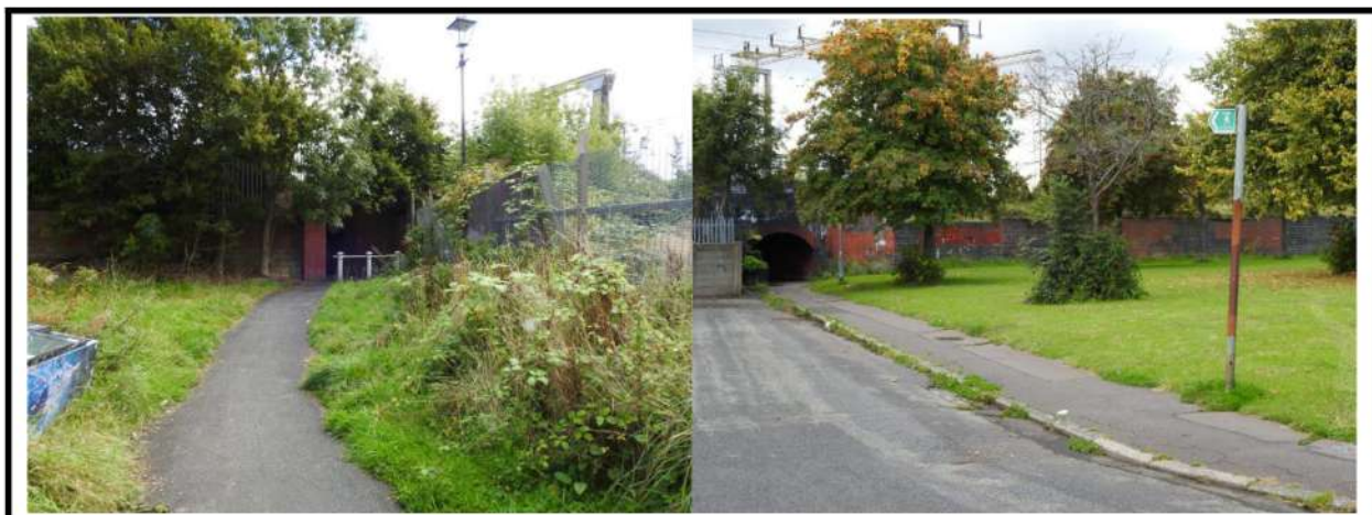
Footpath to west under rail line
