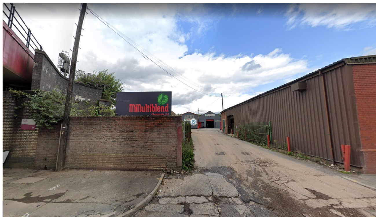
Photo 1 - Showing masonry wall and access to industrial compound
