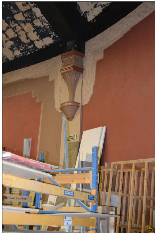
Photograph 32: Detailed view of one of the pilasters and wall details.
