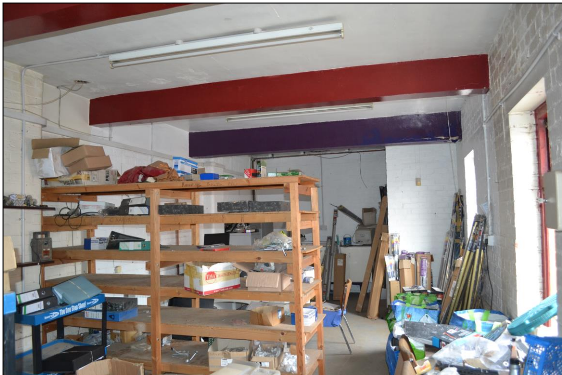
Photograph 30: View west across the storage room on the second floor.
