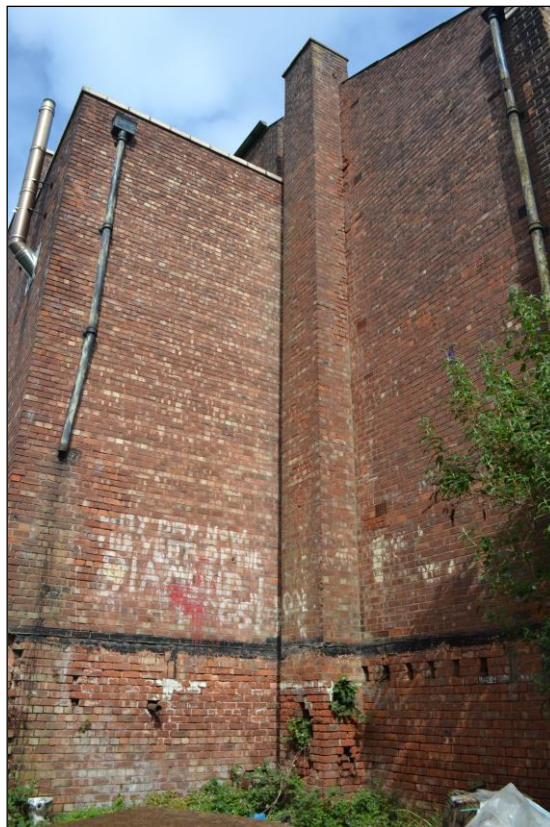
Photograph 12: Detailed view of the chimney attached to the southern elevation.
