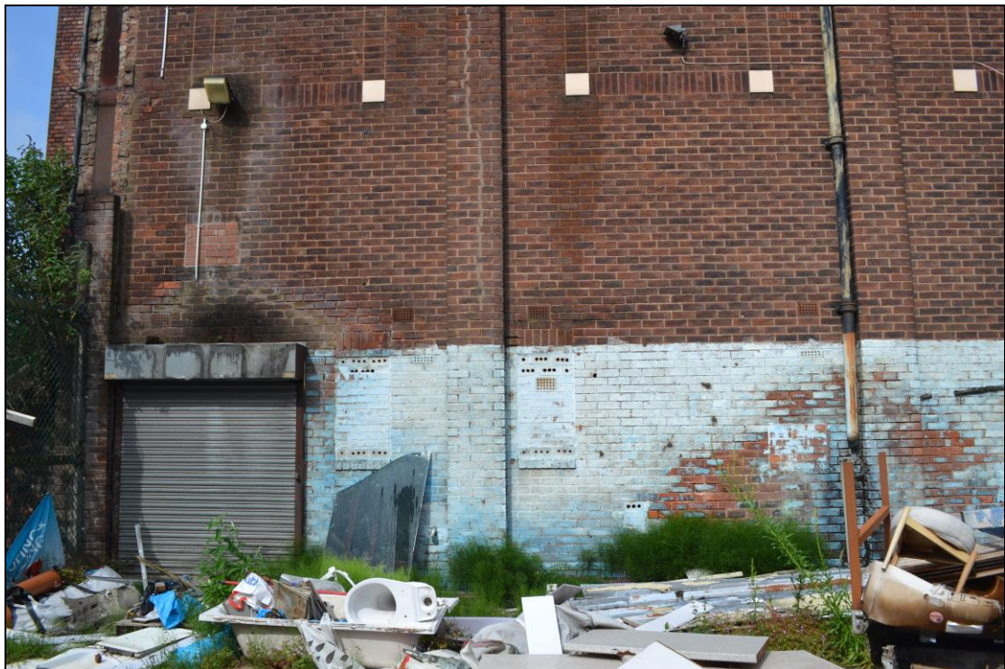
Photograph 10: View west of the southern part of the eastern elevation.
