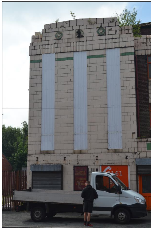
Photograph 4: View of the eastern wing of the northern façade.
