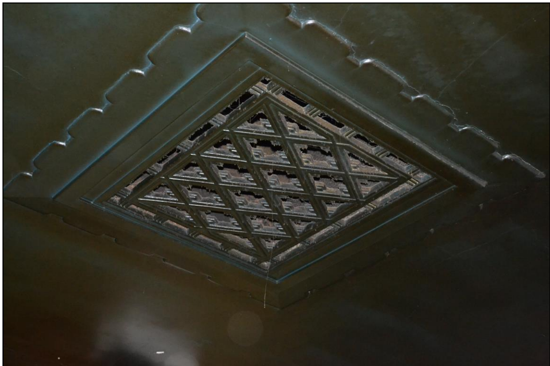
Photograph 36: Detail of one of the iron grates set into the ceiling.
