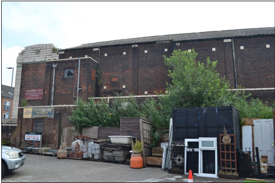
Photograph 13: View east of the northern part of the western elevation.
