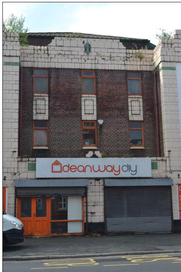
Photograph 2: View south of the central part of the northern façade.
