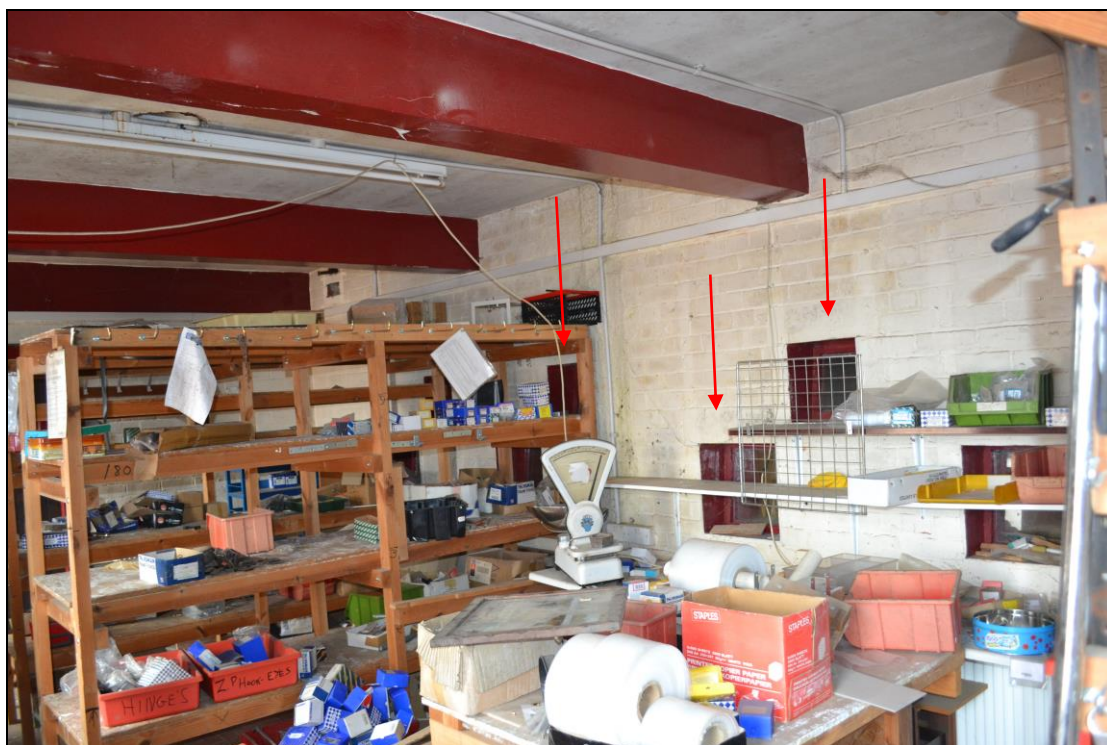
Photograph 26: View south-east across the former projection room. Note the windows built into the southern wall (red arrow).
