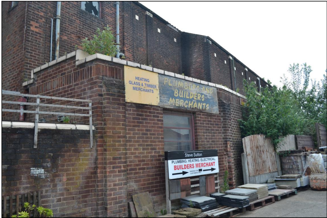
Photograph 15: View south of the extension along the eastern elevation.
