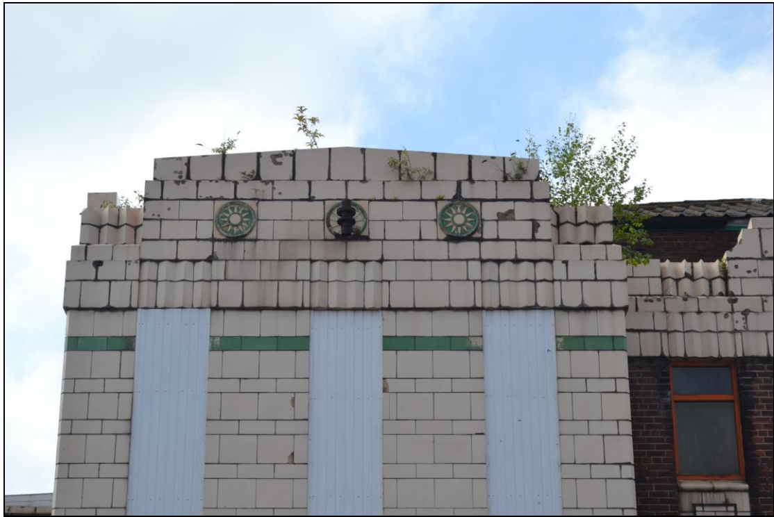
Photograph 5: Detailed view of the roofline detail of the eastern wing of the northern façade
