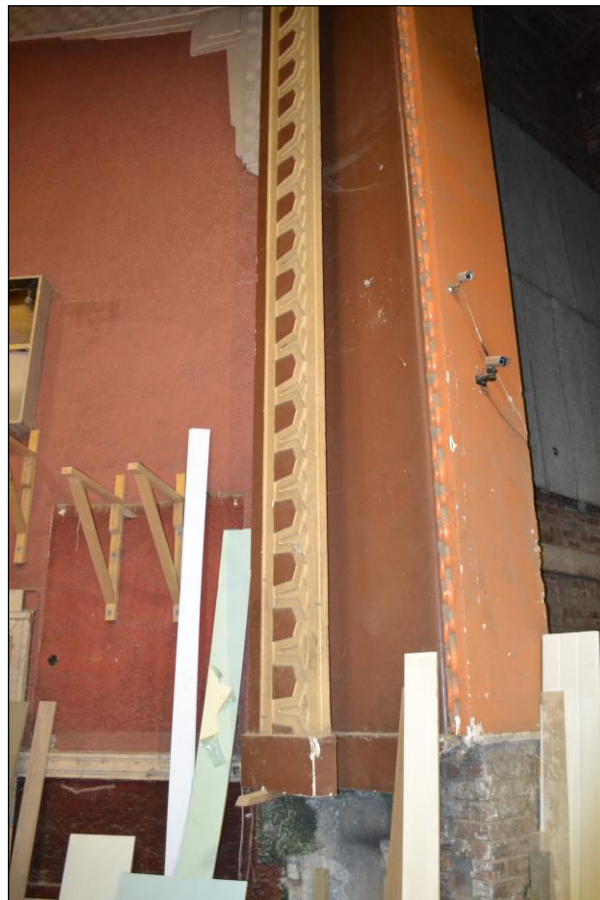
Photograph 40: View of the detail around the proscenium arch.
