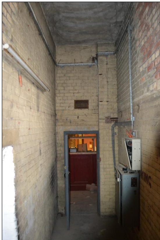
Photograph 24: View south along the corridor in the western wing from the auditorium leading to the offices.
