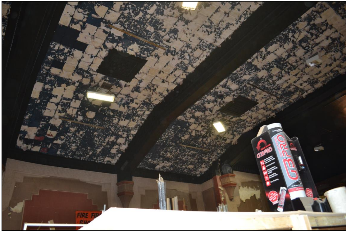
Photograph 35: Detailed view of the ceiling in the auditorium.
