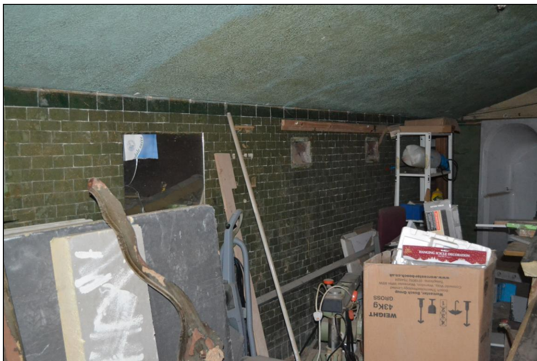
Photograph 17: View of the southern wall of the centre basement room.
