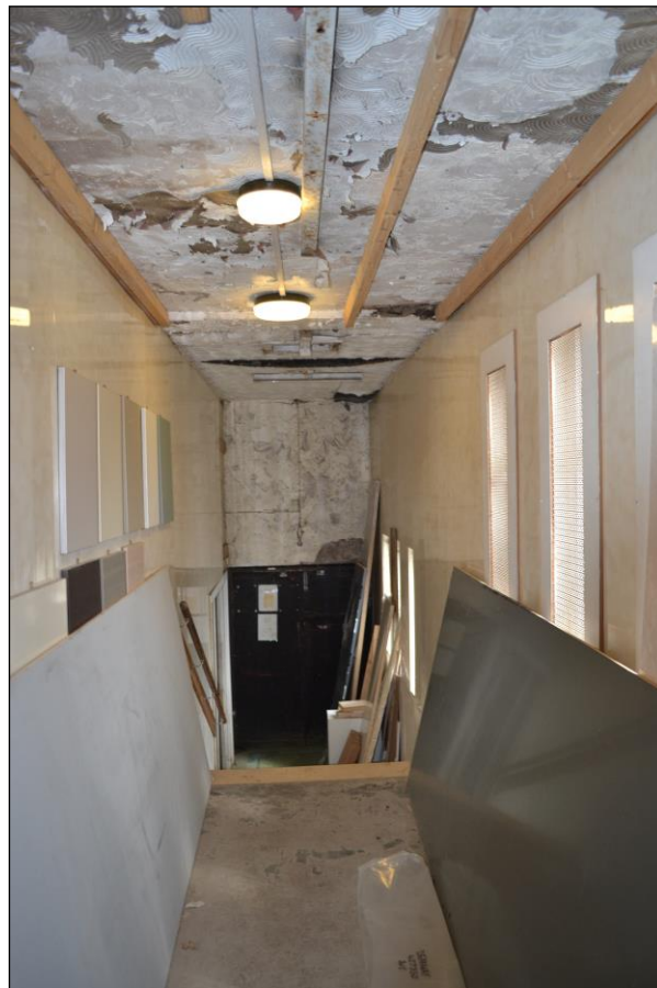
Photograph 22: View north along the hall connecting the showroom to the auditorium.
