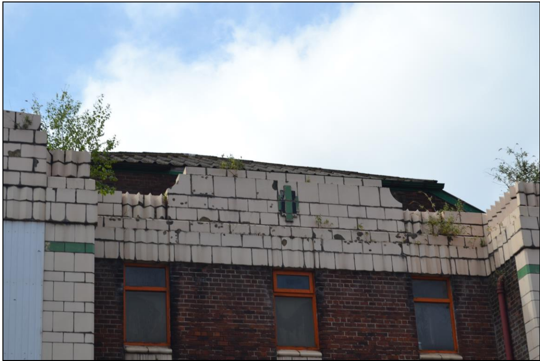
Photograph 3: Detailed view of the roofline detail of the centre section of the northern façade.
