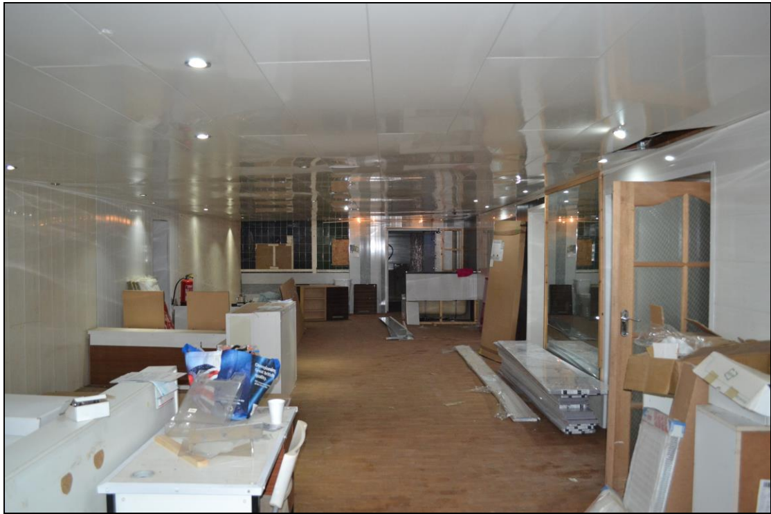
Photograph 21: View east across the main showroom with the new floor and covered walls and ceiling.
