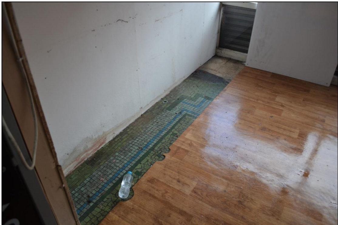
Photograph 20: View of original floor beneath the modern flooring on the ground level.
