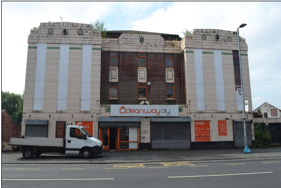
Photograph 1: View south of the northern façade of the former cinema.
