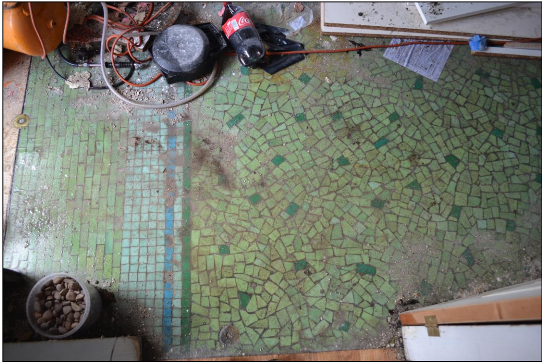
Photograph 19: Likely the original floor in the entry on the ground level.
