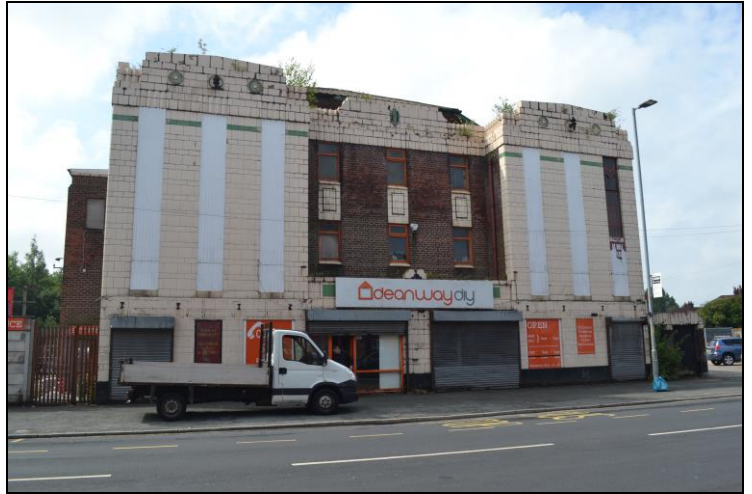
View south-west of the northern façade of Deanway DIY
