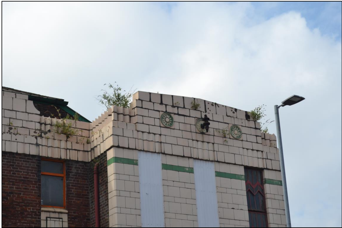
Photograph 7: Detailed view of the roofline detail of the western wing of the northern façade
