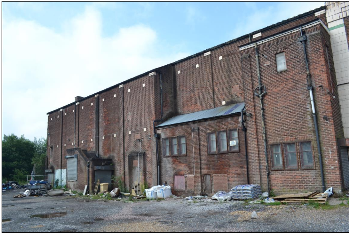
Photograph 9: View south-west along the eastern façade.
