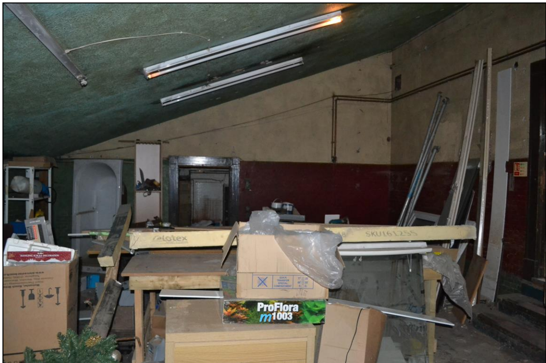
Photograph 16: View west across the centre basement room towards the inaccessible western room.
