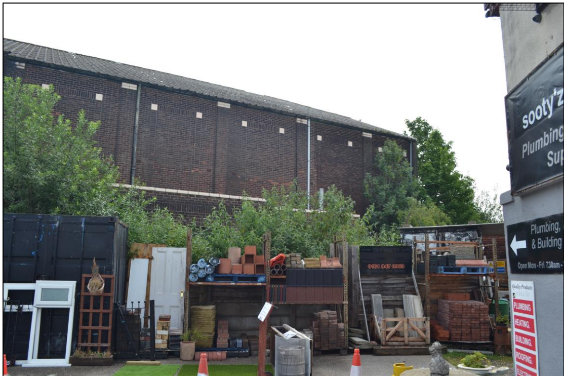
Photograph 14: View south-east of the southern part of the western elevation.
