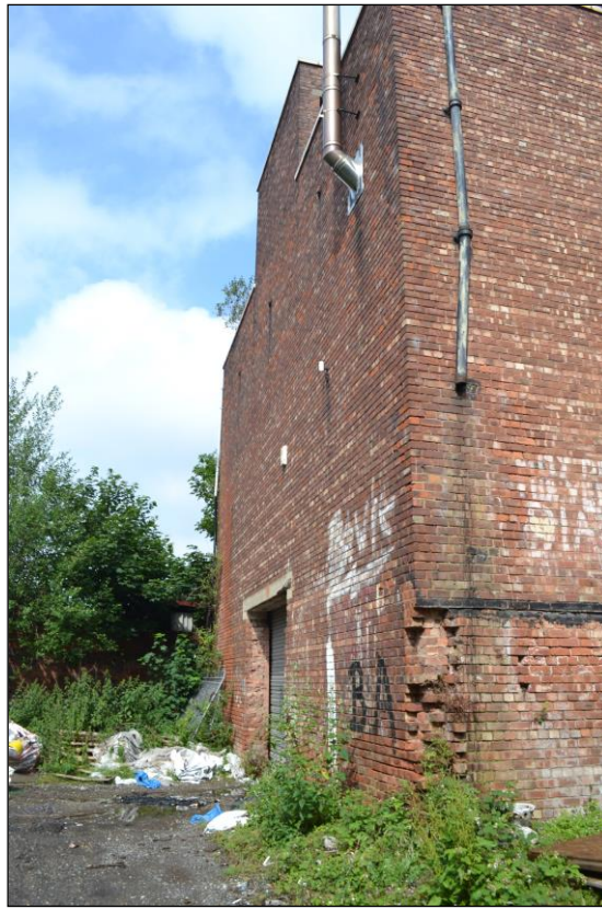
Photograph 11: View west of the southern elevation.
