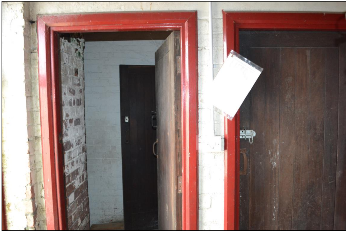
Photograph 27: View of a second office and doorway leading to the stairs in the eastern wing.
