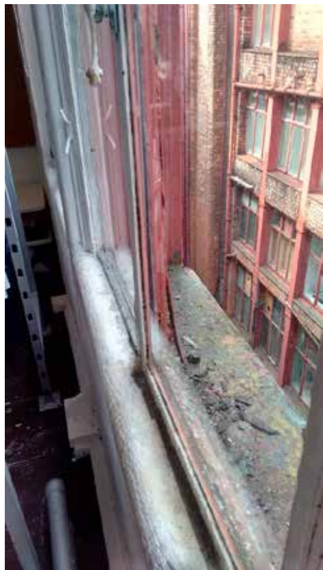
EXISTING STEEL WINDOWS 49-51 DALE STREET
