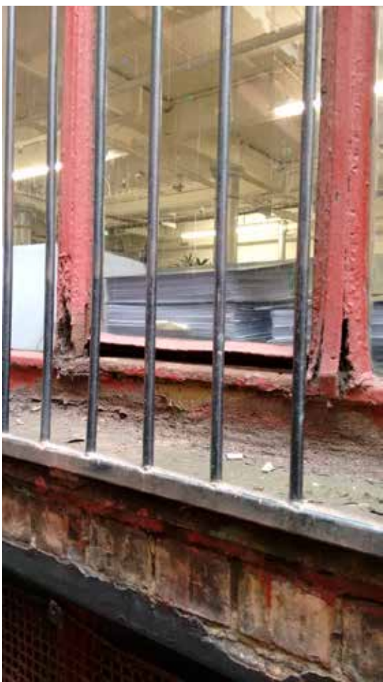
EXISTING STEEL WINDOWS 49-51 DALE STREET
