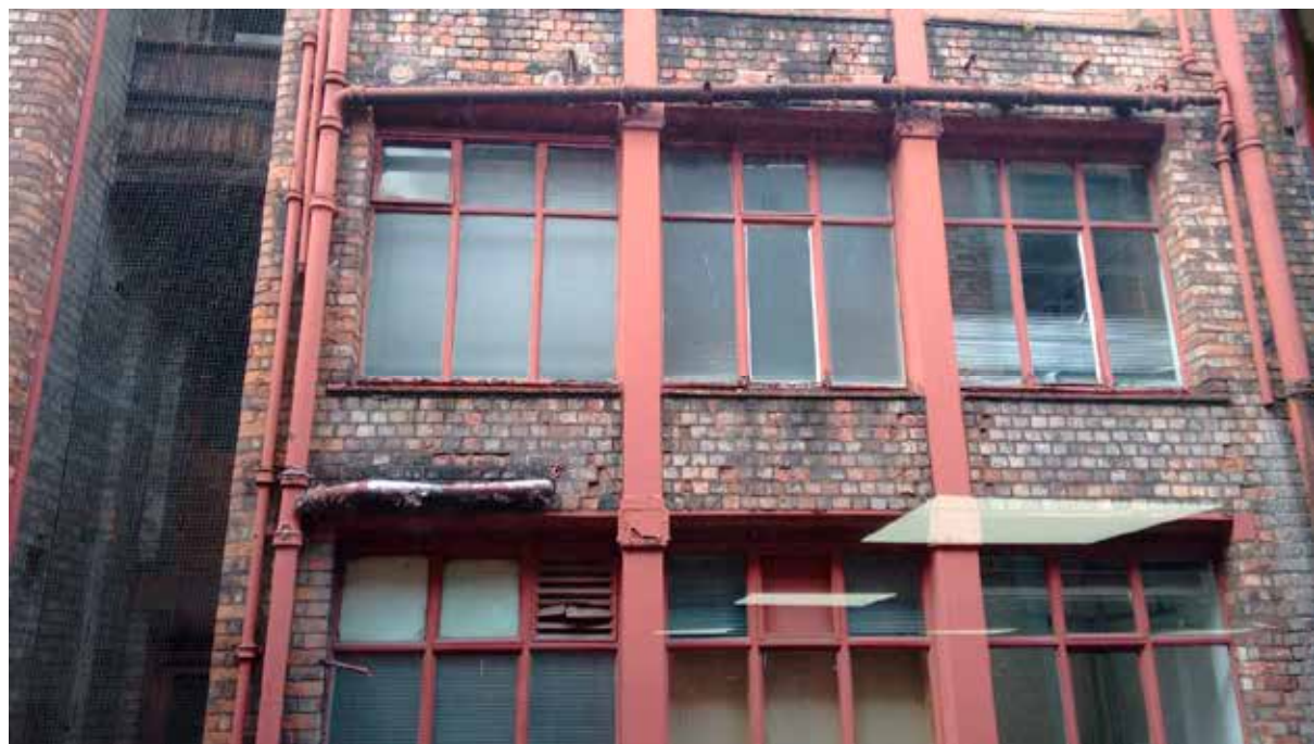
EXISTING STEEL WINDOWS 49-51 DALE STREET
