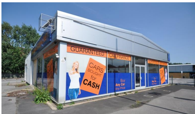
The front elevation facing Bury New Road
