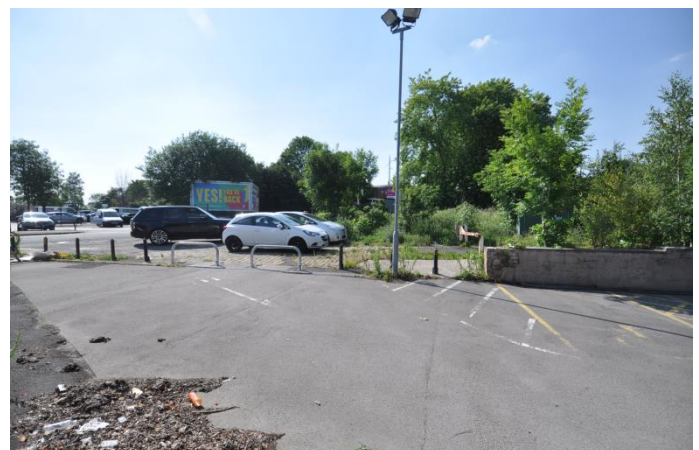
The south elevation that overlooks Pure Gym's car park
