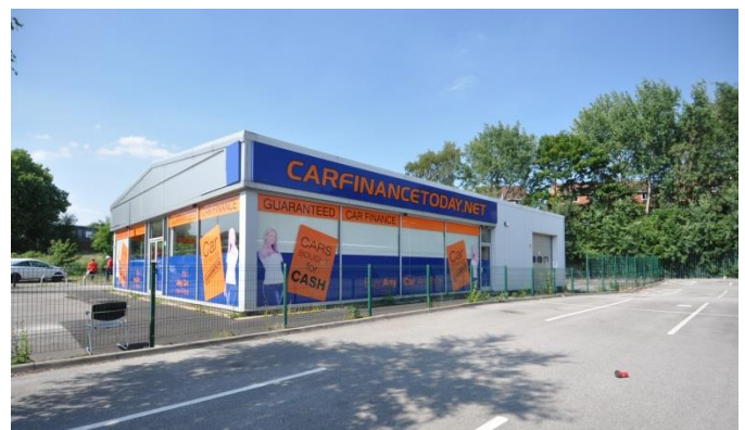
The south elevation that overlooks Pure Gym's car park
