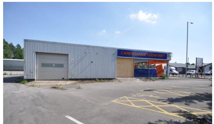
The north elevation facing the site's vehicular entrance
