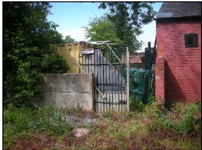
Demolished outbuilding location
