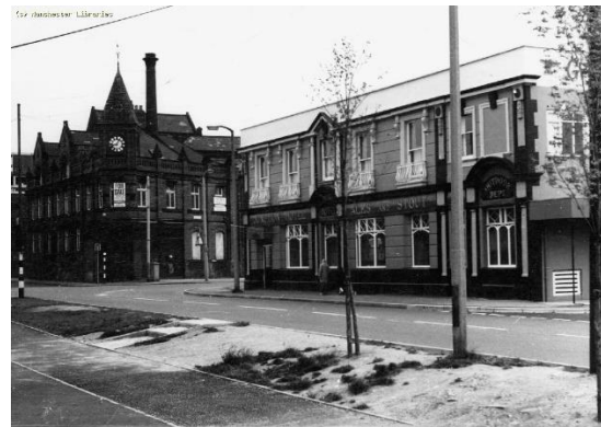
Image 14: 1971 photo of former hotel from Rolls Crescent.
