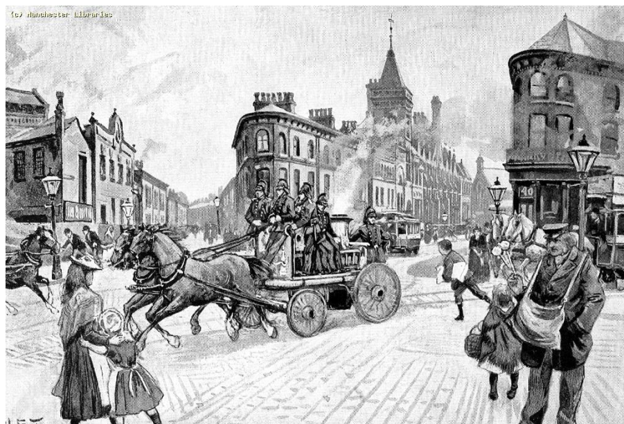
Image 17: 1890 Sketch of Hulme Junction, HT Tidmarsh – The Junction Hotel is just out of view to the right, the sketch being undertaken from directly outside it. From right to left, no.40 Upper Jackson Street, South Hulme Senior Girls School (with tower), and the Naval Brewery are all visible.
