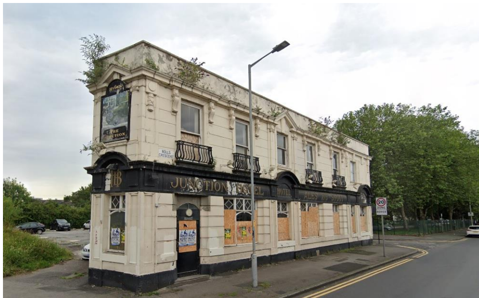
Image 3: Former Junction Hotel – north elevation
