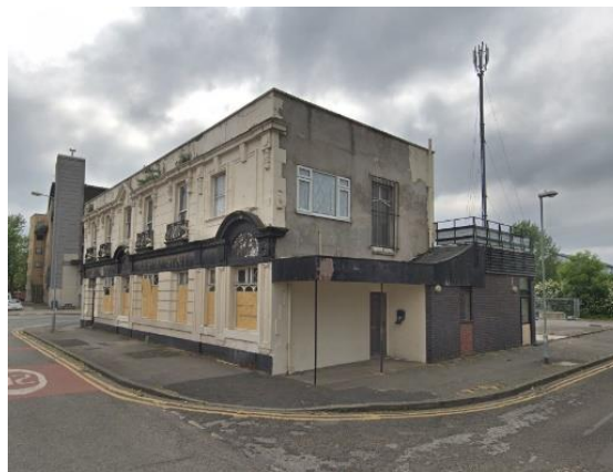
Image 5: West Elevation and single storey extension
