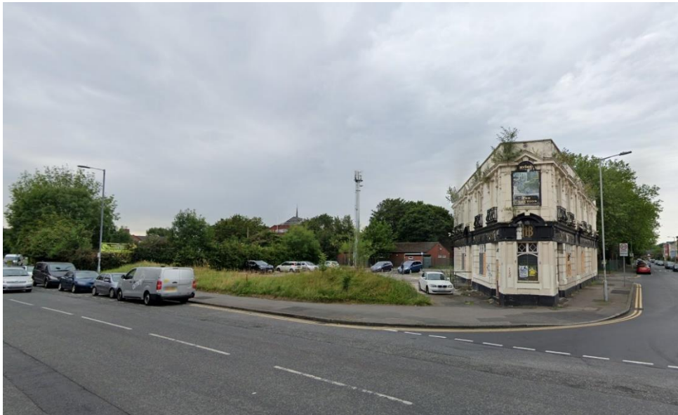
Image 18: East elevation and wider site – present day
