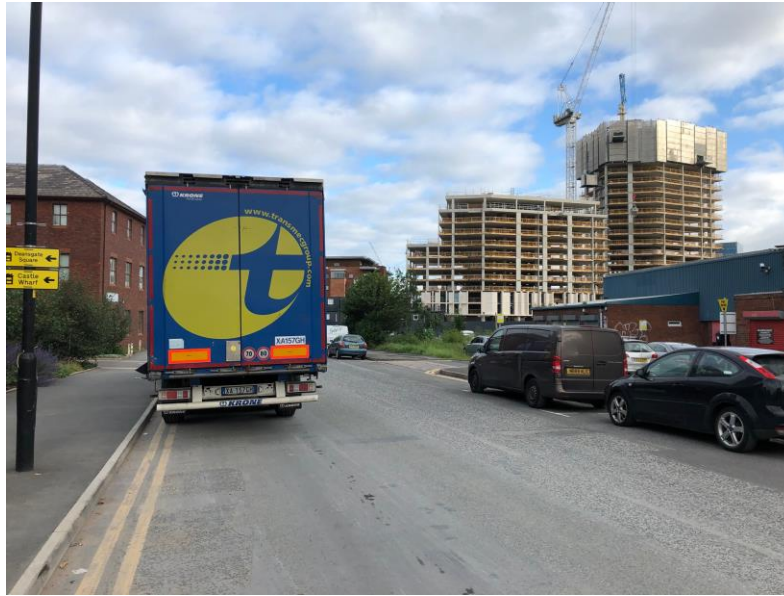
View looking north showing Gaddum House, Chester Rd and Castle Wharf to north east
