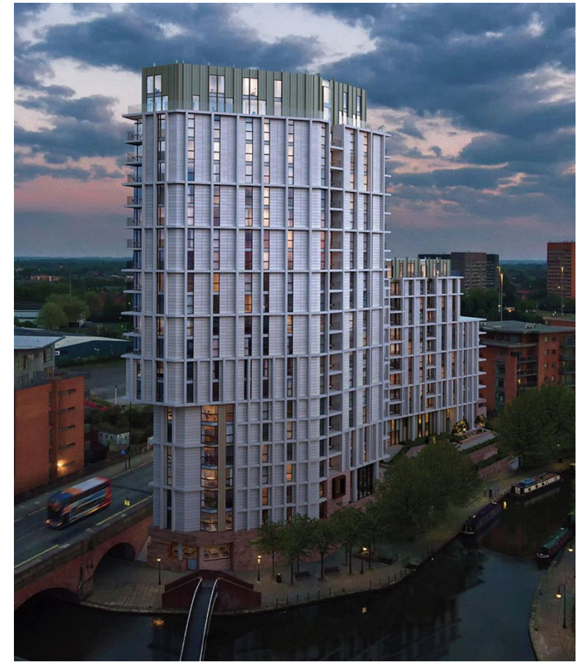
Castle Wharf Development
