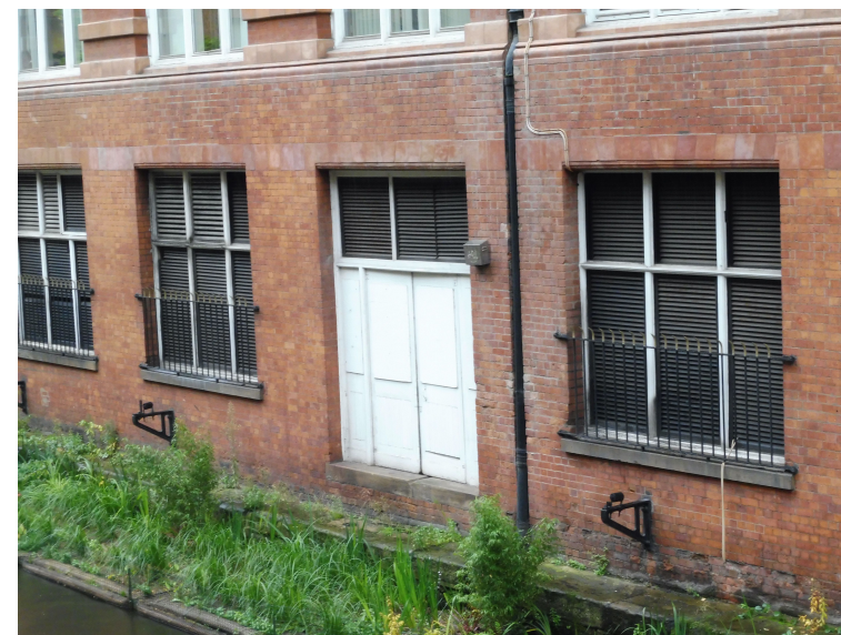
Photo of existing louvred window with ornate metal security bars on the canal side elevation
