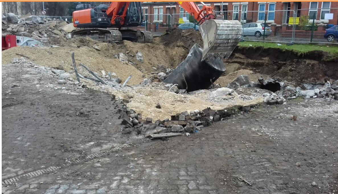
PLATE 5 – REMOVAL OF TANKS
