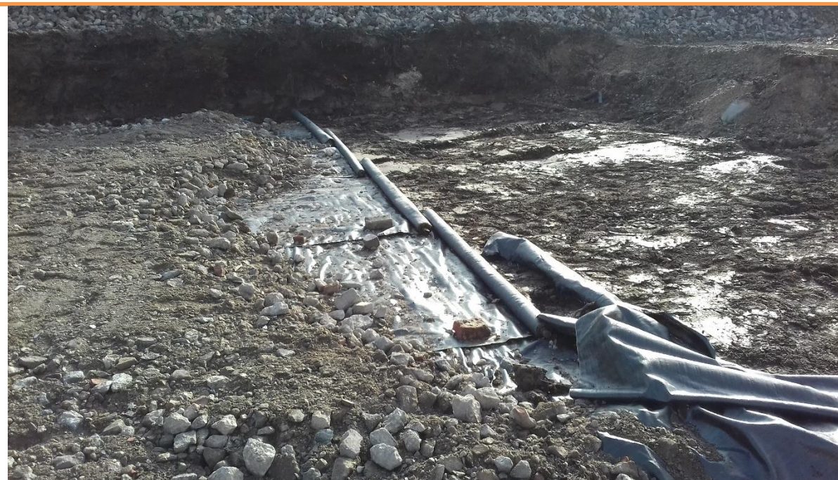
PLATE 29 – PLACEMENT OF CRUSH MATERIAL WITHIN PILING MAT
