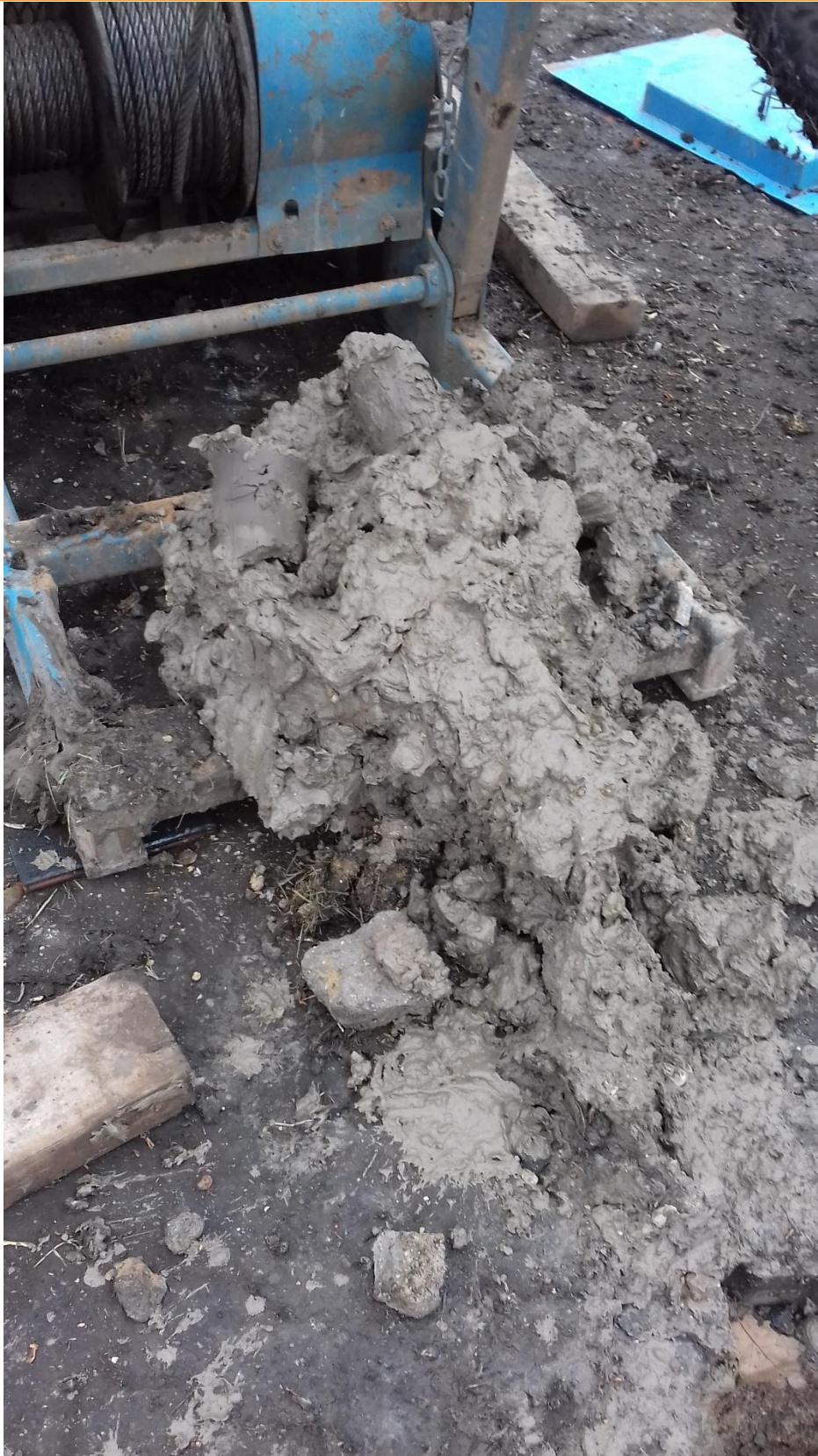
PLATE 3 – ARISING FROM REDRILLED BOREHOLE
