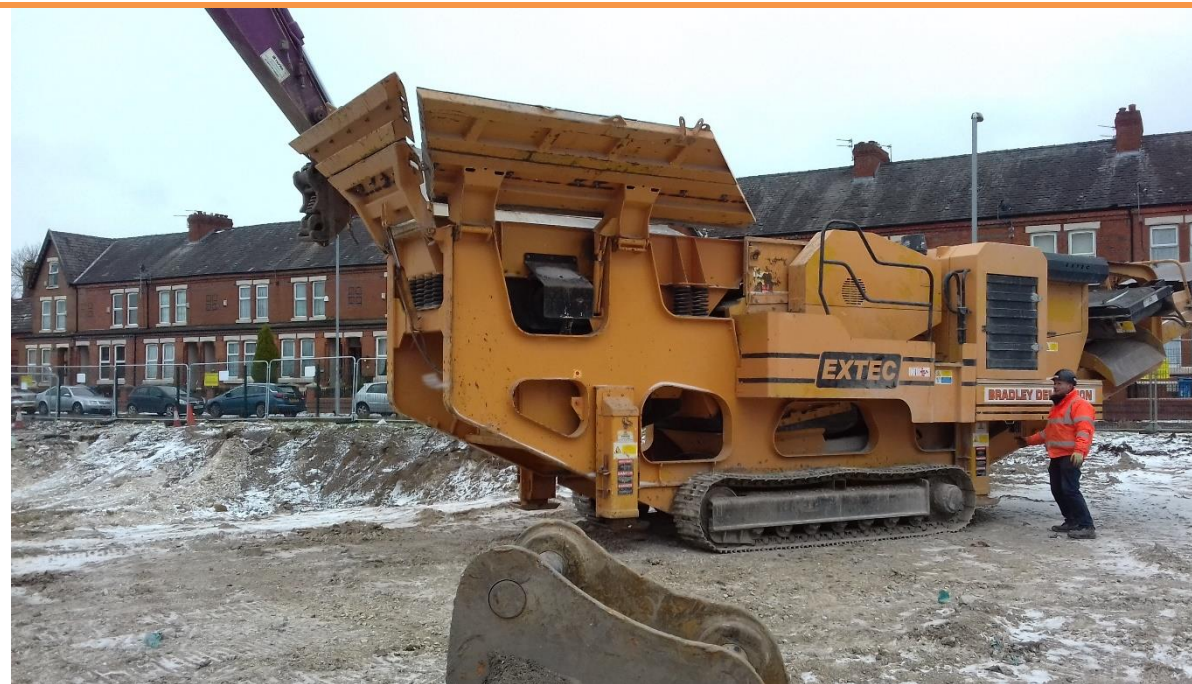
PLATE 28 – CRUSHER USED TO GRADE OVERSIZE MATERIALS
