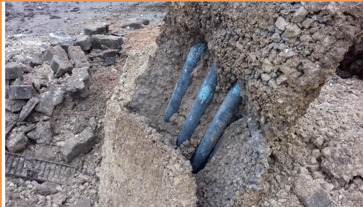
PLATE 15 – FUEL PIPES WERE ENCASED IN CEMENT
