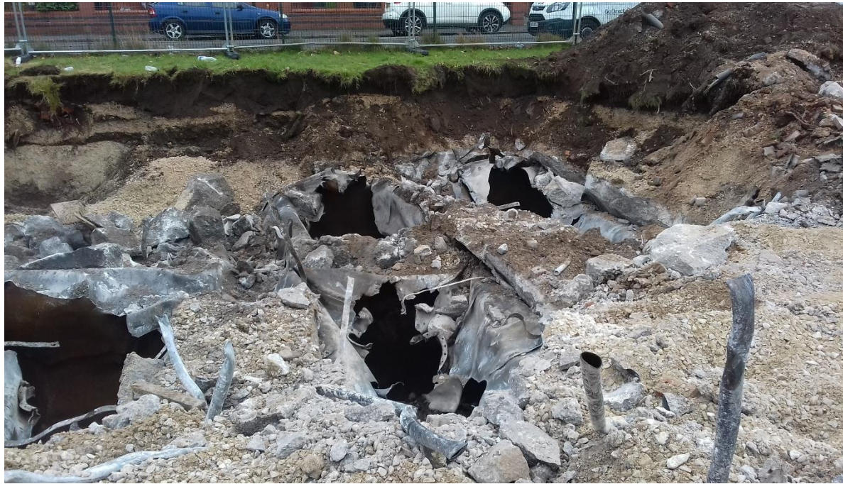
PLATE 4 – DECOMMISSIONED WITHIN CONCRETE CASING
