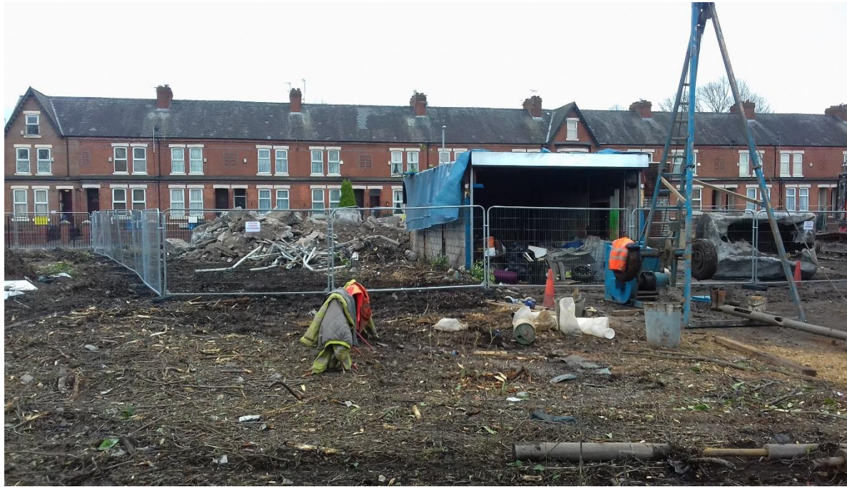
PLATE 1 – REDRILLING AND BACKFILLING OF FORMER MONITORING WELLS
