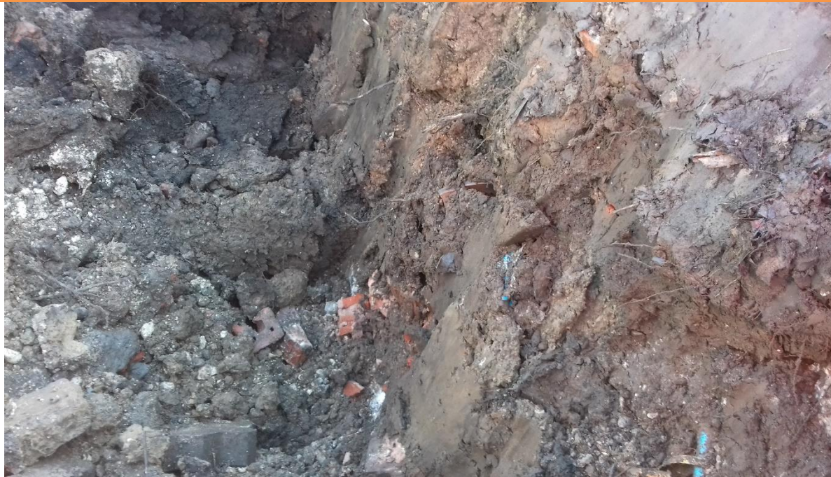
PLATE 24 – HS1 FOLLOWING EXCAVATION
