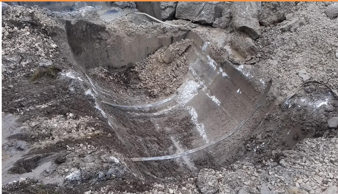
PLATE 11 – BASE OF TANK 1 CASING FOLLOWING REMOVAL OF FUEL SOAKED MATERIAL
