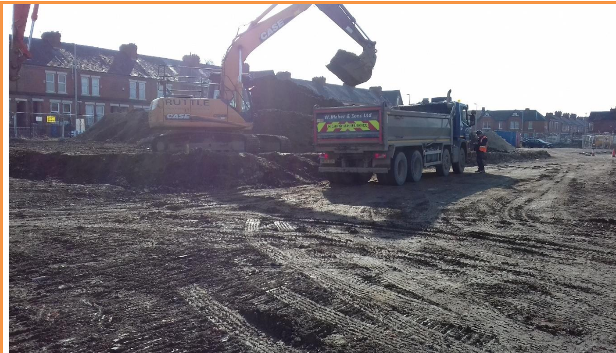
PLATE 32 – EXPORTATION OF TOPSOIL MATERIAL
