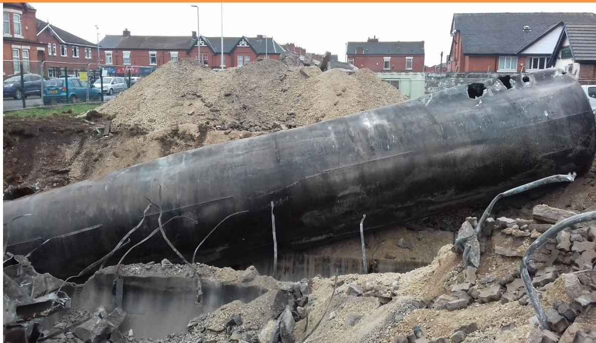
PLATE 7 – REMOVAL OF TANK 5
