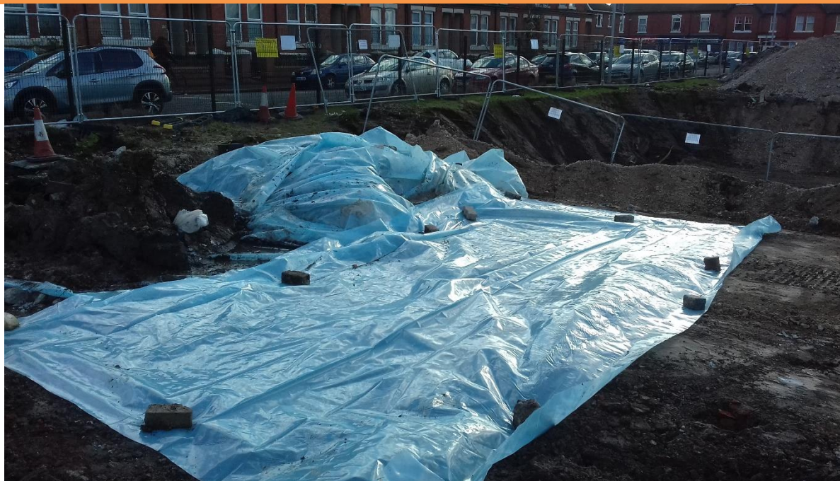
PLATE 25 – PLACEMENT OF HS1 ARISINGS ON IMPERMEABLE MEMBRANE
