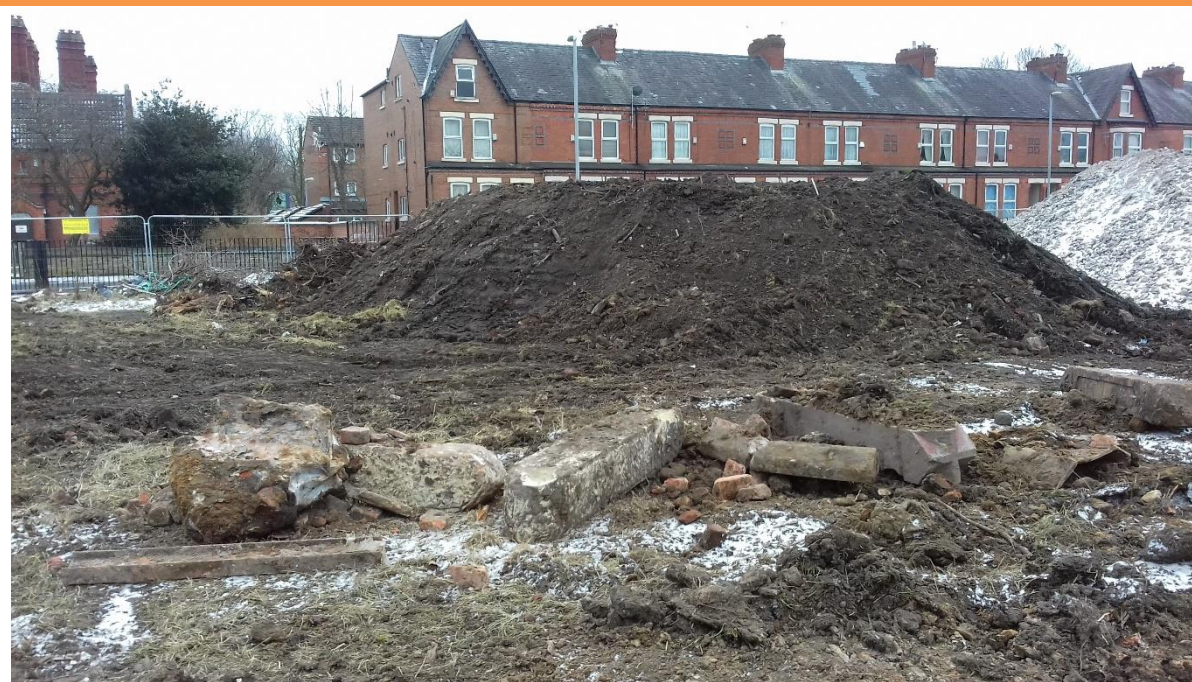
PLATE 26 – STOCKPILE OF STRIPPED TOPSOIL PRIOR TO REMOVAL FROM SITE
