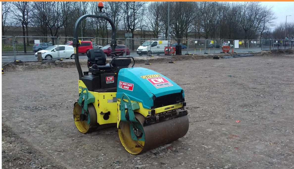
PLATE 30 – ROLLER USED TO ACHIEVE REQUIRED CBR FOR PILING MAT
