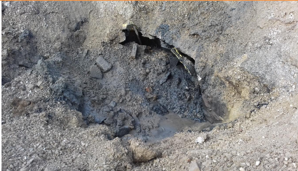
PLATE 18 – INTERCEPTOR DURING EXCAVATION
