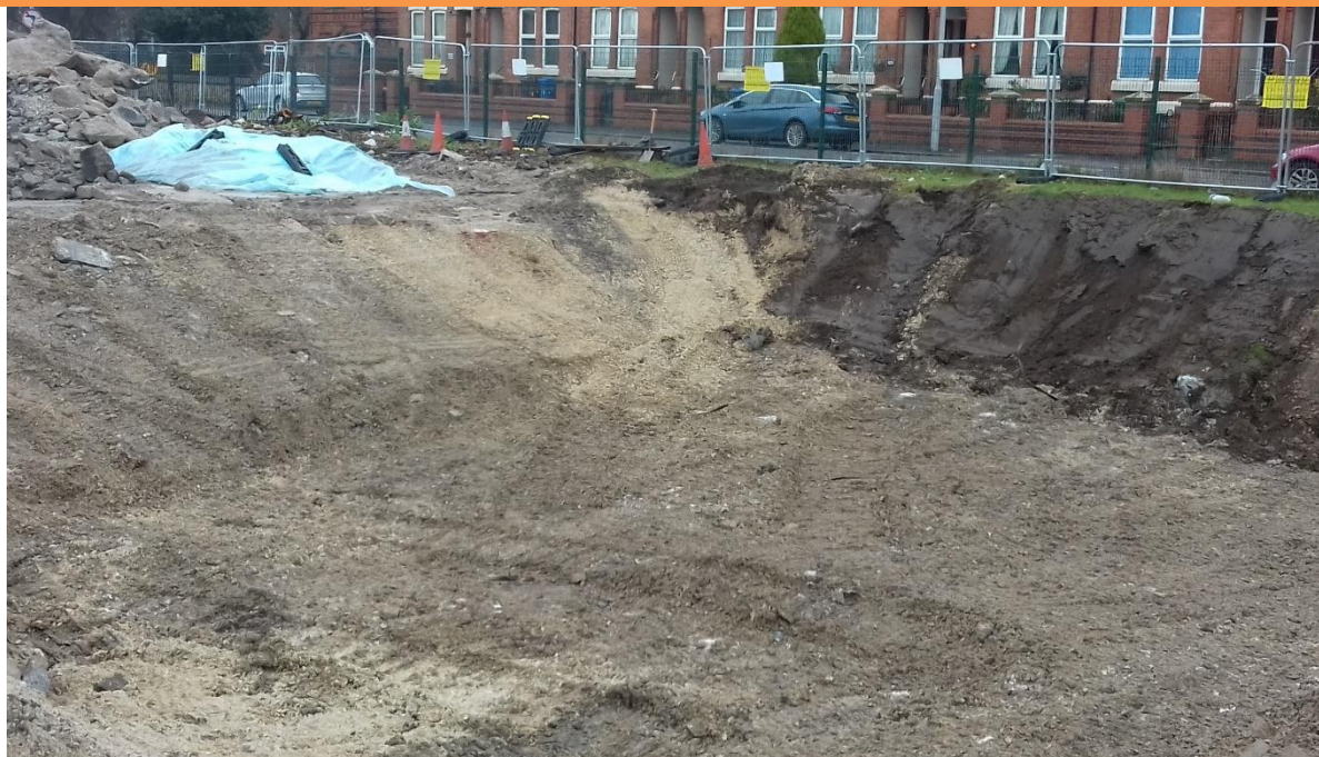
PLATE 13 – AREA OF TANKS FOLLOWING BACK FILL OF CONCRETE CASING WITH GRANULAR MATERIAL
