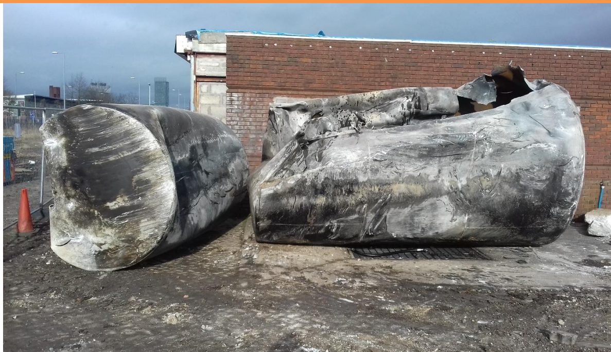
PLATE 6 – TANKS FOLLOWING REMOVAL
