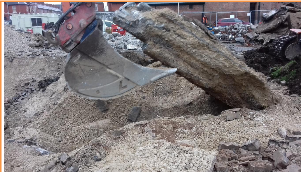
PLATE 14 – REMOVAL OF PIPES BETWEEN TANKS AND FILLING BAYS
