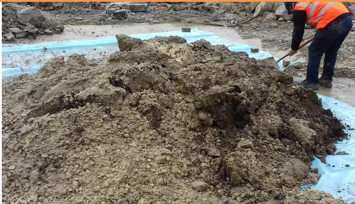
PLATE 12 –PLACEMENT OF MATERIAL USED TO SOAK UP LIQUID IN TANK 1 ON IMPERMEABLE MEMBRANE
