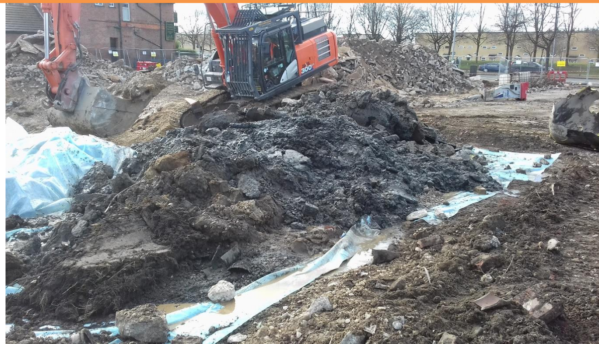
PLATE 22 – PLACEMENT OF EXCAVATED MATERIAL ON IMPERMEABLE MEMBRANE
