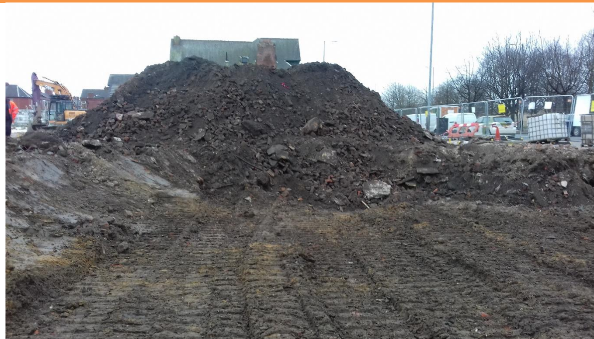
PLATE 27 – REDUCED LEVEL DIG AND STOCKPILE OF SITE WON BULK FILL
