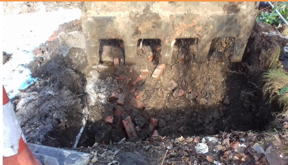
PLATE 23 – EXCAVATION OF HS1
