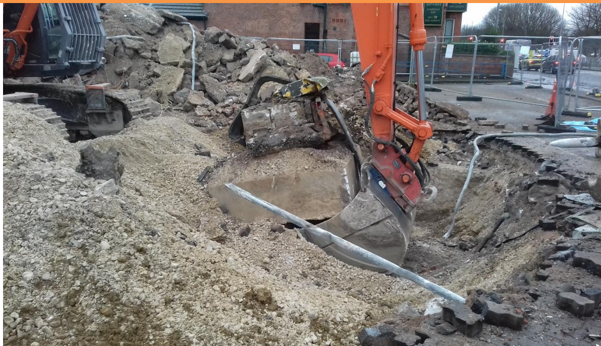
PLATE 16 – REMOVAL OF FILLING BAY INCLUDING CONCRETE FOOTING
