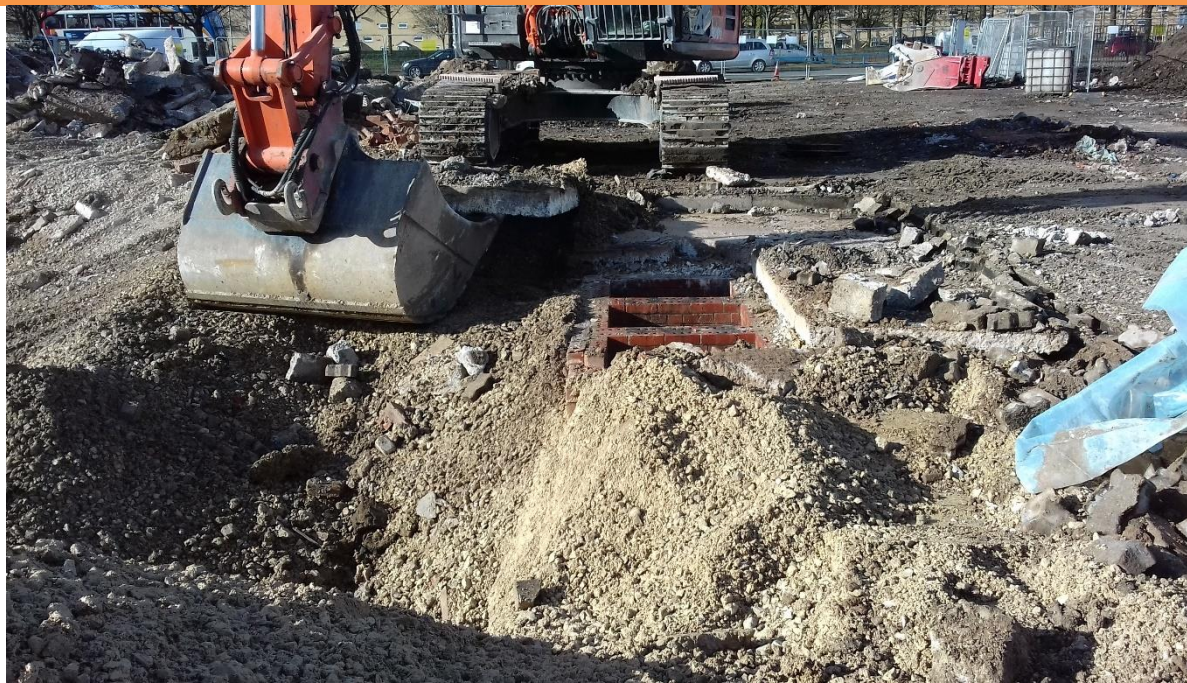
PLATE 17 – EXCAVATION AROUND INTERCEPTOR
