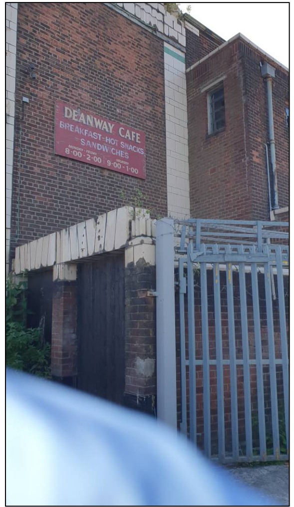
Plate 2 West face of the building
