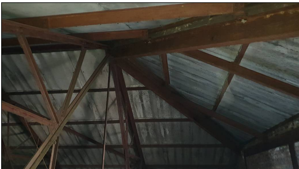
Plate 8 Beams within the roof structure
