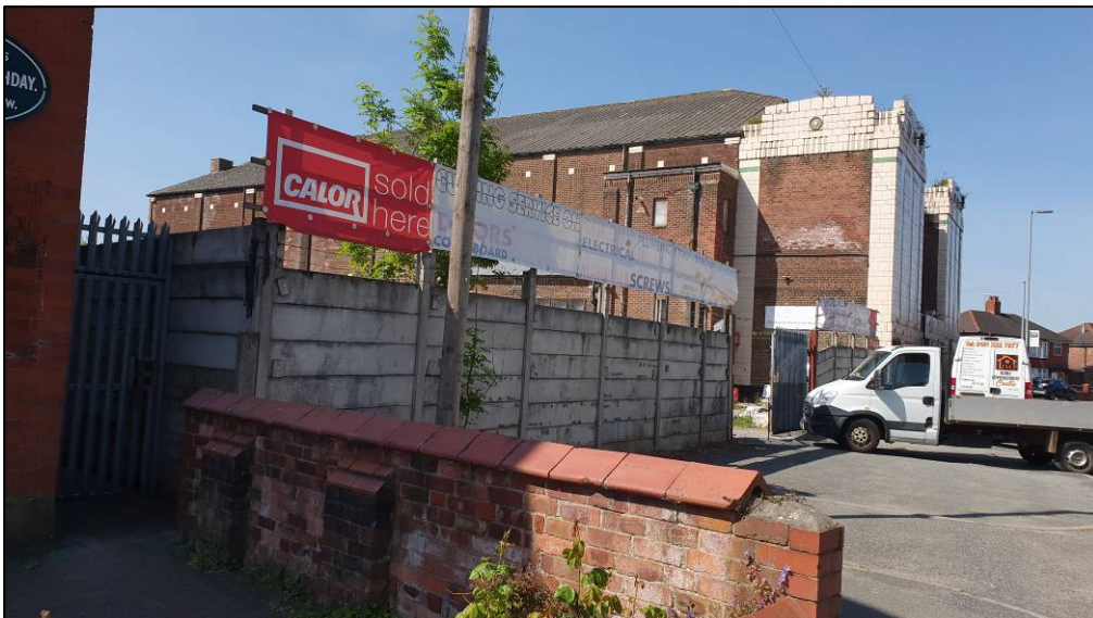
Plate 3 East face of the building from a distance
