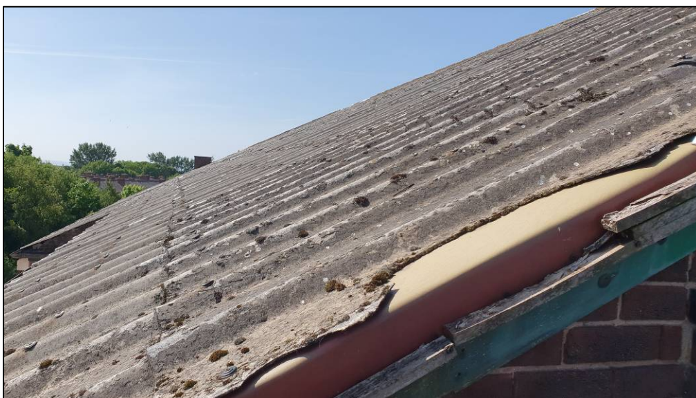
Plate 5 Asbestos pitched roof
