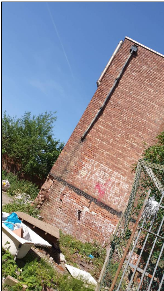
Plate 4 Southern east face of the building
