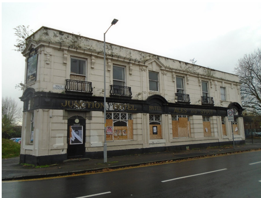
Photo 1: Junction Hotel Building
