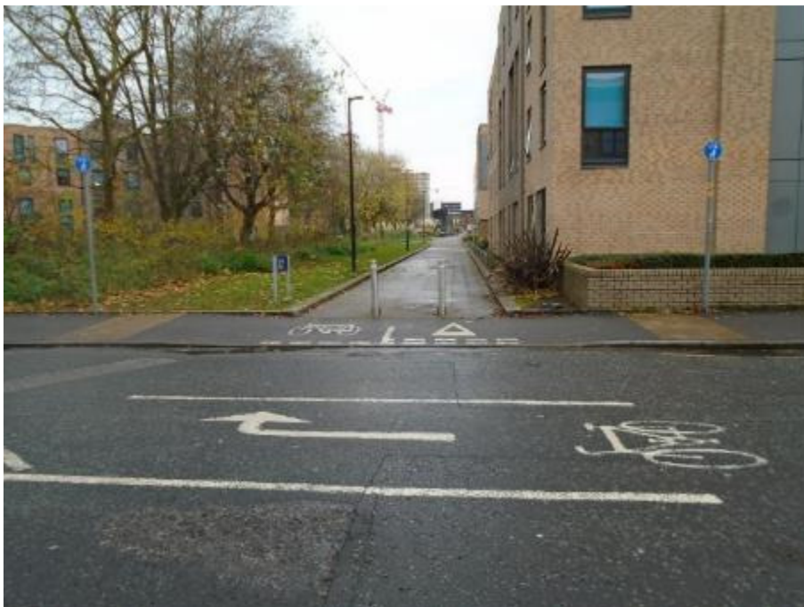
Photo 11: Off-road Cycle Connection from Old Birley Street
