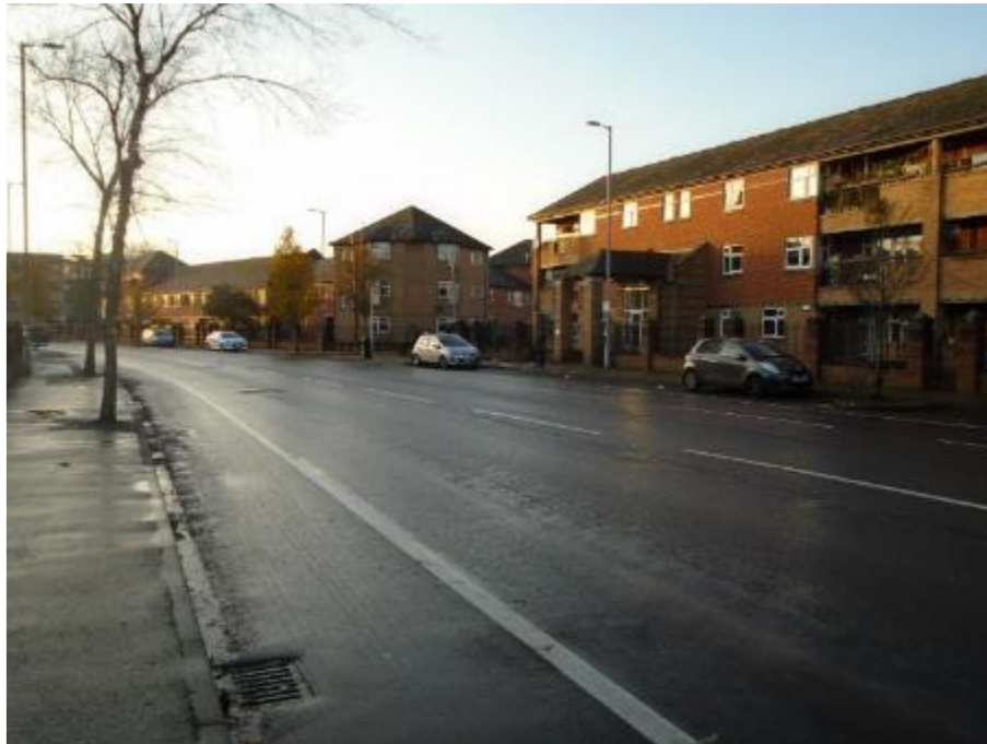
Photo 12: Cycle Lanes on Greenheys Lane West
