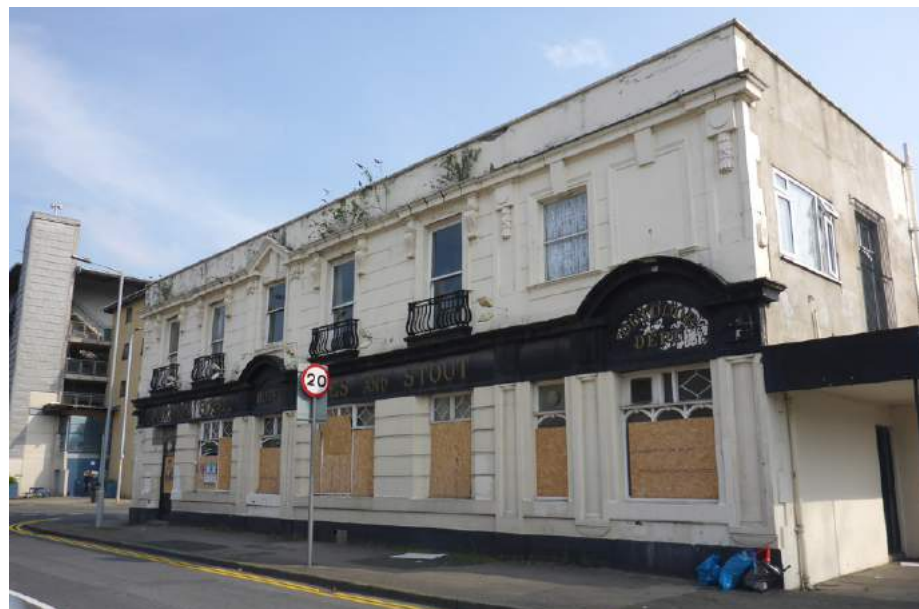
Junction Hotel old Warde Street North Facade
