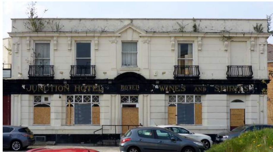
Junction Hotel old Preston Street South Facade
