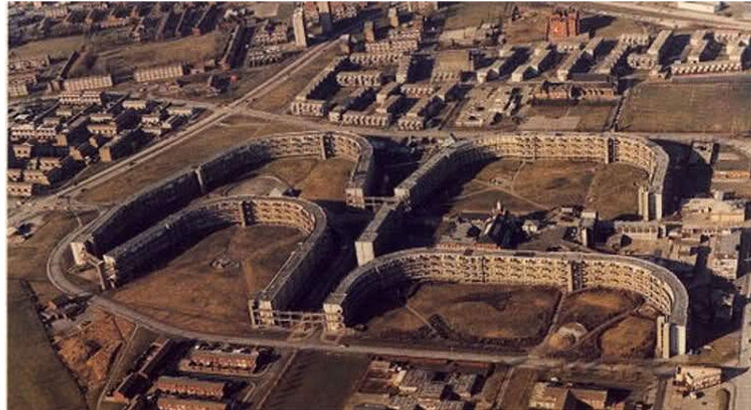
Hulme Crescents before demolition - the Junction Hotel is recognisable in the bottom right of the image.
