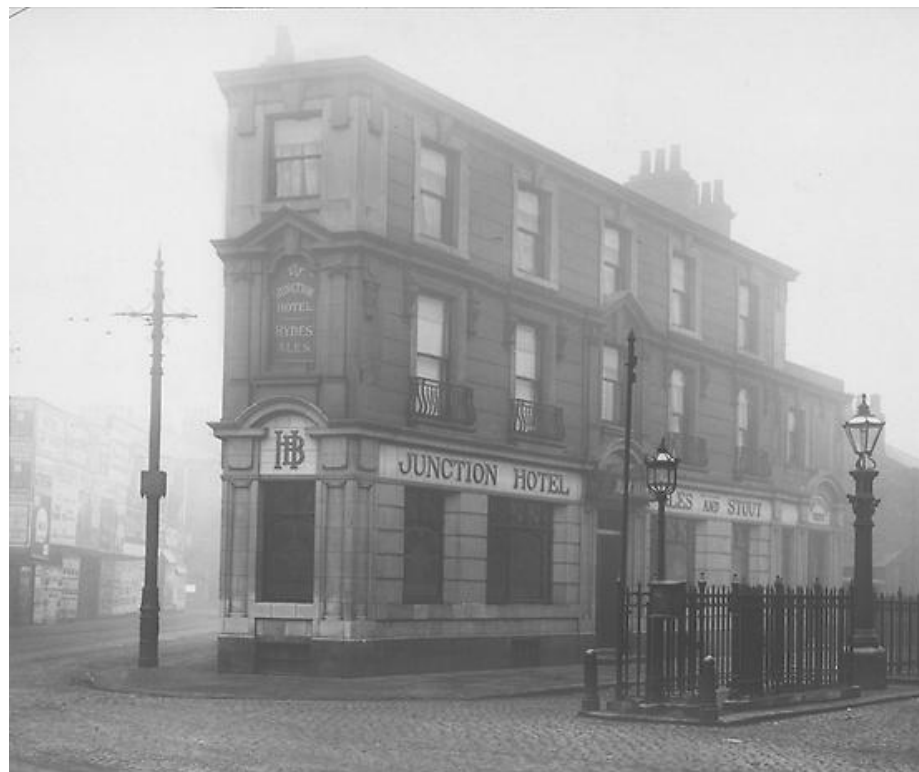
Junction hotel prior to removal of third storey
