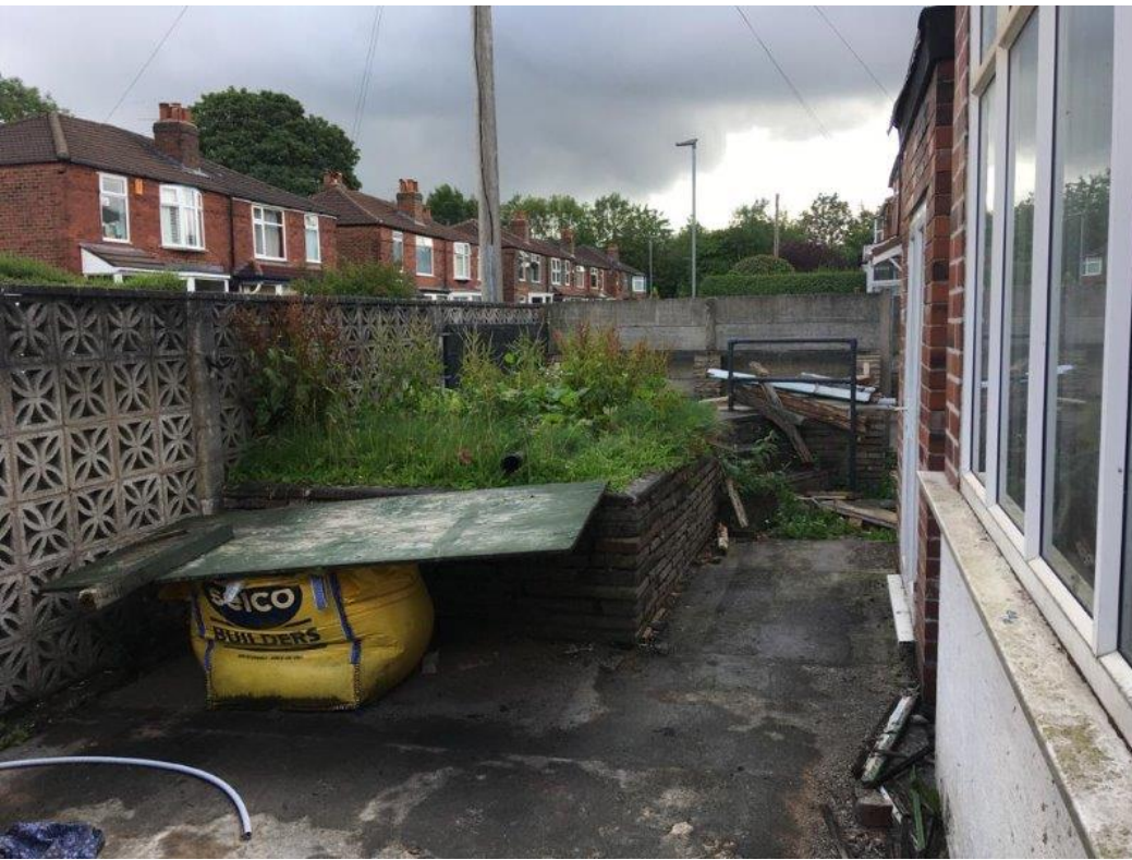
IMAGE 8 INTERNAL BOUNDARY VIEWED FROM RAISED DECK
