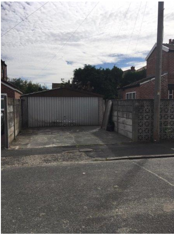
IMAGE 4 EXTERNAL BOUNDARY VIEWED FROM EAST END OF CRAIGWEIL ROAD
