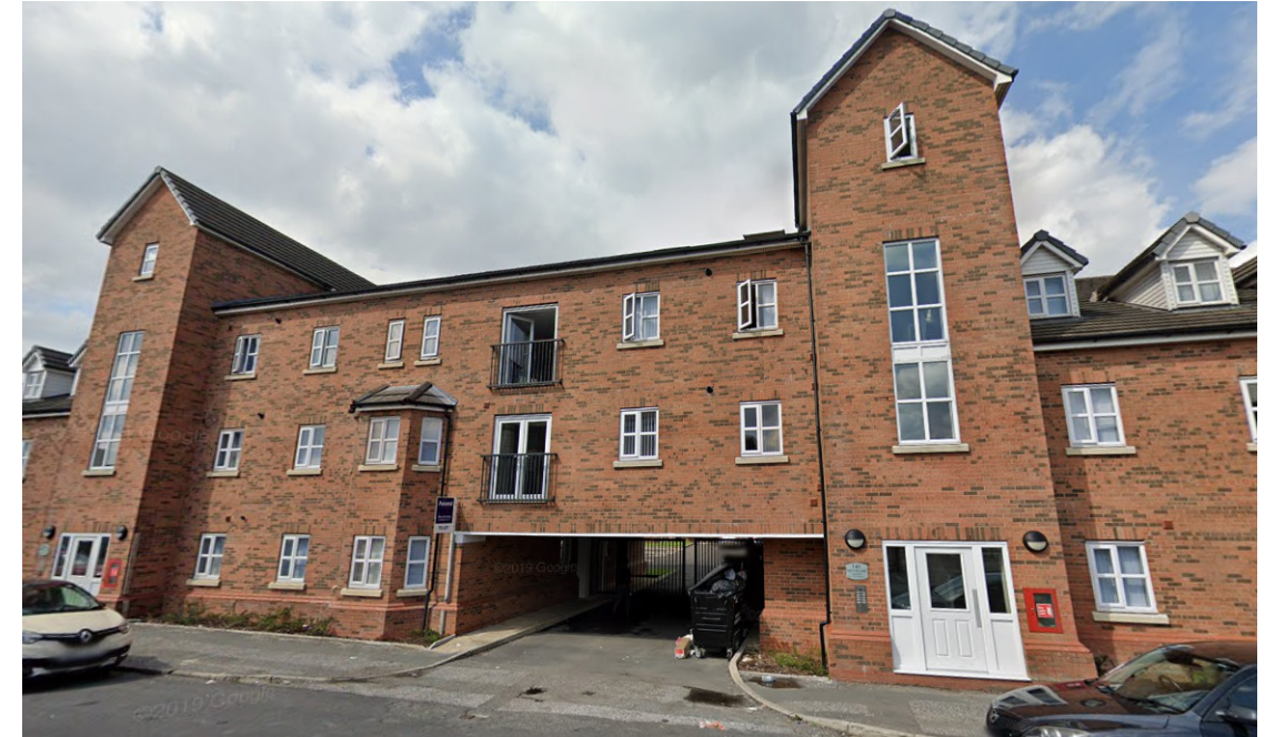
2. Undercroft providing access into the development.
