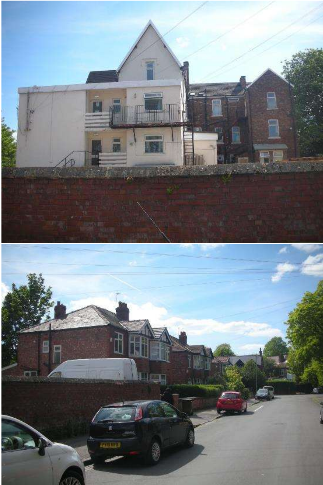
Figure 22: View to South of parking lot and commercial building / Dwellings to the West (down May Road)
