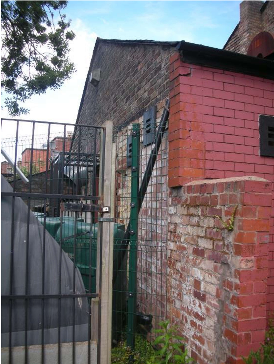
Figure 11: Demolished outbuilding (white outline on wall)
