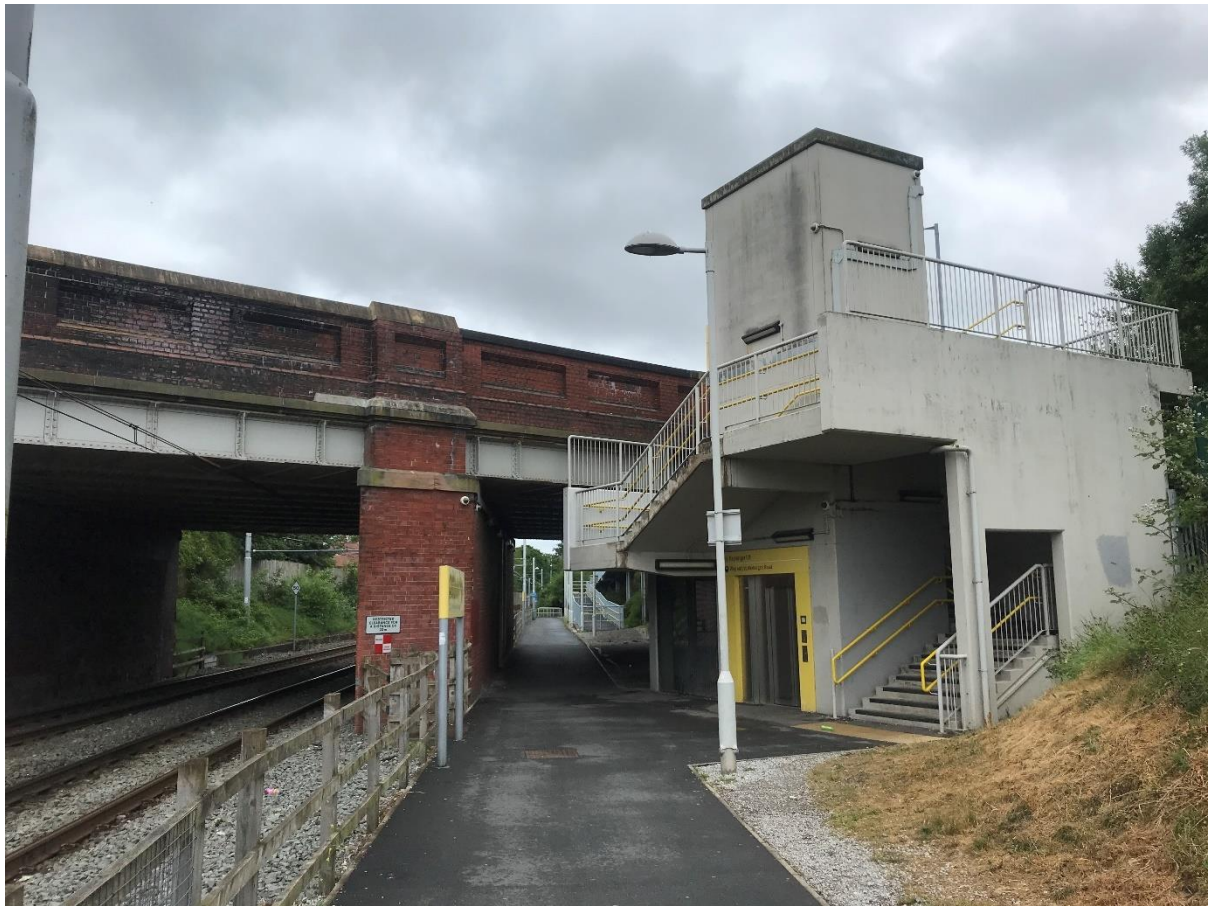
Figure 2: Picture Showing Monitoring Position 2
